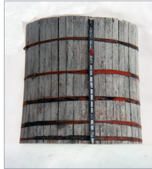
10. The water-level gauge.
