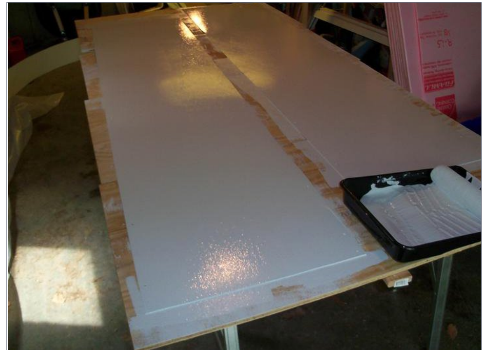
6. Bonding primer appears shiny when wet but dries flat, ideal for applying paint.
