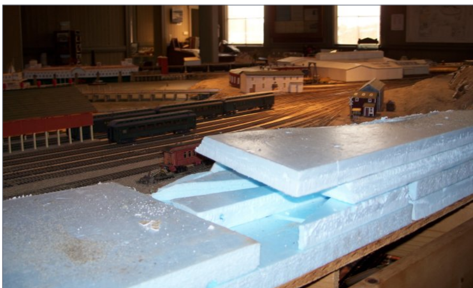
12. Here blue foam is being glued and carved into a hillside land form at the back of the layout.
