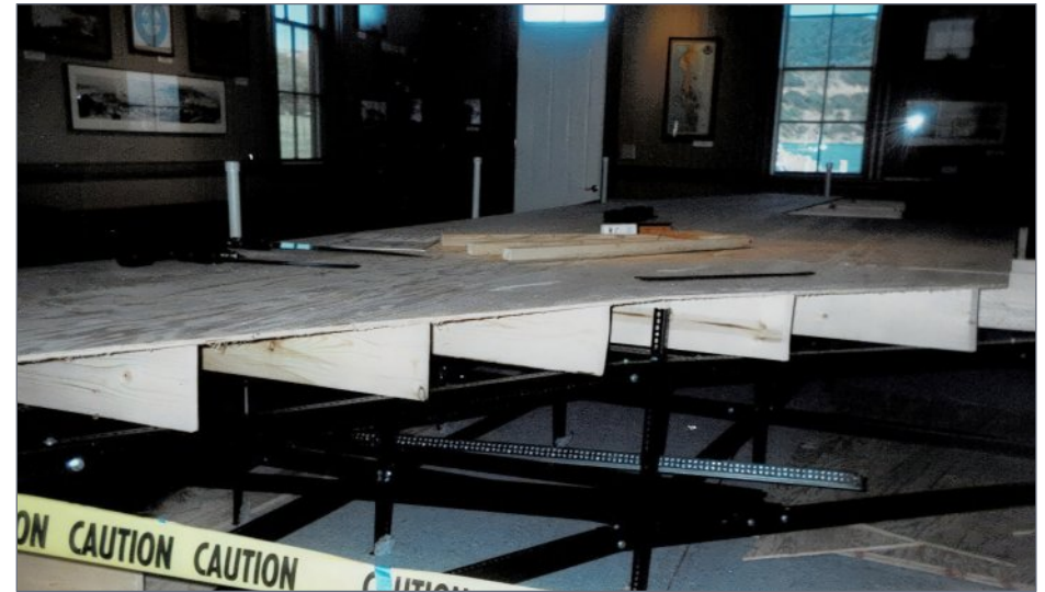
13. Benchwork supported by black angle iron creates a solid foundation for the 1x8 joists and half-inch plywood tabletop.
