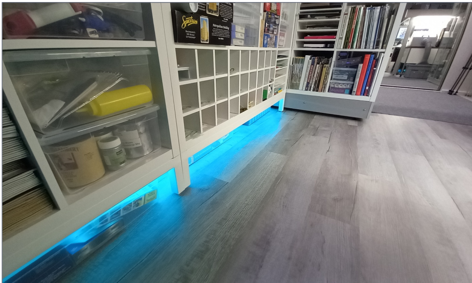
13. LED light strips are an inexpensive and creative way to add color accents. Magnets hold this strip to the metal shelf legs.
