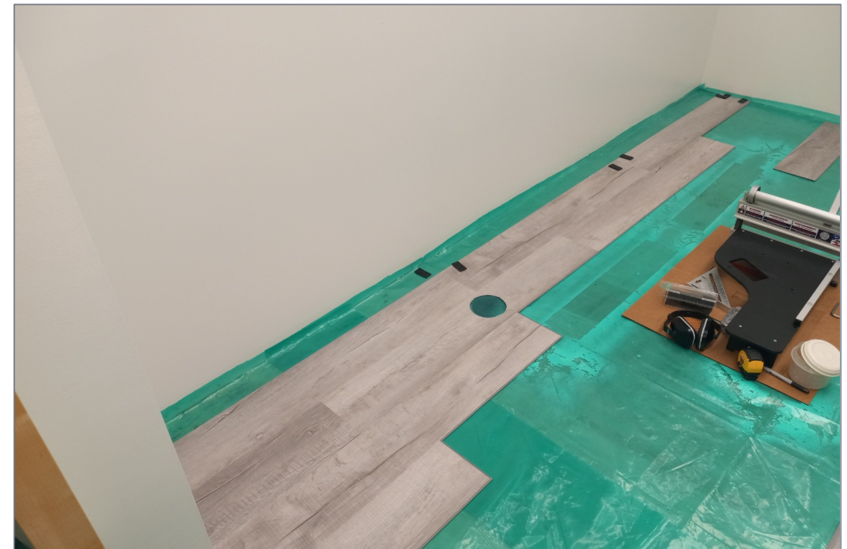
5. Vinyl plank flooring is easy to cut and it's waterproof.
