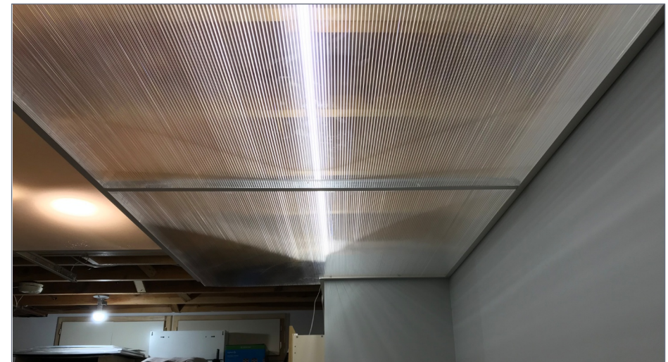
3. Polycarbonate panels are lightweight but rigid, easy to cut, and diffuse light evenly.
