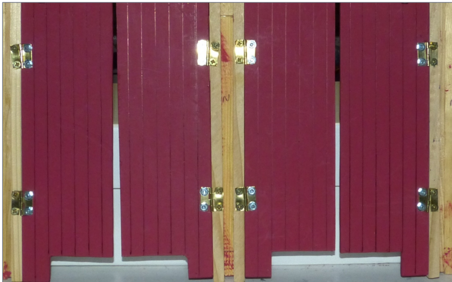
4. Doors installed on front structure as viewed from inside the building.
