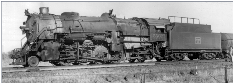
1. Burlington 5507, photographed near Faulkner, TX in November 1956, was a USRA Heavy Mikado modified with a Worthington feedwater heater on the right side of the boiler, just in front of the firebox. The original coal tender was converted to oil by 1926. Harold K. Vollrath collection
