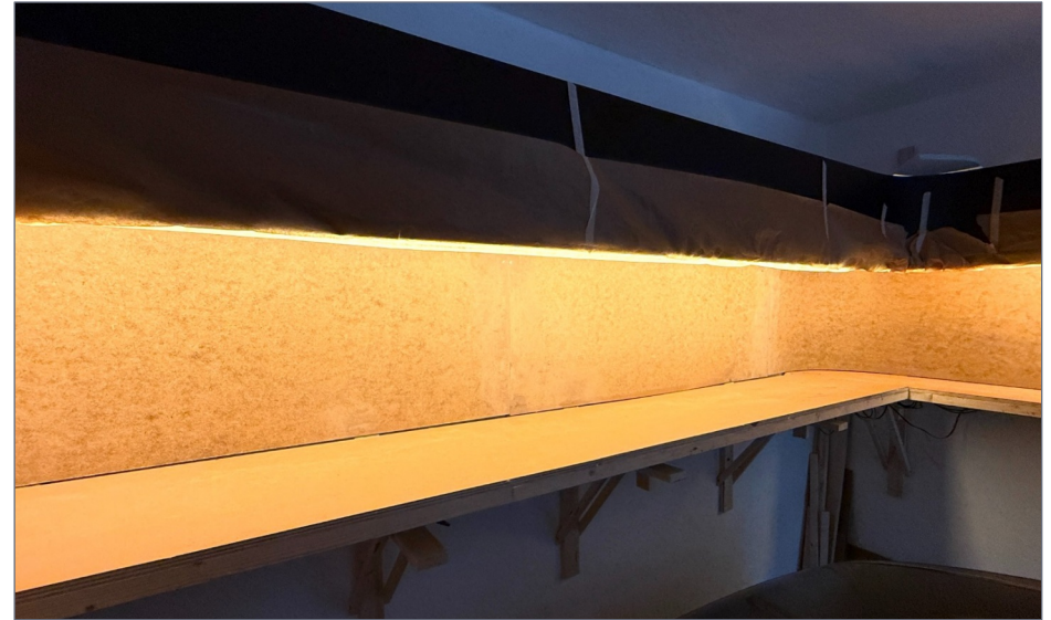
7. I bit the bullet and ripped out the old backdrop and installed a new one that was level with the benchwork tabletop.
