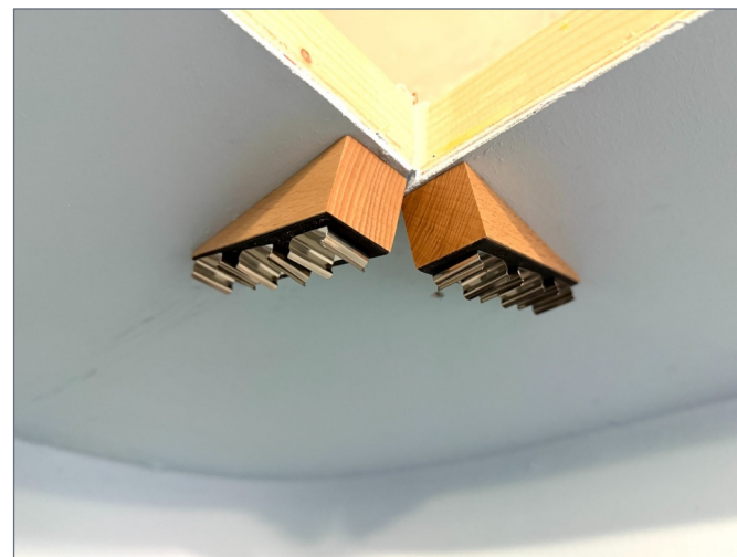
9. Wooden door-stop wedges served as mounting strips for the lighting channel clips to set the lighting source at an angle. See [10].
