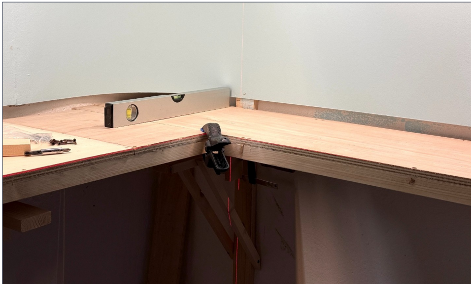
6. Even with the layout shelf perfectly level, I had not accounted for the garage walls not being perfectly square. I found this caused an ugly gap between the backdrop and the bench.
