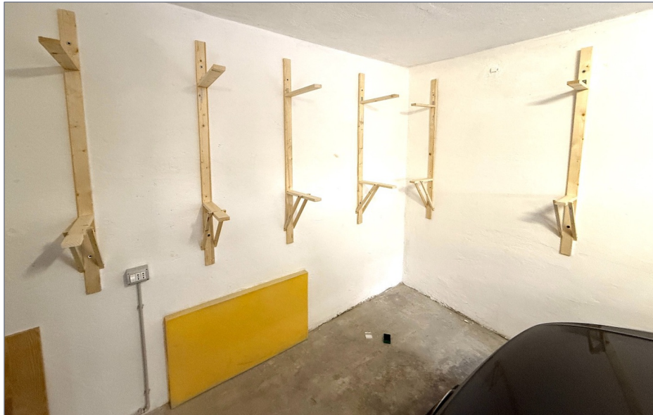
3. I started with wood supporting brackets on the wall.
