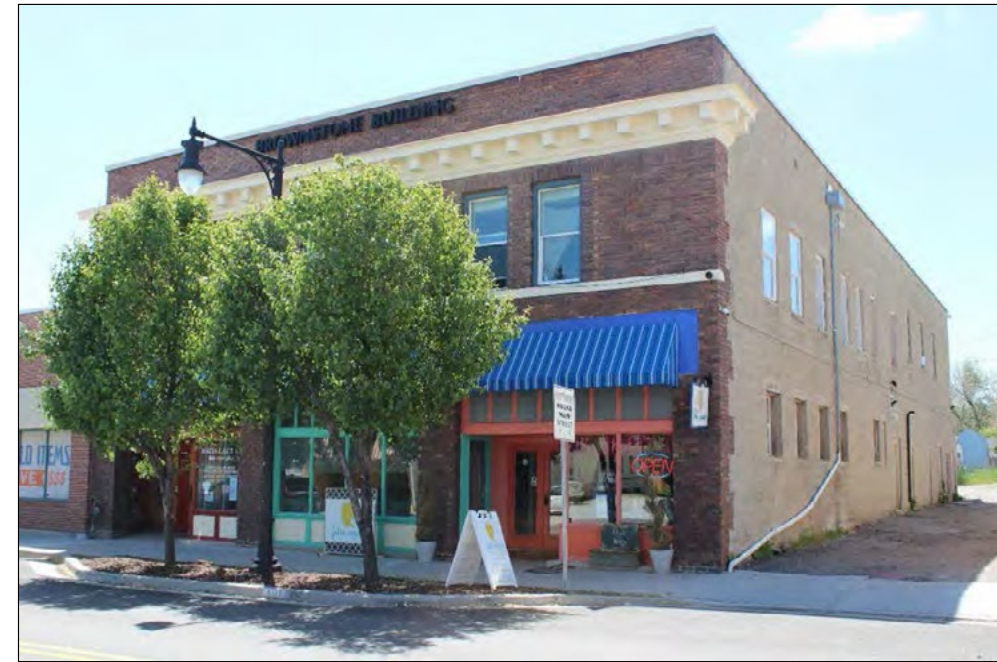
38 of 56 9113 West Magna Main Street, contributing, north and west elevations, facing south. Photographer: K. Hovanes Date photographed: 5/12/17
