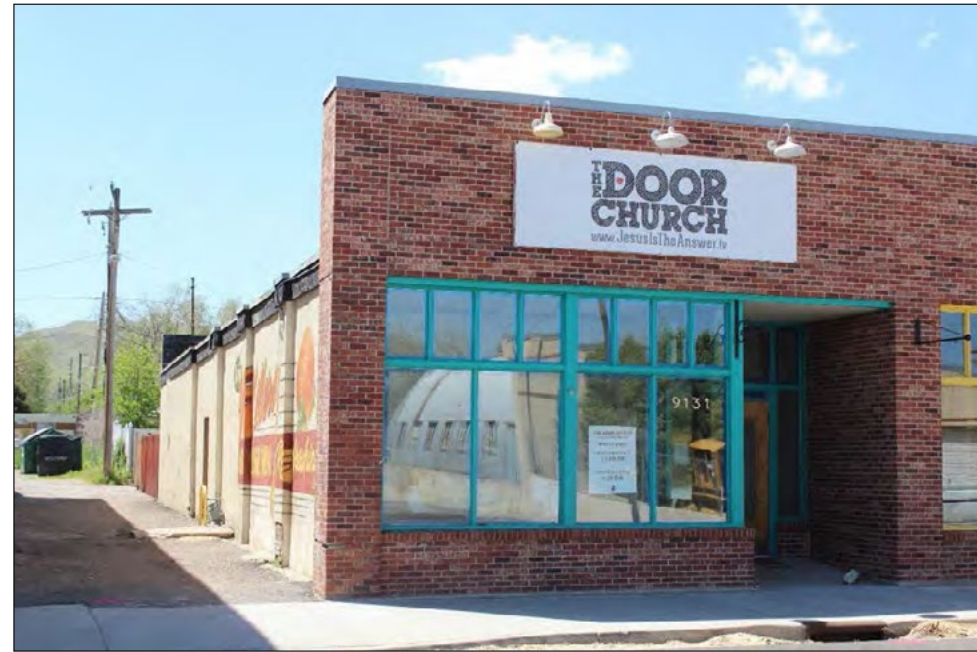
41 of 56 9131 West Magna Main Street, contributing, north and east elevations, facing south.
