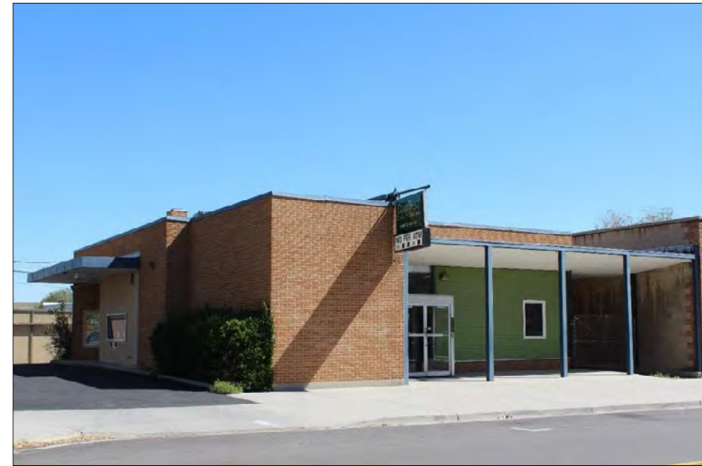
18 of 56 9024 West Magna Main Street, contributing, south and west elevations, facing north-northeast.
