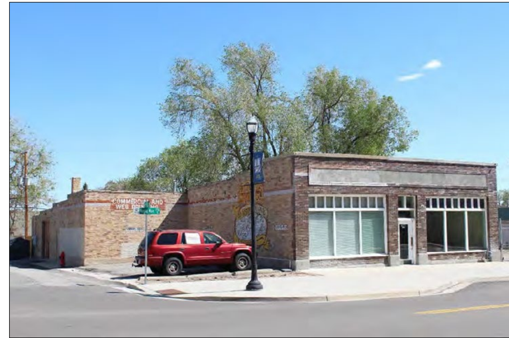
10 of 56 8980 West Magna Main Street, contributing, south and west elevations, facing north.
