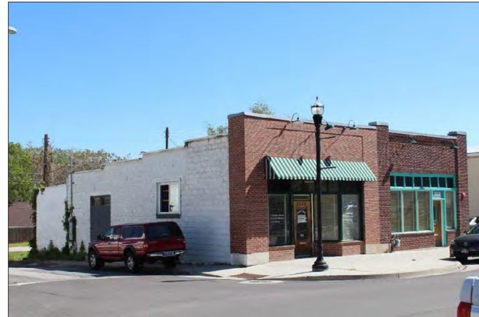
40 of 56 9124 West Magna Main Street, contributing, south and west elevations, facing north-northeast.
