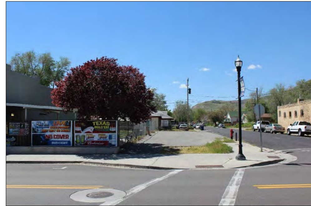
12 of 56 8997 West Magna Main Street, non-contributing, facing south.
