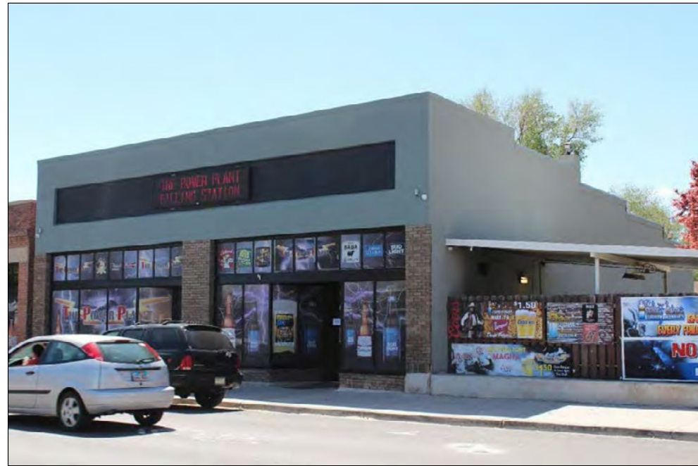
11 of 56 8987 West Magna Main Street, non-contributing, north and west elevations, facing south-southeast.
