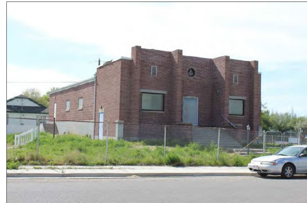
48 of 56 2618 South 8950 West Street, contributing, south and east elevations, facing west-northwest.
