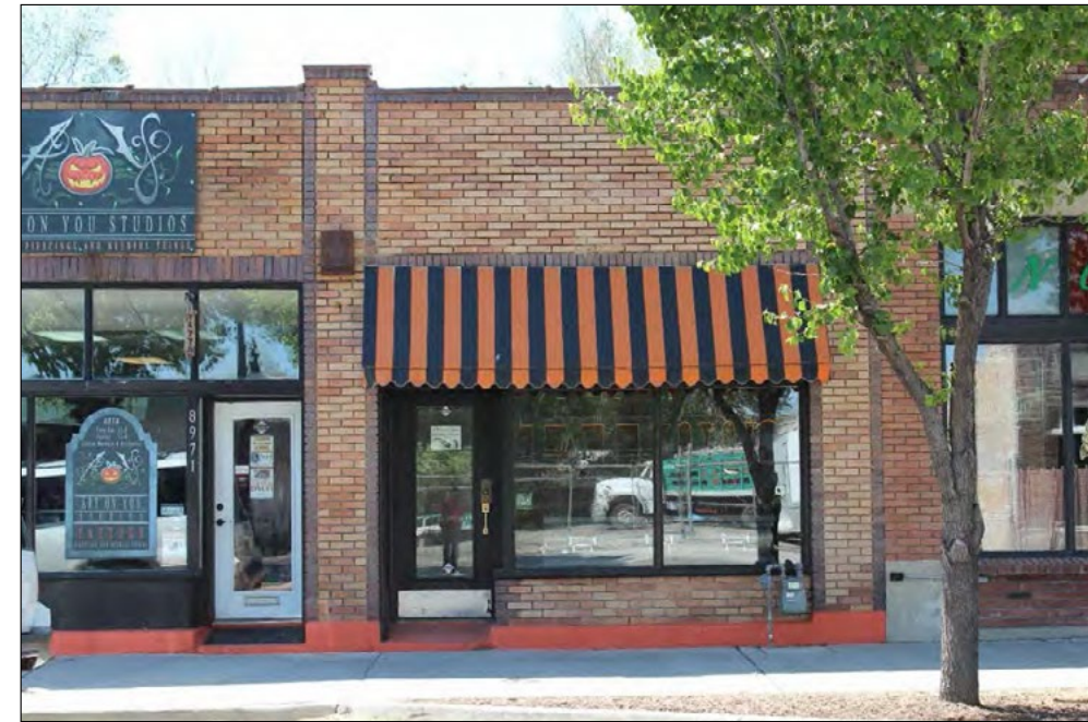
8 of 56 8975 West Magna Main Street, contributing, north elevation, facing south.
