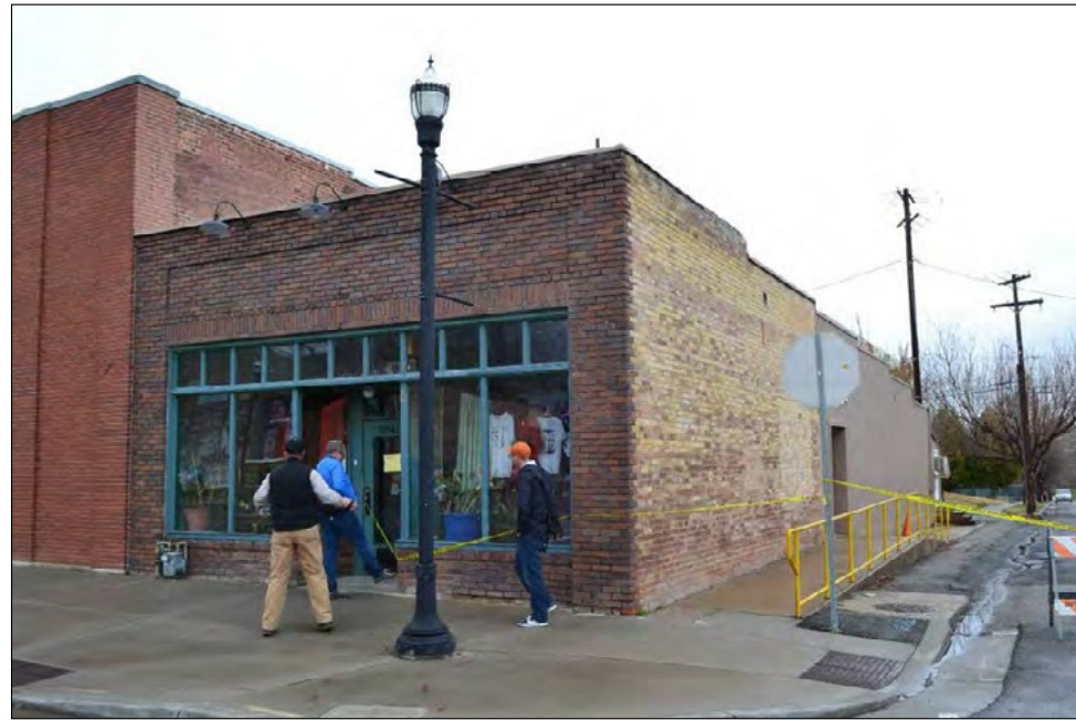
21 of 56 9046 West Magna Main Street, contributing, after earthquake, south and east elevations, facing north.
