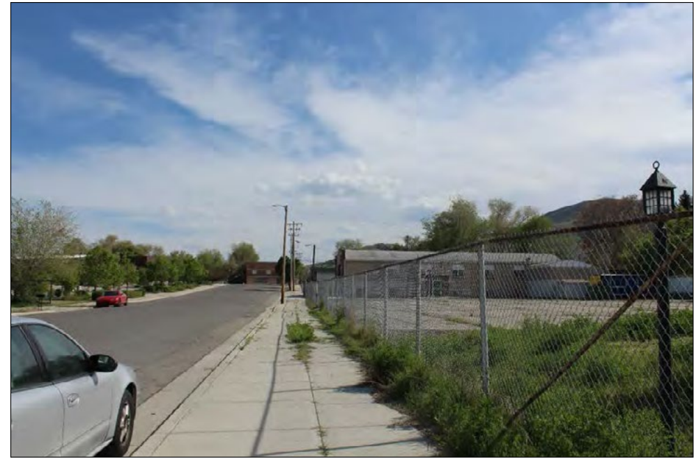
56 of 56 Overview of district from north boundary, facing south. Photographer: K. Hovanes Date photographed: 5/10/20
