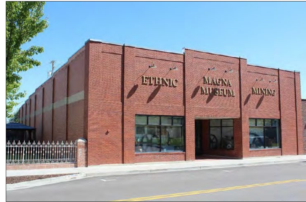
22 of 56 9056 West Magna Main Street, contributing, south and west elevations, facing north-northeast.
