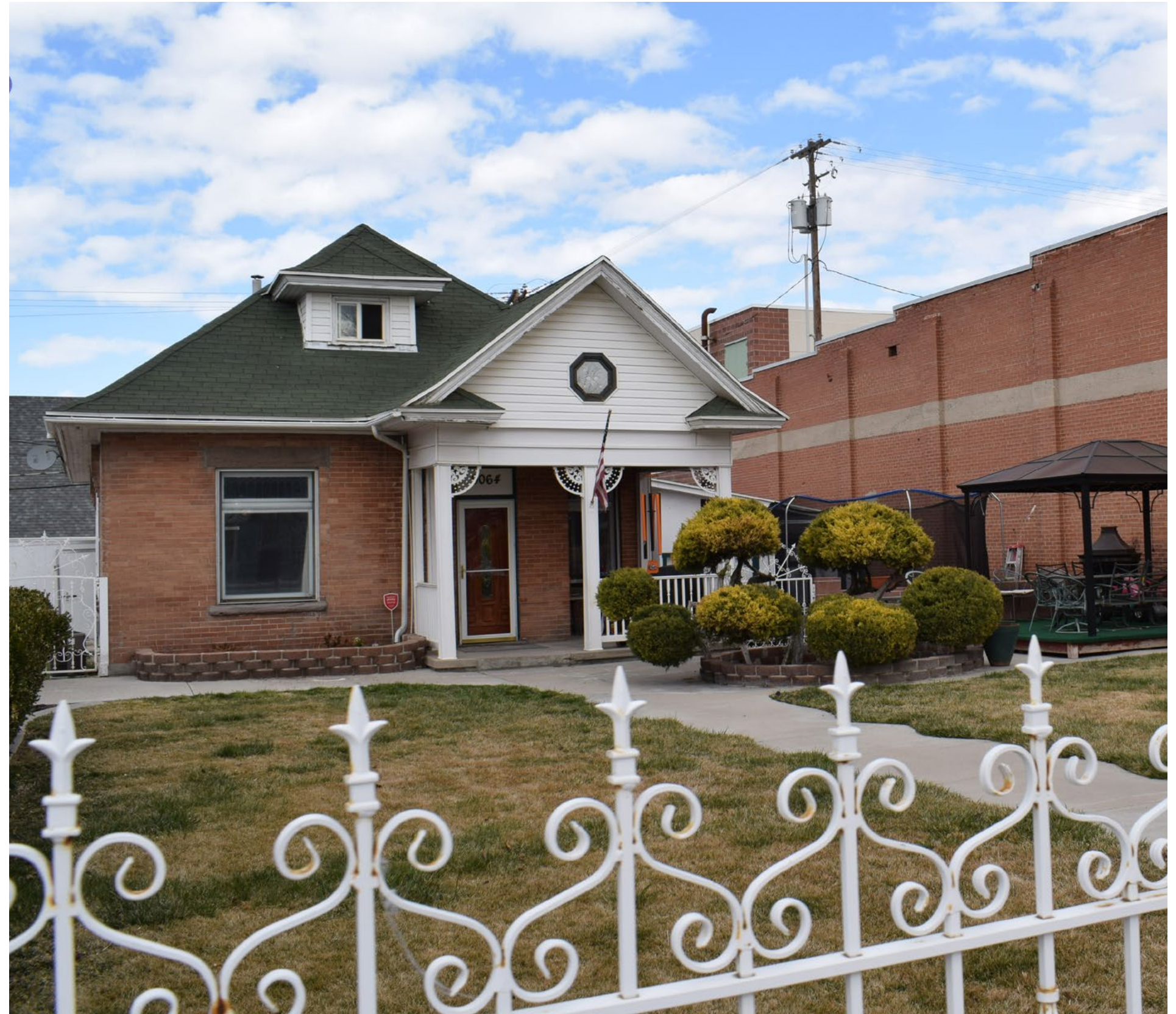
A historic single family structure in Magna (GSBS Consulting)
