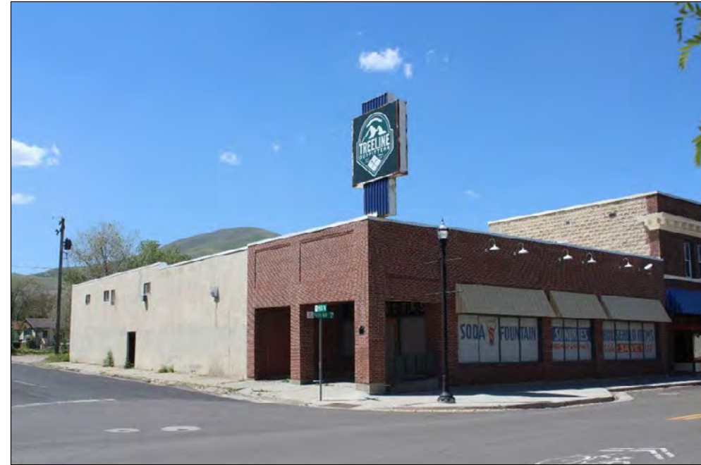
34 of 56 9105 West Magna Main Street, contributing, north and east elevations, facing southwest.
