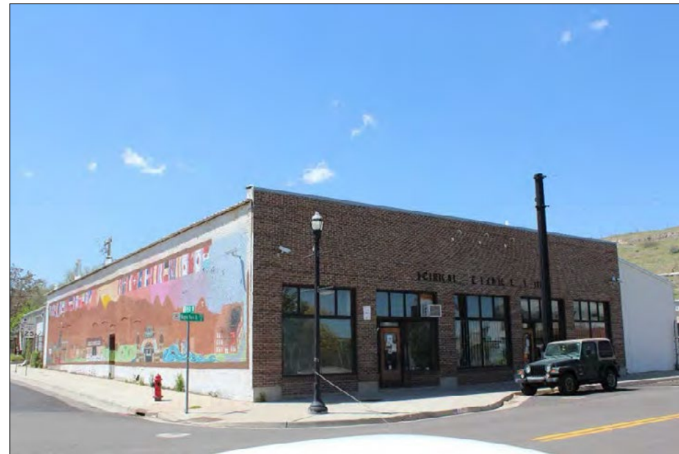
47 of 56 9187 West Magna Main Street, contributing, north and east elevations, facing south-southwest.
