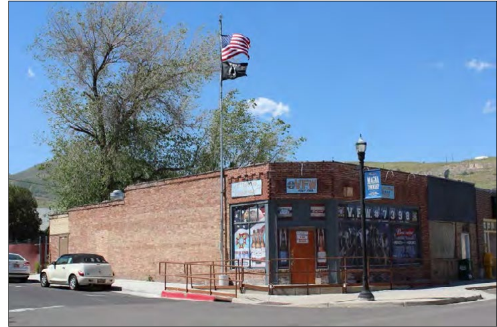
24 of 56 9057 West Magna Main Street, contributing, north and east elevations, facing southwest. Photographer: K. Hovanes Date photographed: 5/12/17
