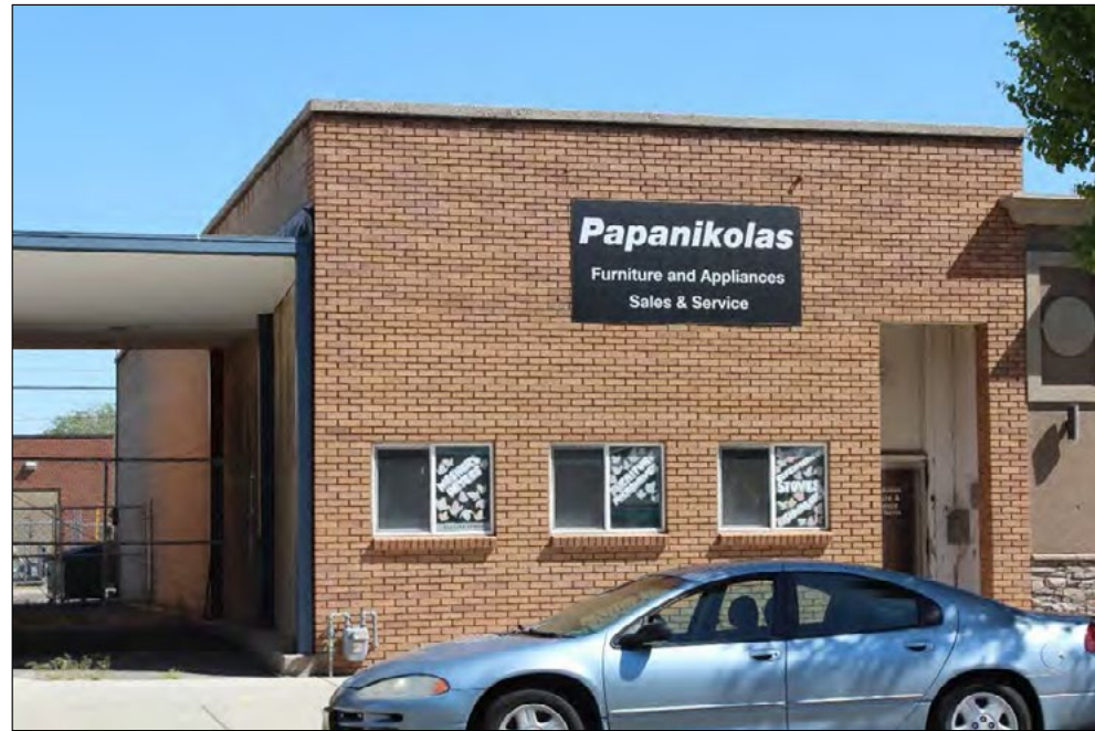
17 of 56 9014 West Magna Main Street, contributing, south and west elevations, facing north.
