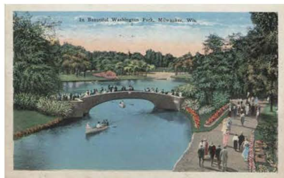
Washington Park lagoon bridge Image source: Villa Terrace Decorative Arts Museum
