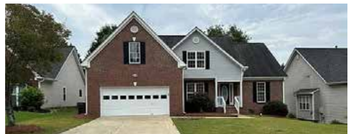
Figure 5.25. Large Lot Single Family Home in Lawrenceville
