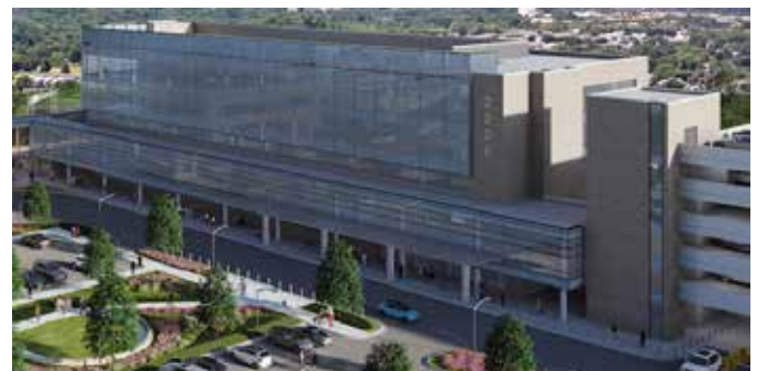
Source: Northside Hospital
