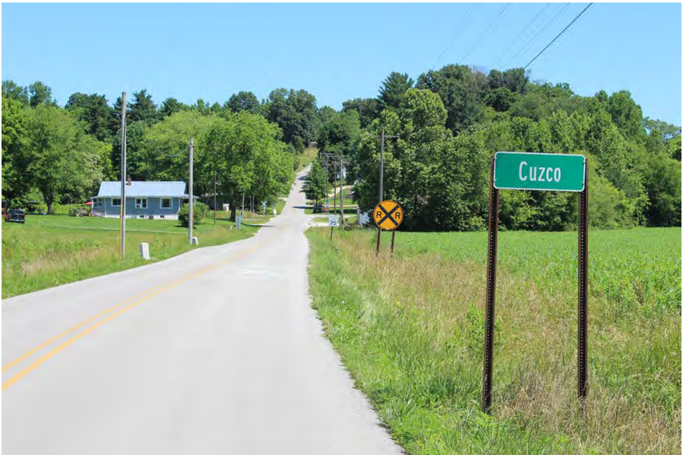
Figure 52 - Route 1C includes the construction of a new train platform at Cuzco and a new two-mile sidepath to connect the French Lick Scenic Railroad to the Patoka Lake Army Corps of Engineers property.
