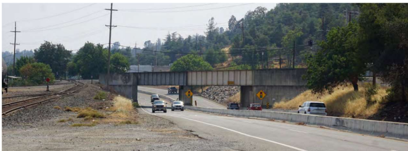
Southbound view of the “mousehole” at the UPRR freight rail overcrossing on SR 273. Image Source: S. Market Street (SR 273), Redding Summary and Recommendations Report, 2021.
