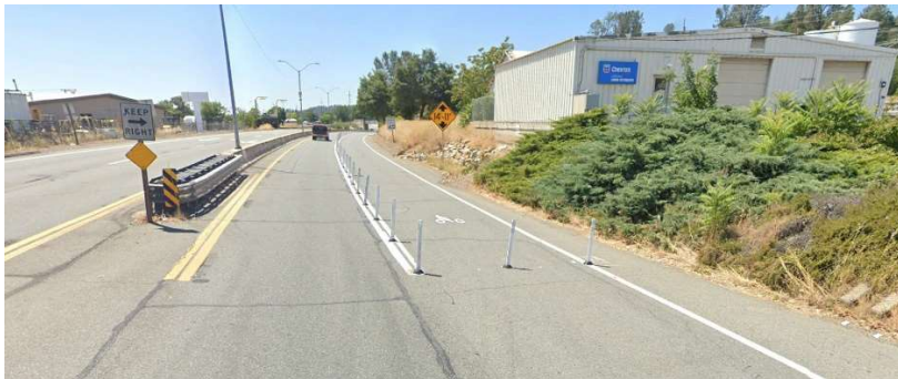
Start of quick build multiuse path on Southbound SR 273. Image source: Google, 2023.
