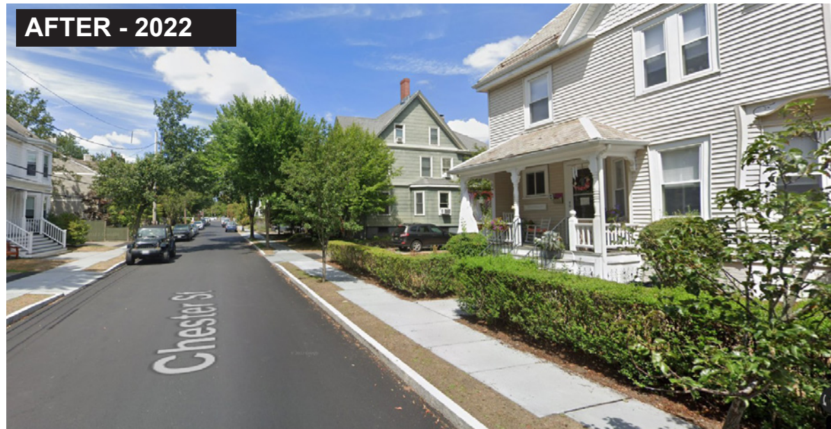
A recent roadway project added granite curbing, a planter strip, and a concrete sidewalk to beautify the street and improve the pedestrian experience.
