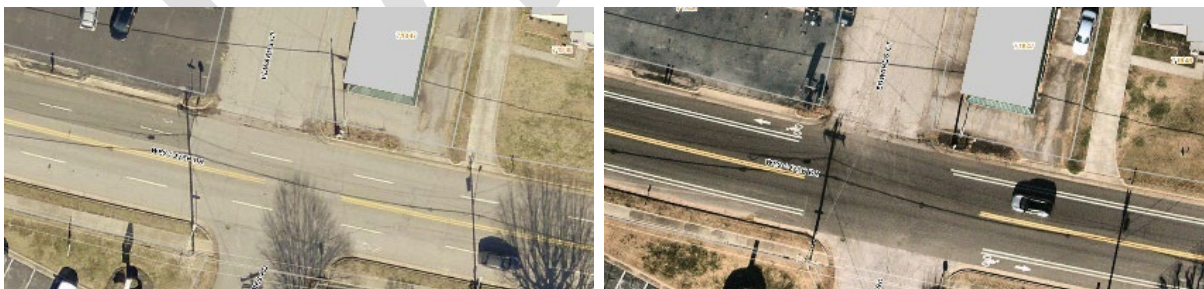
Figure 21. Before and After images of Westover Drive Roadway Reconfiguration.
