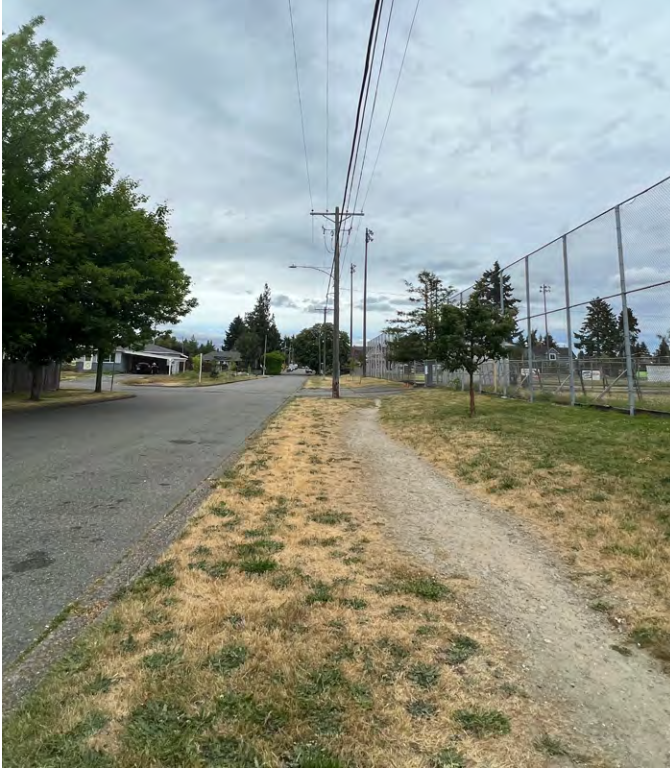
State Street along the west edge of the fields will receive new paving, sidewalks, curb ramps & vegetation as part of upcoming Tacoma Streets Initiative Improvements.
