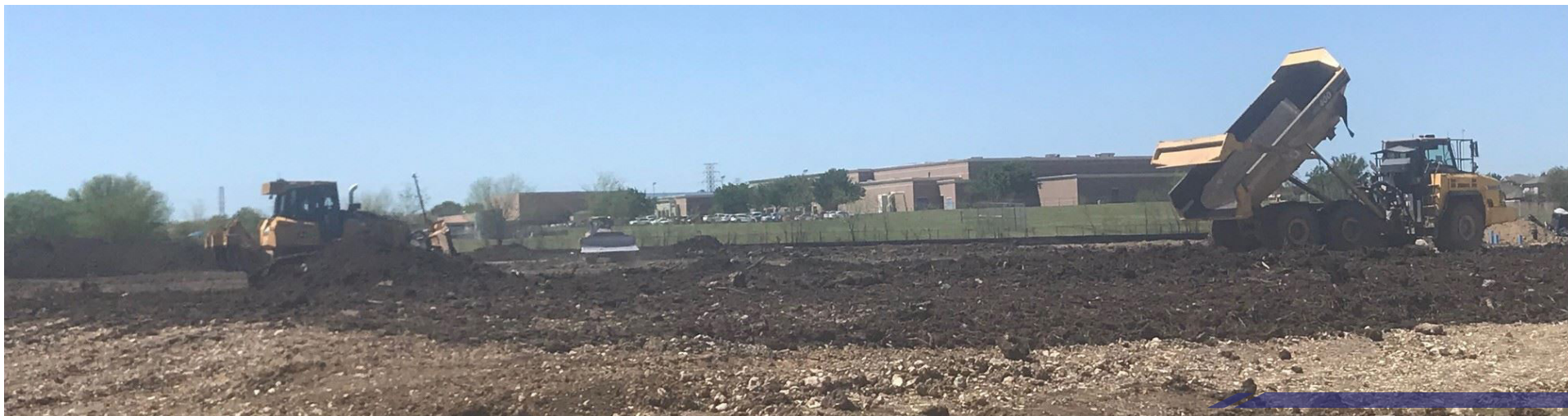
Construction Progress Photo of the UCD Mixed-Use Development
