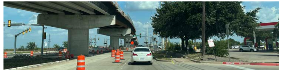
Bailey Boswell Road and Overpass Construction
