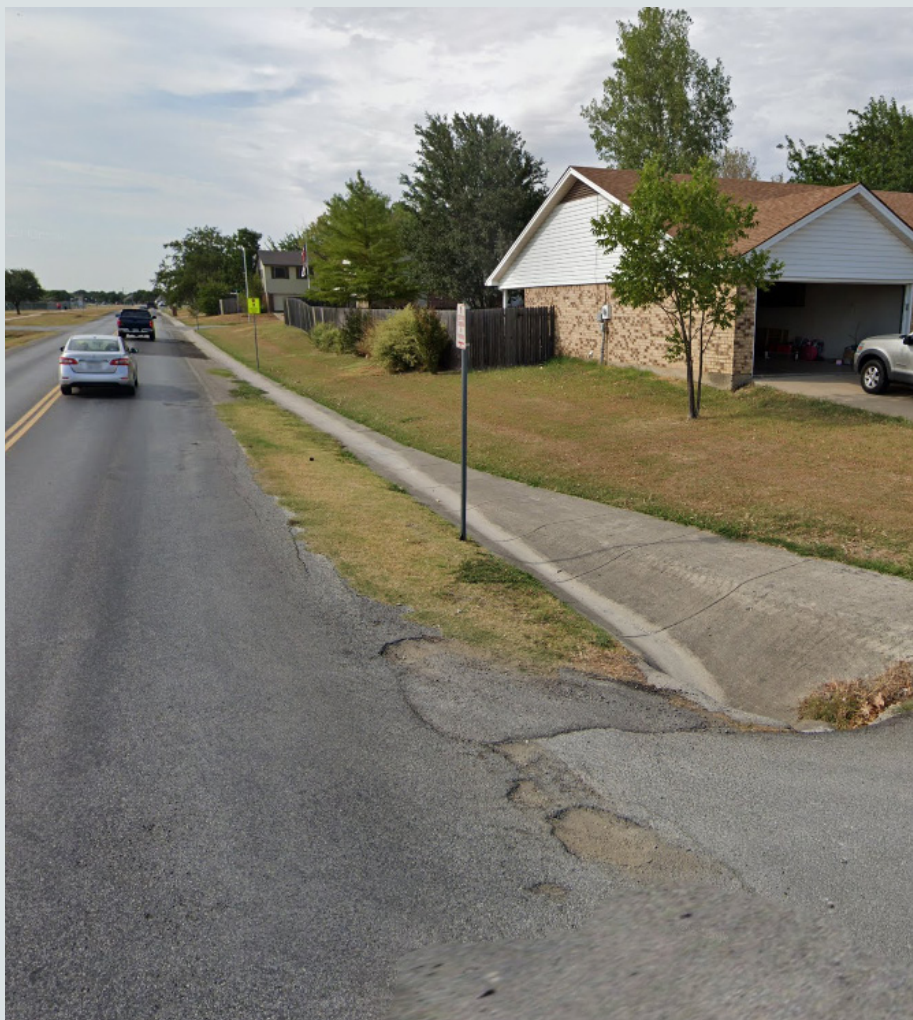
Stormwater Infrastructure along Knowles Drive
