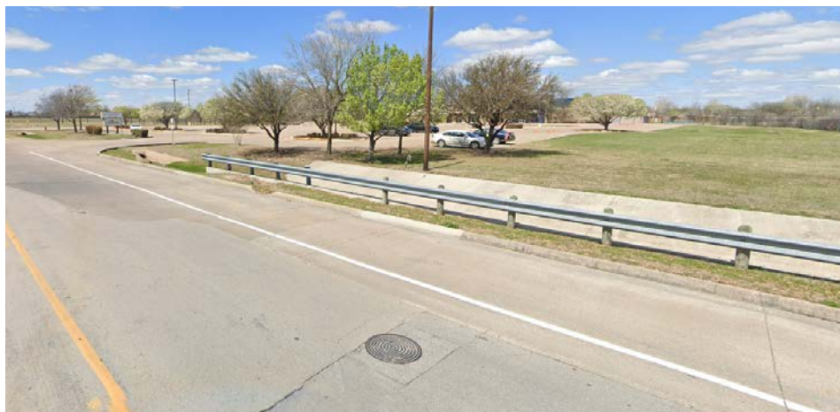
Saginaw Culvert Along W McLeroy Boulevard
