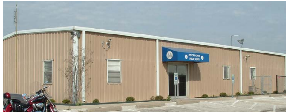
Saginaw Public Works Building
