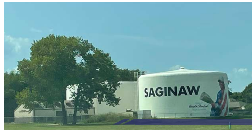
Saginaw Ground Storage Tank
