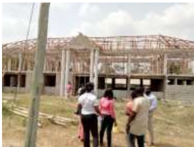
Construction of 1No. 2-storey Administration Block at Kumasi Academy
