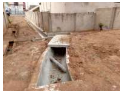
constructed storm drain at the administration block
