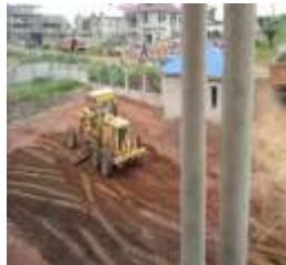
Gravelling of forecourt of the
