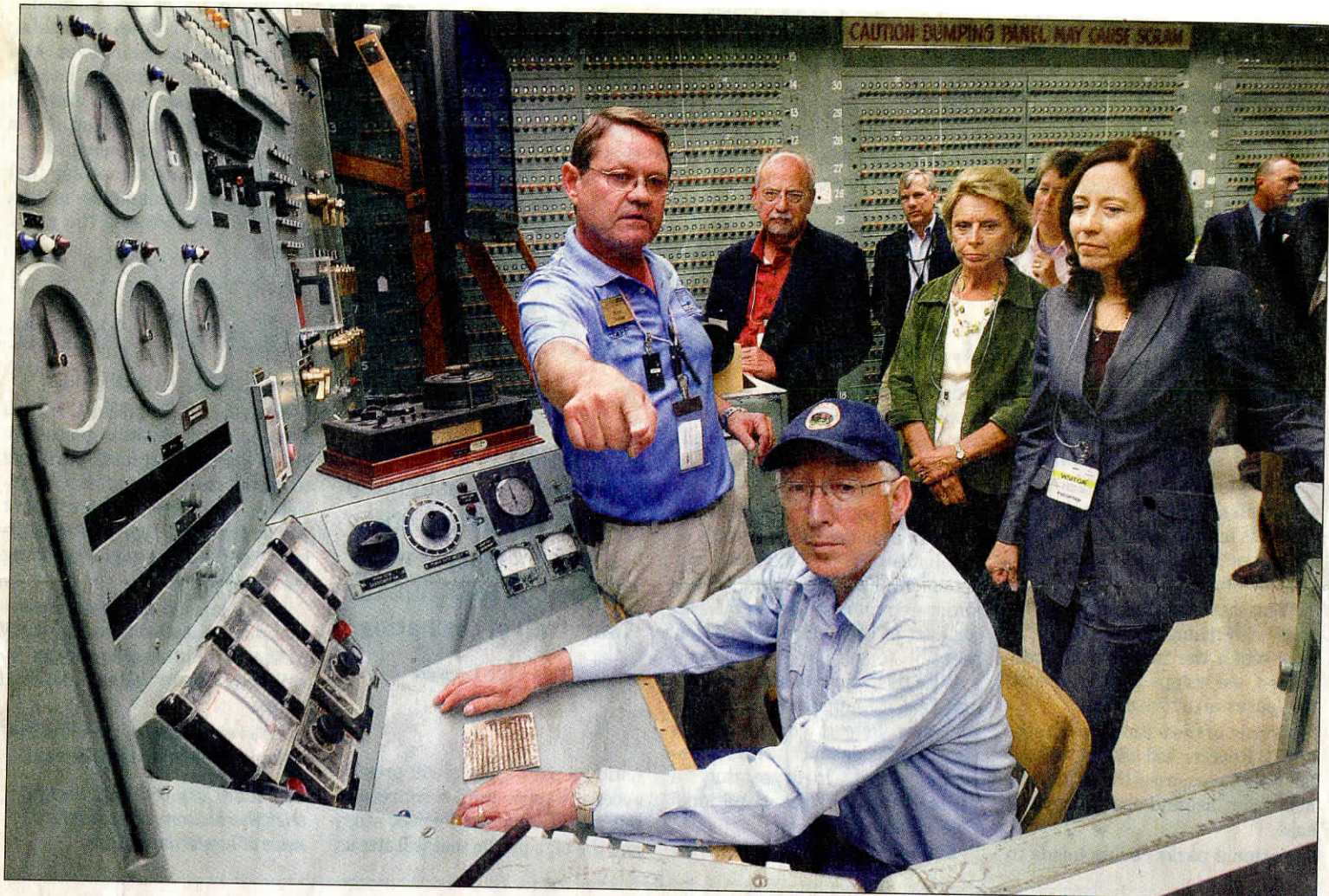
Secretary of the Interior Ken Salazar, seated in the operator's chair in the B Reactor, listens as Russ Fabre, B Reactor tour manager, left, explains the workings of the reactor's control panel Sunday during a tour at Hanford as Gov. Chris Gregoire, second from right, Sen. Maria Cantwell, right, and Rep. Doc Hastings, second from left, listen. See a photo gallery at tricityherald.com. Photos by Paul T. Erickson | perickson@tricityherald.com
