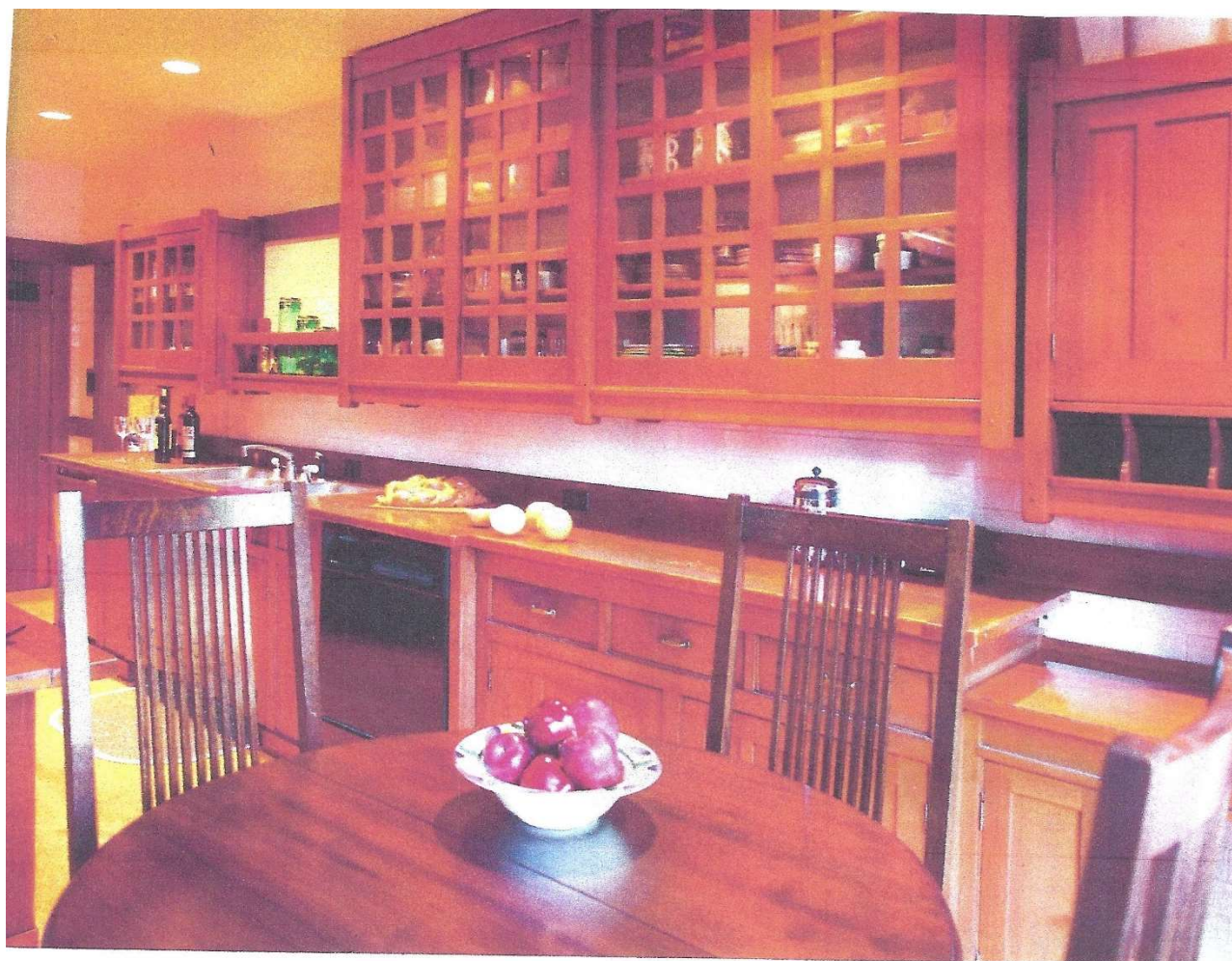
Restored in the late 1970s, the kitchen fits the tenor of the home, with cabinets that match original units in the butler's pantry. The upper doors slide on rails—a concession Greene & Greene made after the San Francisco earthquake to prevent cupboard doors from swinging open during a temblor.
