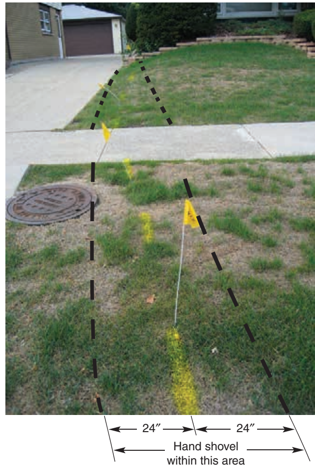
Figure 2-12. The local utilities mark the position of underground service lines. You may use powered equipment to excavate no closer than 24" to the markings. Any digging within the 24" zone must be done with a hand shovel.
