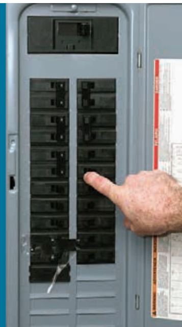
Figure 2-16. Turn off the power to an individual household circuit by shutting off the circuit's breaker in the home's main service panel.
