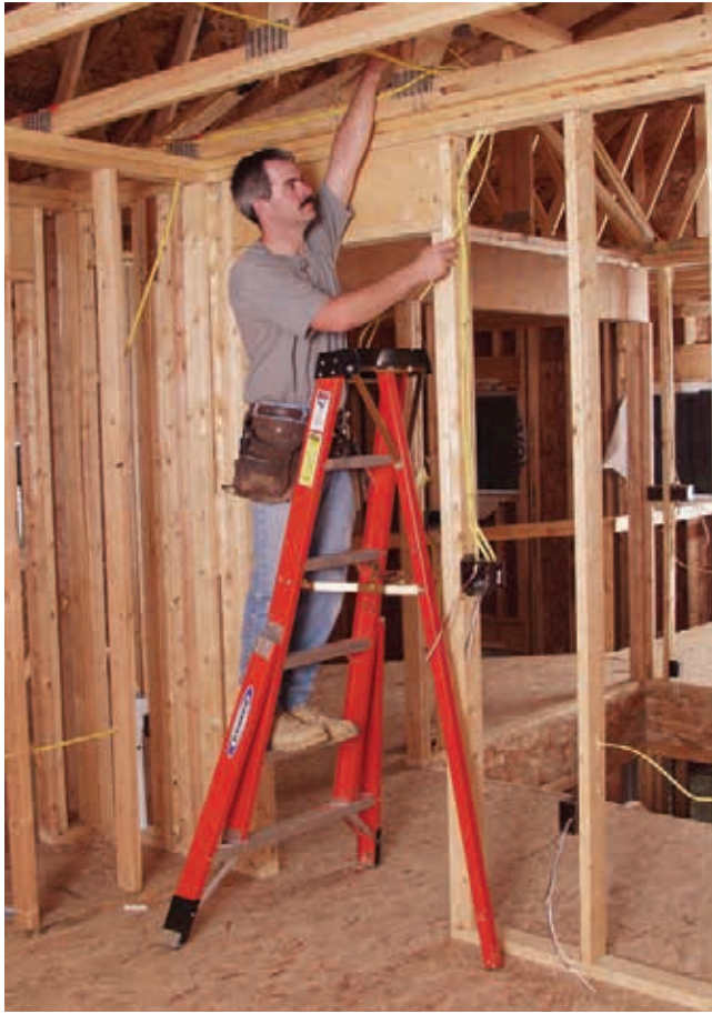
Figure 2-7. Always face the ladder and never stand on the top rung.
