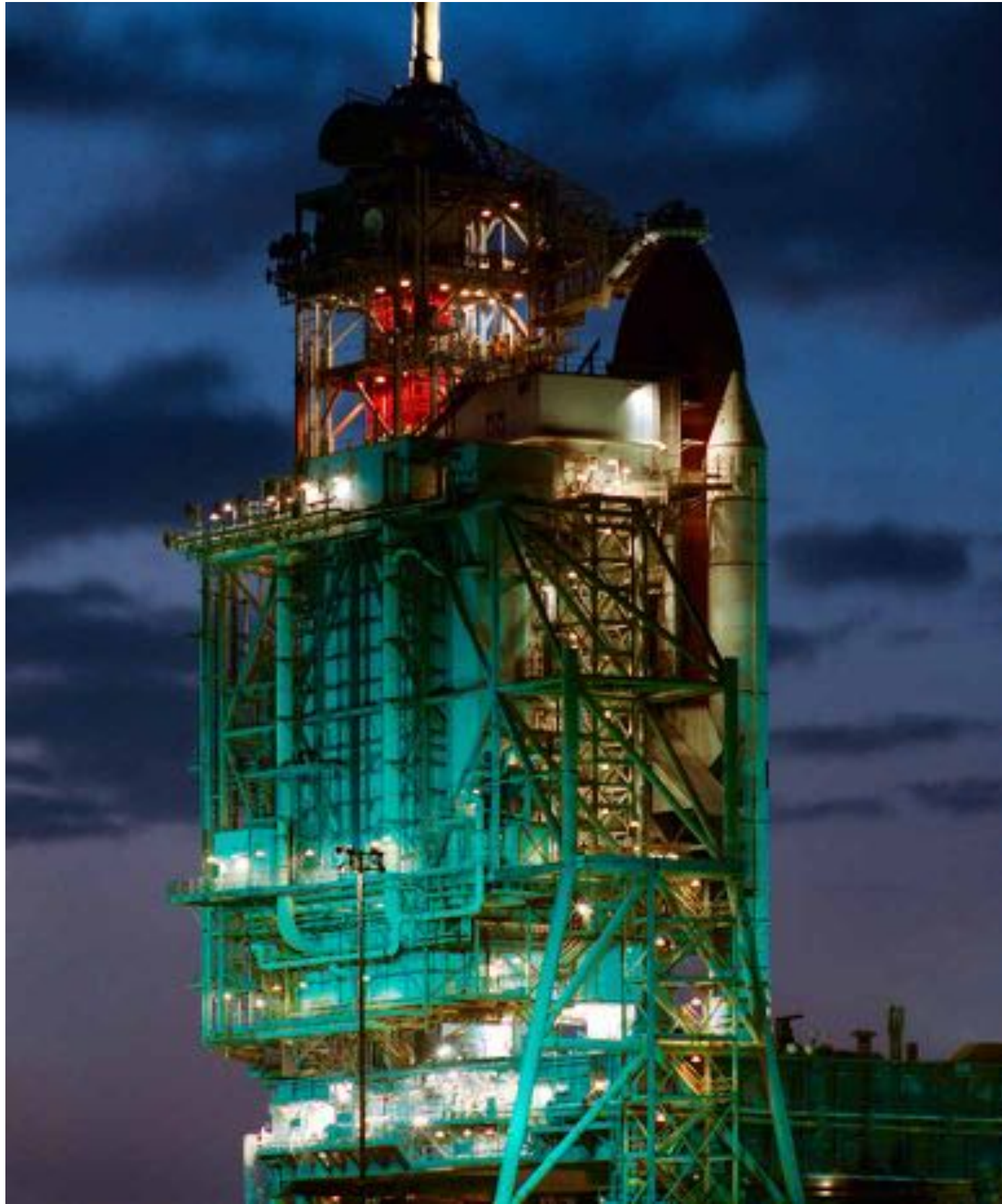
Challenger, Closed Service Structure Launch Complex 39A, 1984
