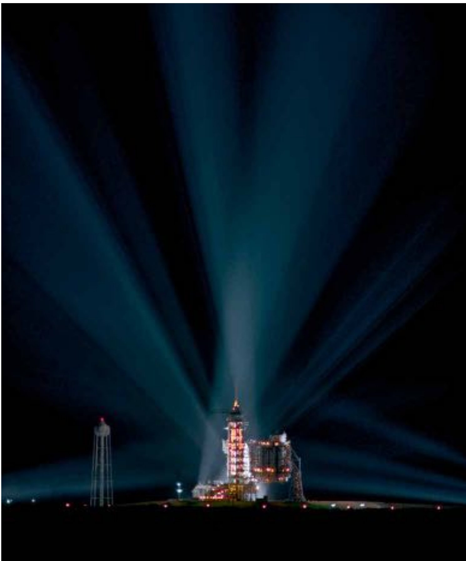
Launch Complex 39A, Xenon Lights Press Site, 1985
