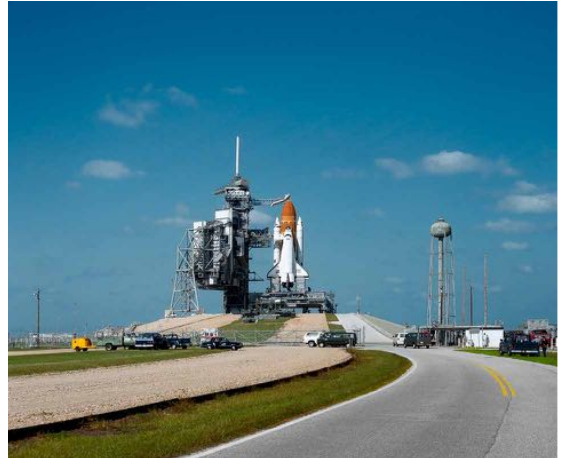
Discovery, Crawler Way Pad 39A Entrance, 1984
