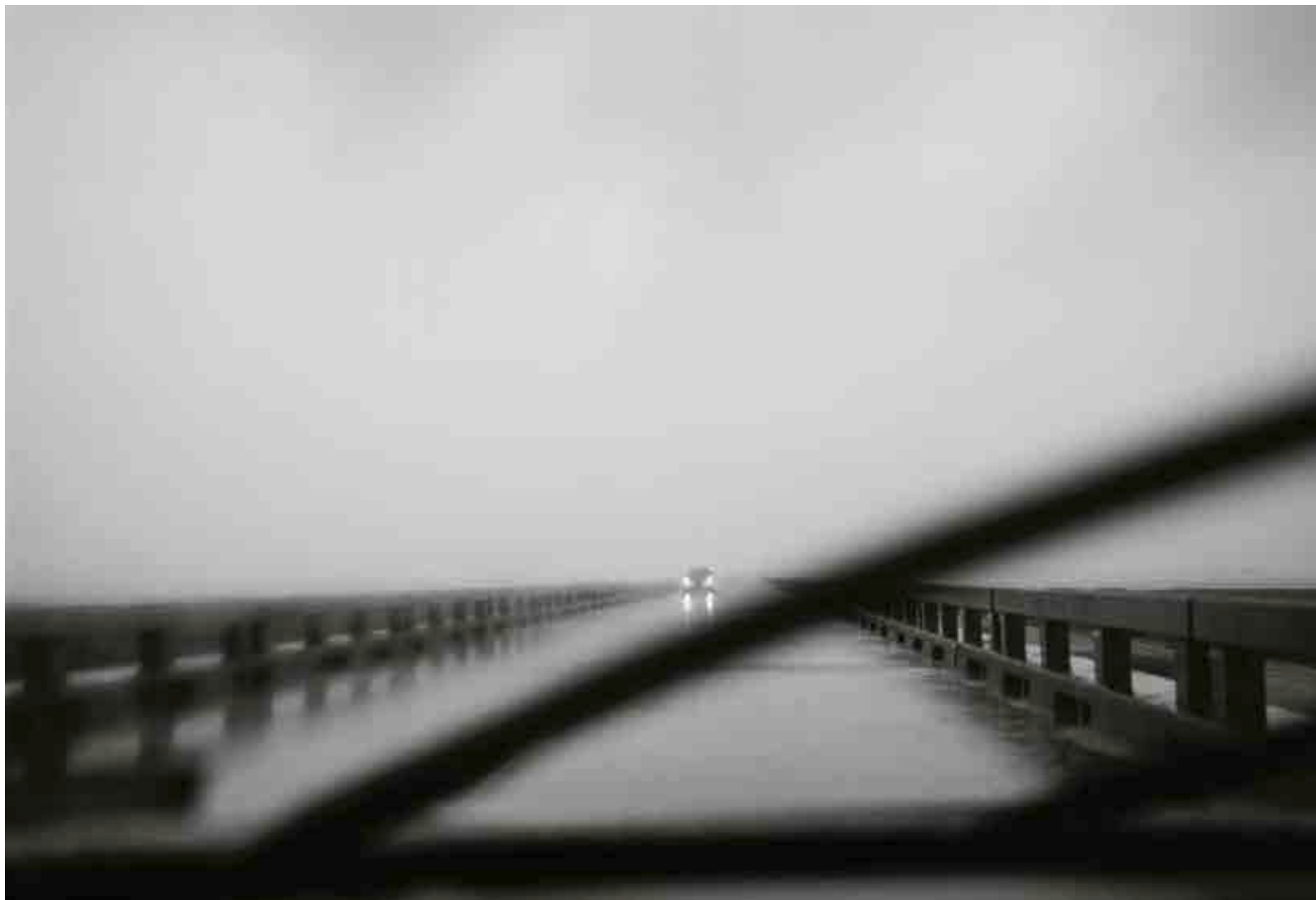
San Luis Pass-Vacek Toll Bridge on a rainy day, Galveston Island, Nov. 2015
