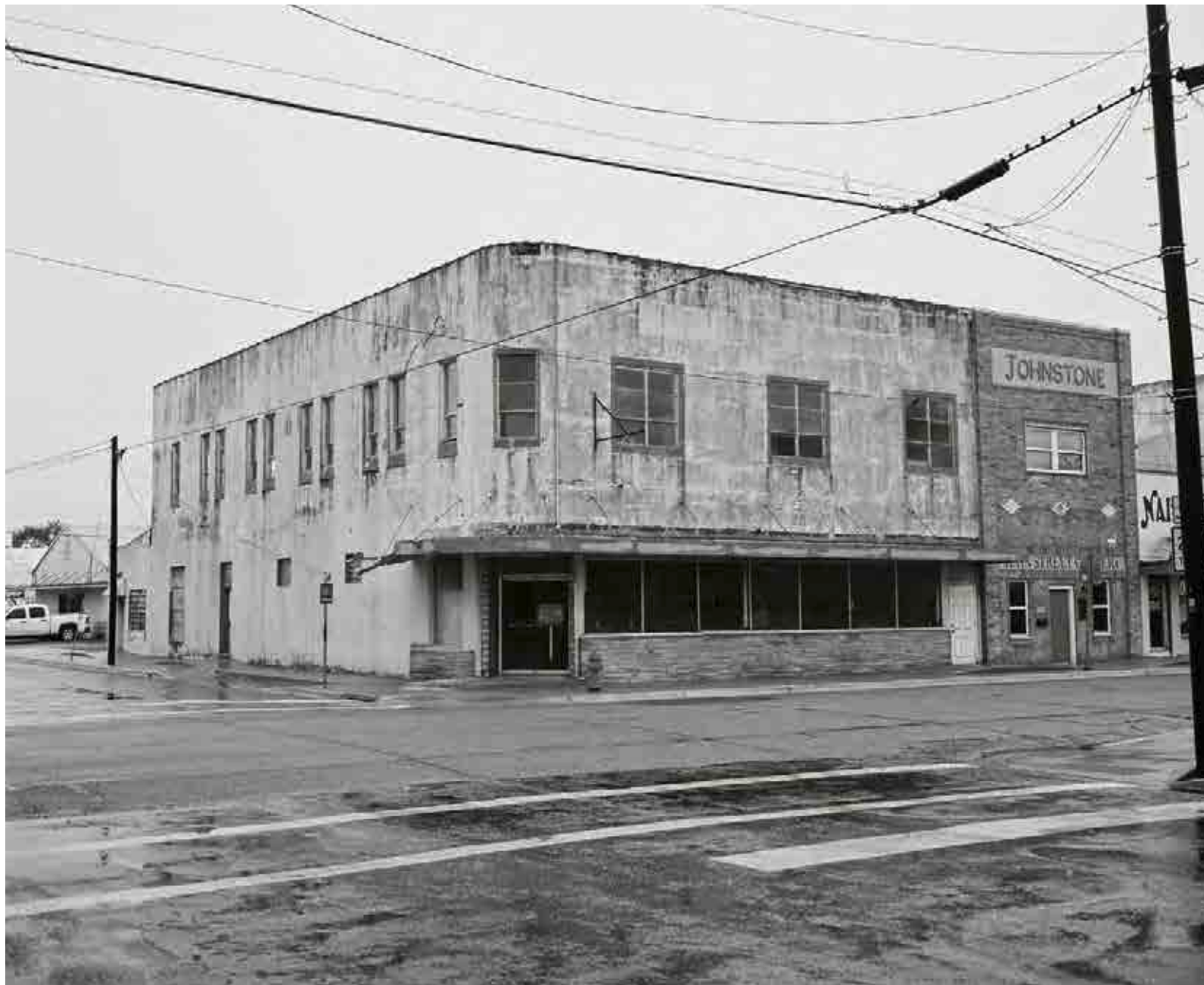
Johnstone Building, E. Main Street, Port Lavaca, Oct. 2015
