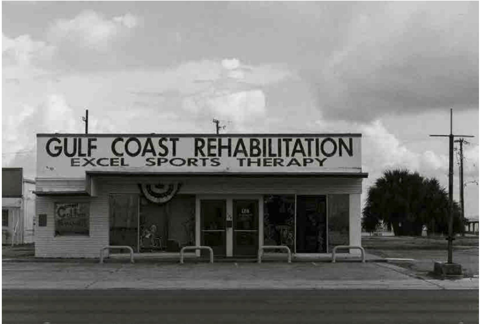
Gulf Coast Rehabilitation Center, 128 N Commerce Street, Port Lavaca, Nov. 2024
