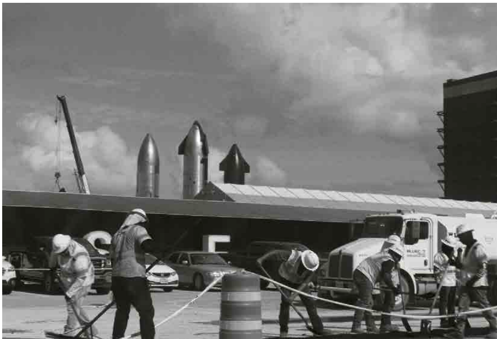
Asphalt work in front of the SpaceX rocket factory, Boca Chica, Oct. 2024
