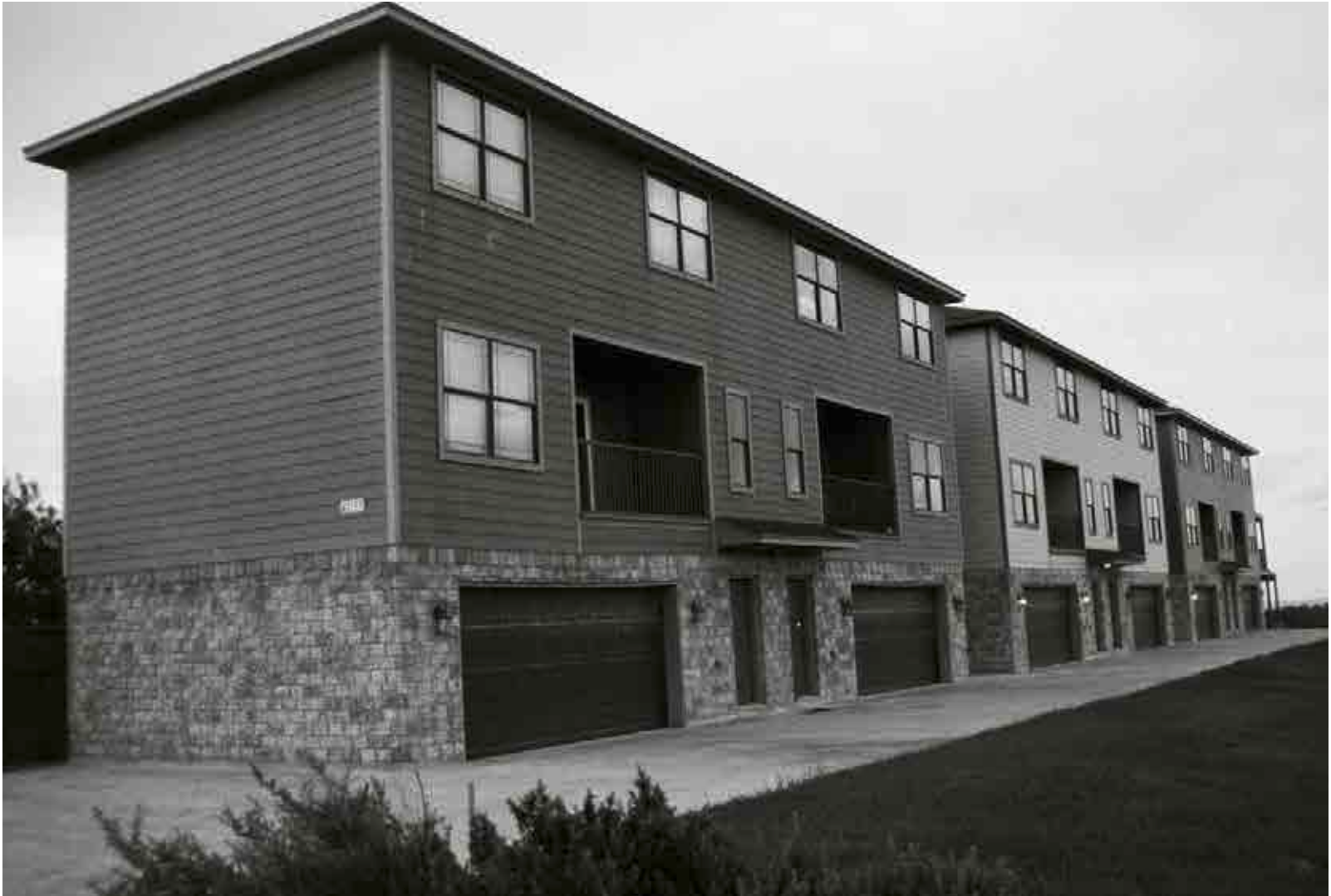
Abandoned apartment block, Laguna Heights, Oct. 2024
