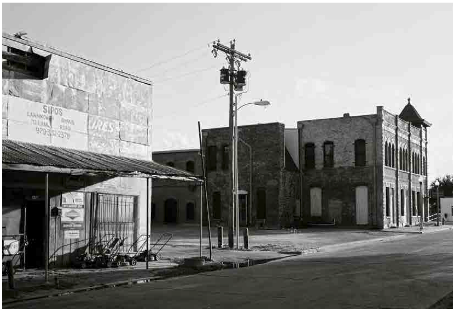
East Railroad Street, El Campo, Oct. 2024
