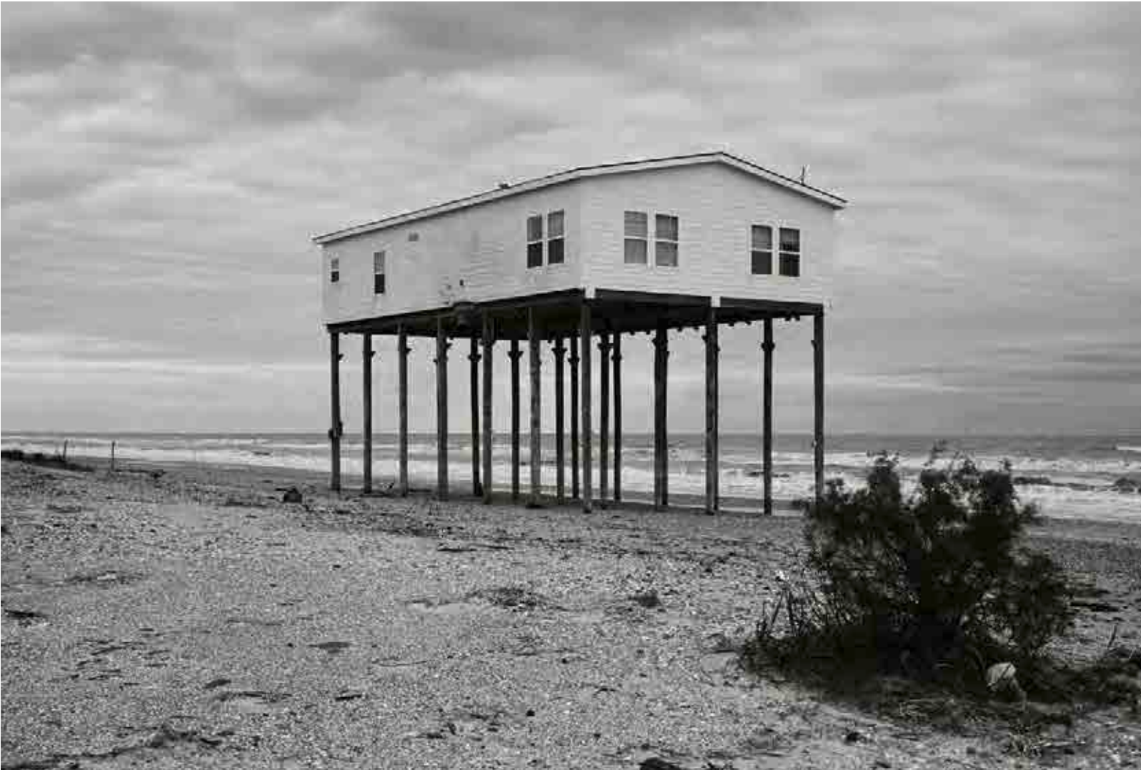
Beachfront house on stilts, SH 87 near High Island, Bolivar Peninsula, Nov. 2022
