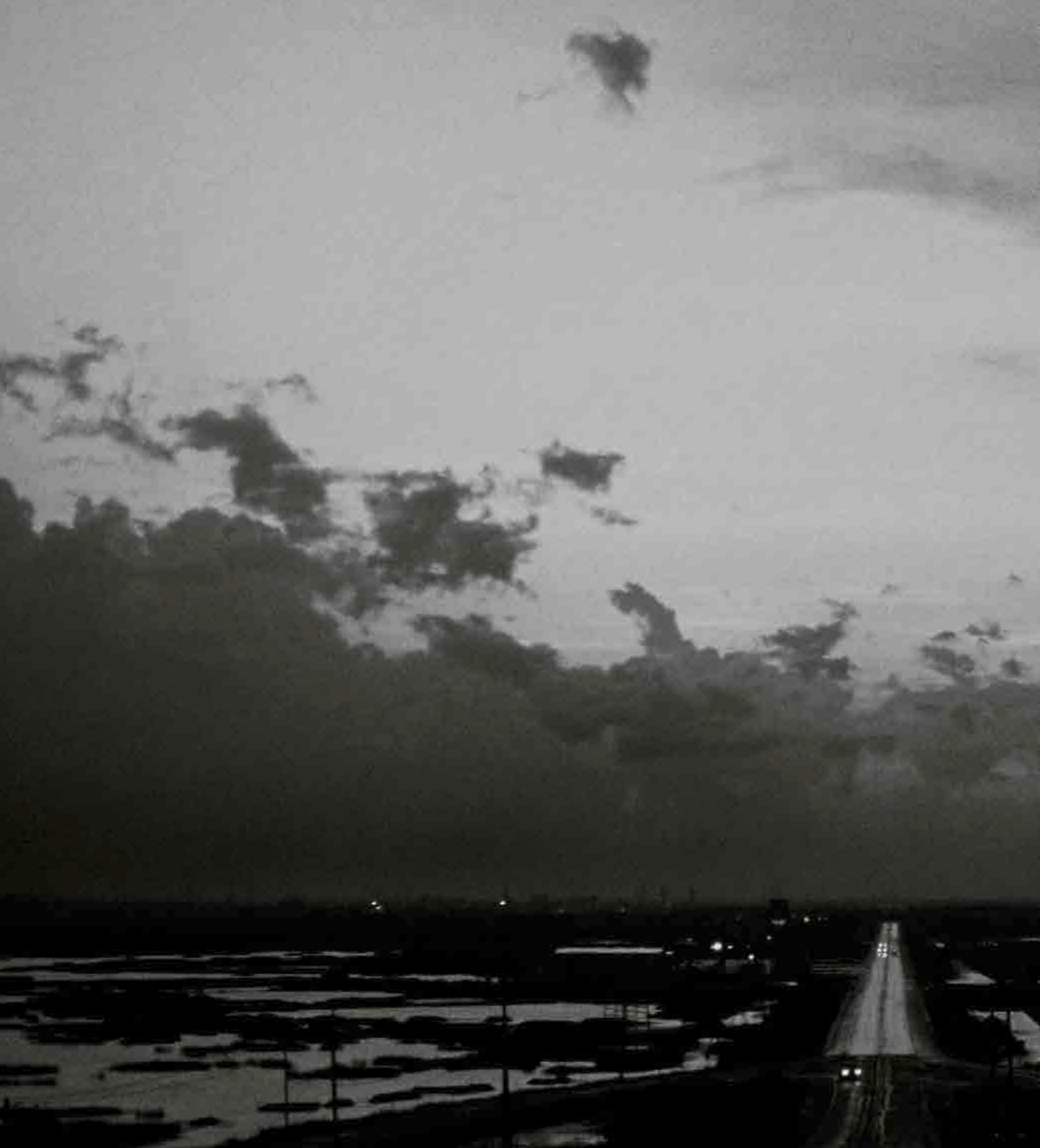
Intracoastal Waterway bridge on TX 332 (northbound view), Freeport, July 1987
