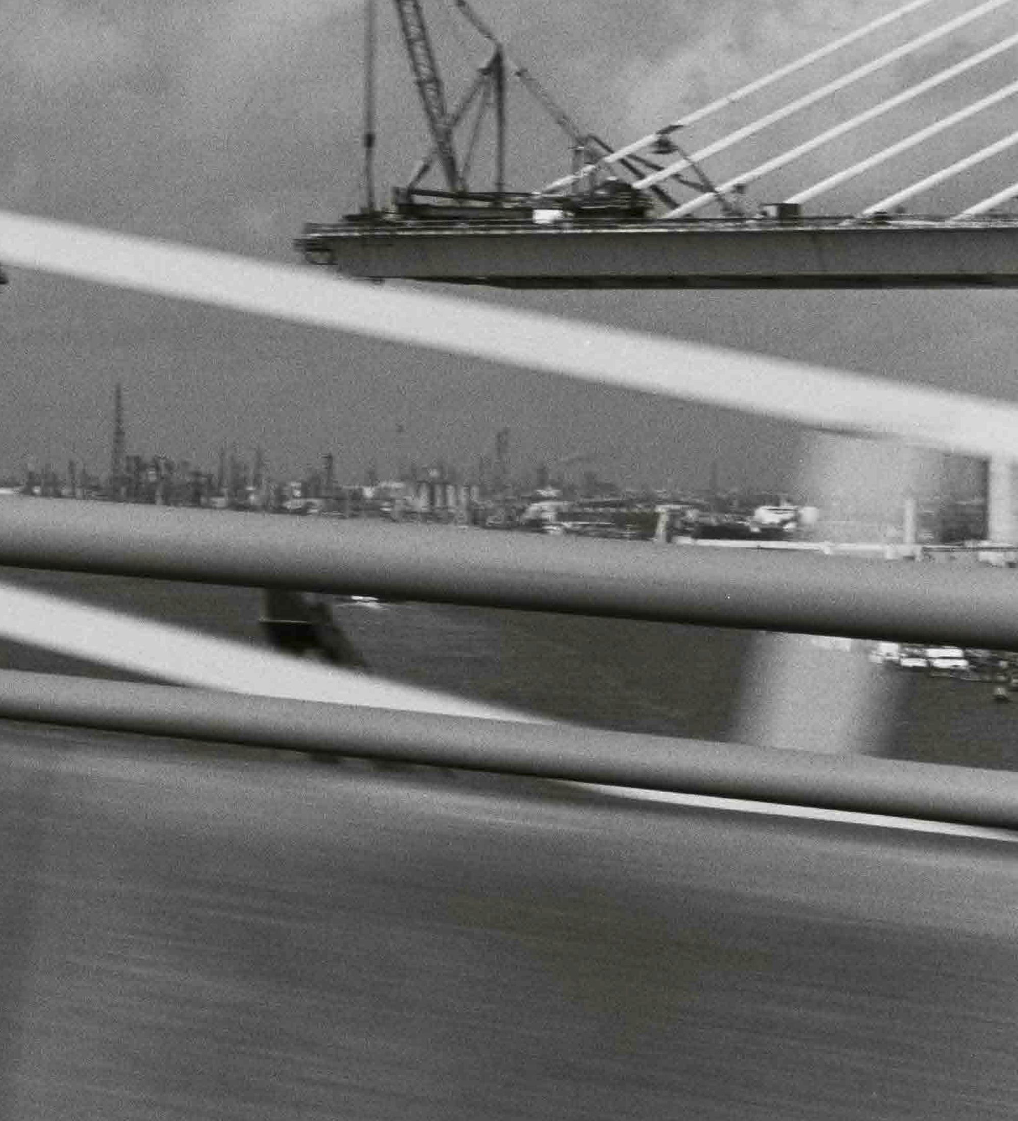
New Harbor Bridge on US 181 under construction, Corpus Christi, Nov. 2024
