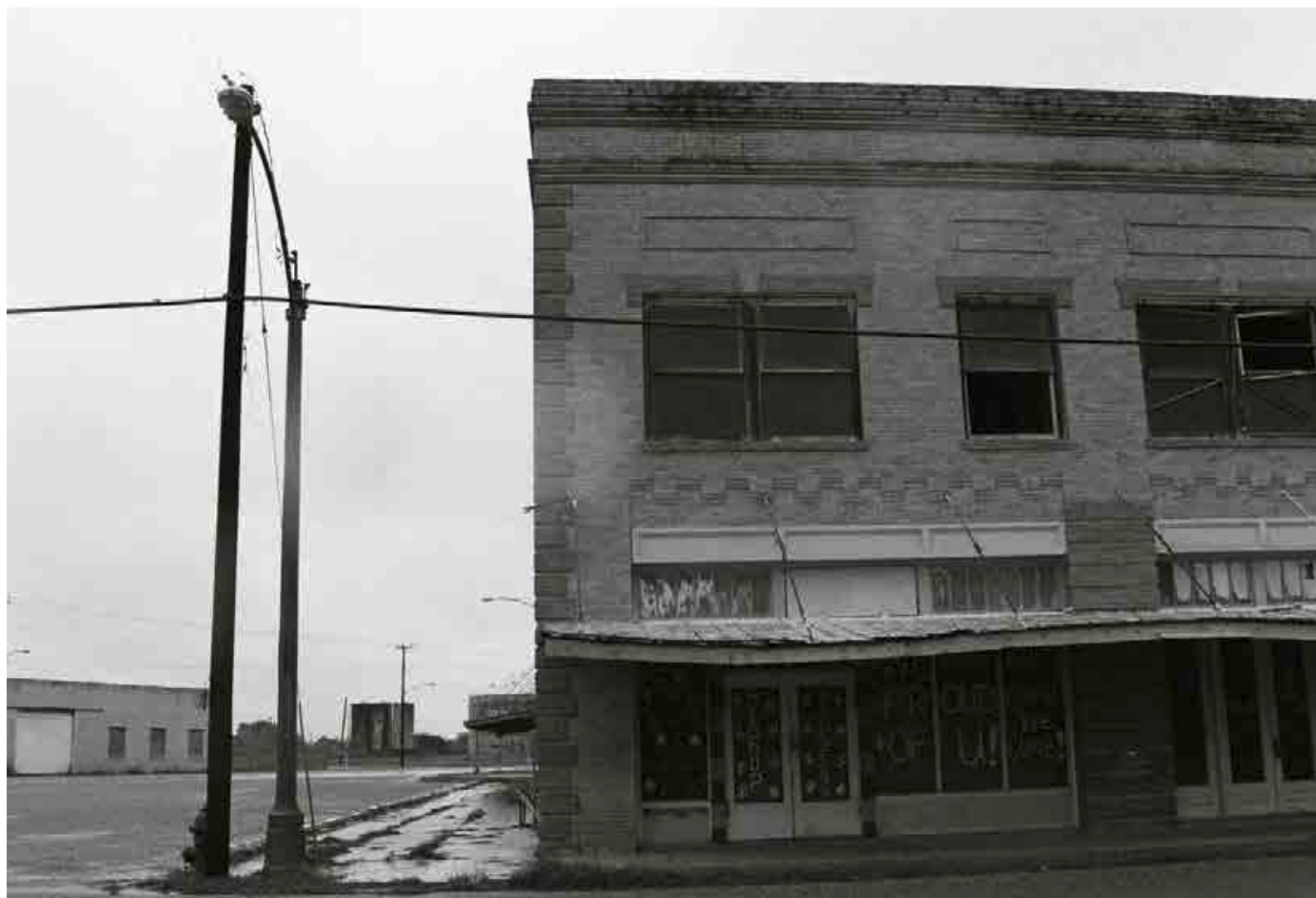
"WE ARE PROUD OF YOU", abandoned building on East Main Street, Bishop, Nov. 2023
