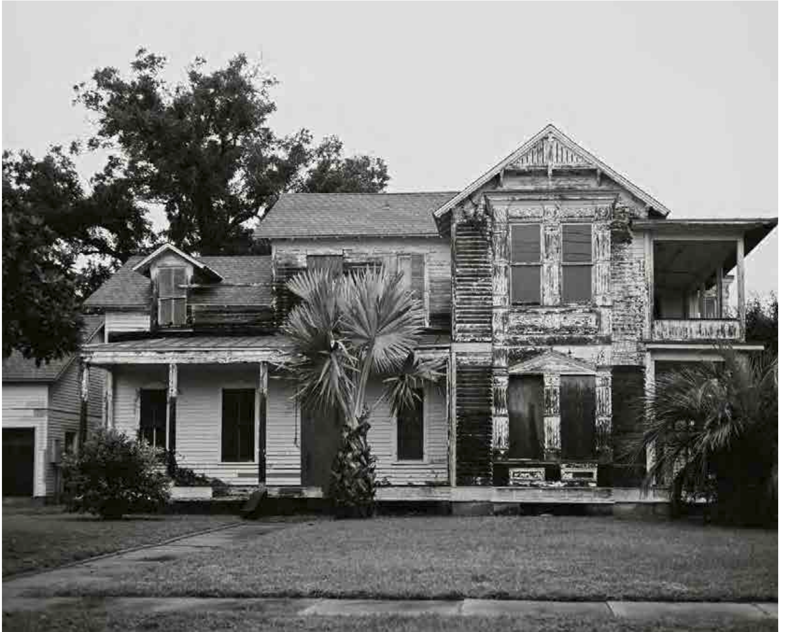
Weathered mansion, Palacios, Oct. 2015
