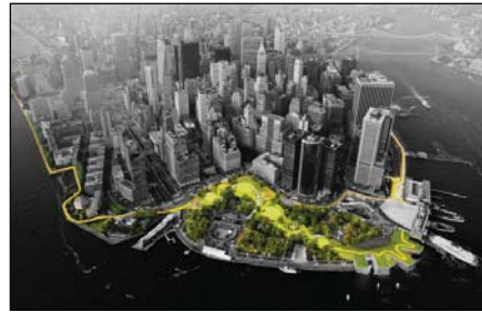
THE BATTERY BERMS
