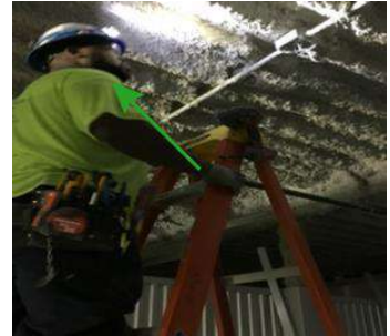
Eye protection is worn when on electrical box work above his head.
