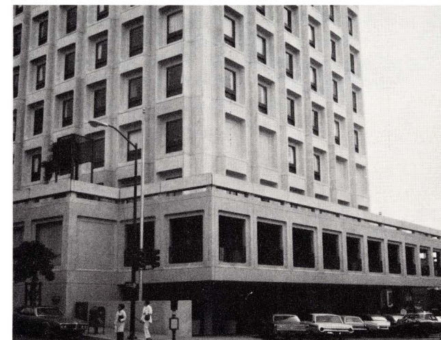
St. Francis Hospital
