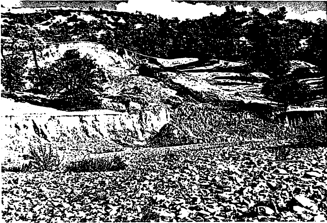
Figure 2.35. Landslide along left bank Cache Creek, River Mile 21.34.
