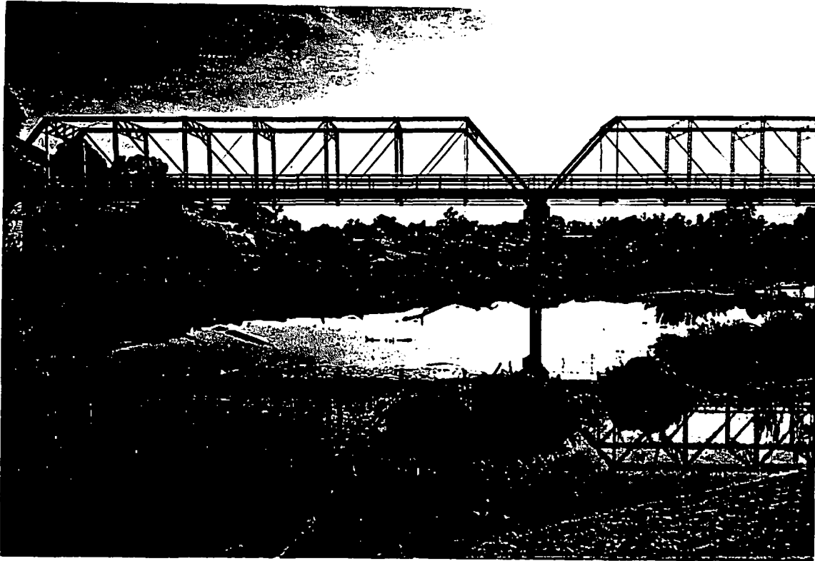
Figure 2.33. Guinda Bridge, River Mile 20.0 (looking downstream).
