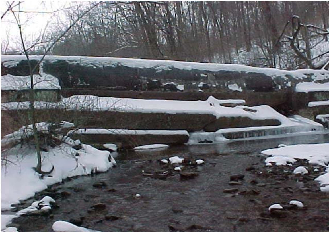
Photo 1. Alameda Park dam (10-007) prior to removal, winter 2005.
