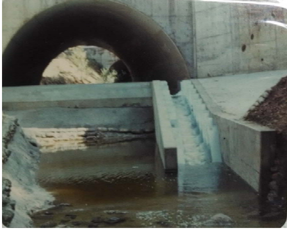
Photos after construction of the 1970's denil ladder
