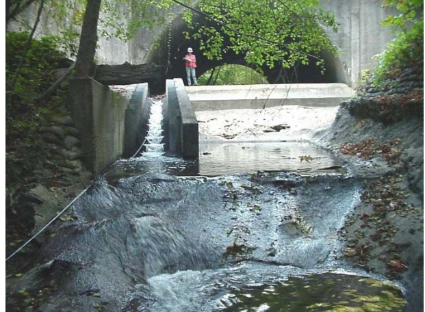
Photos after construction of the 1970's denil ladder
