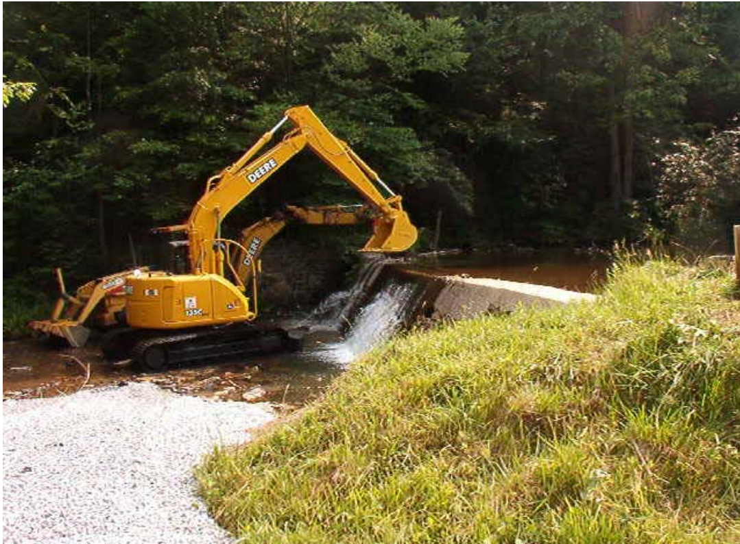
Photo 1. Bens Creek dam removal. Summer 2005.
