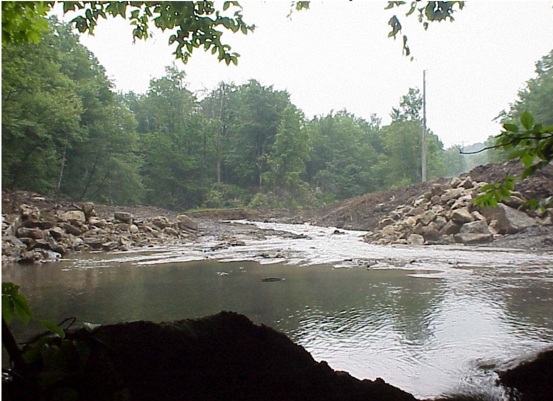
Photo 4. Bens Creek dam site following dam & coffer dam removal. Summer 2005.
