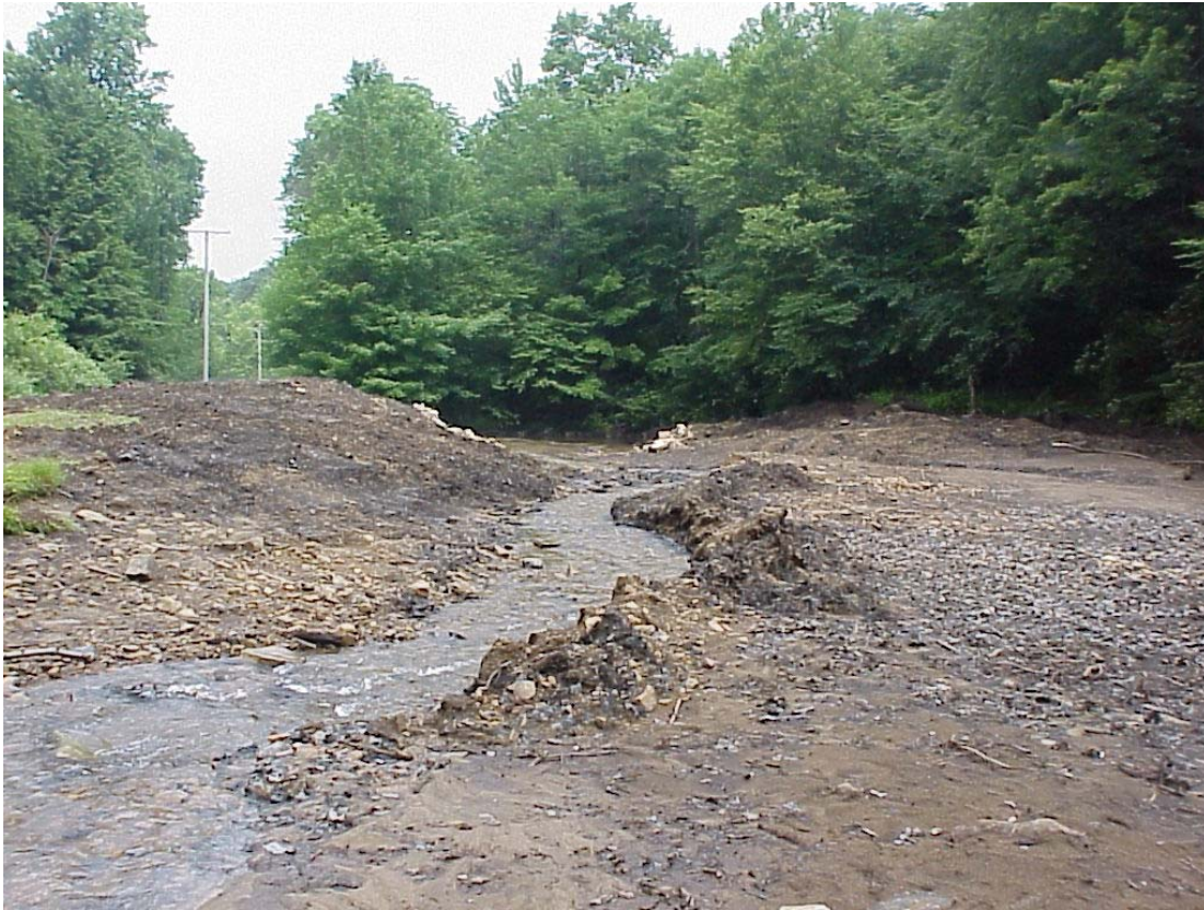
Photo 3. Bens Creek former impoundment immediately following removal. Summer 2005.
