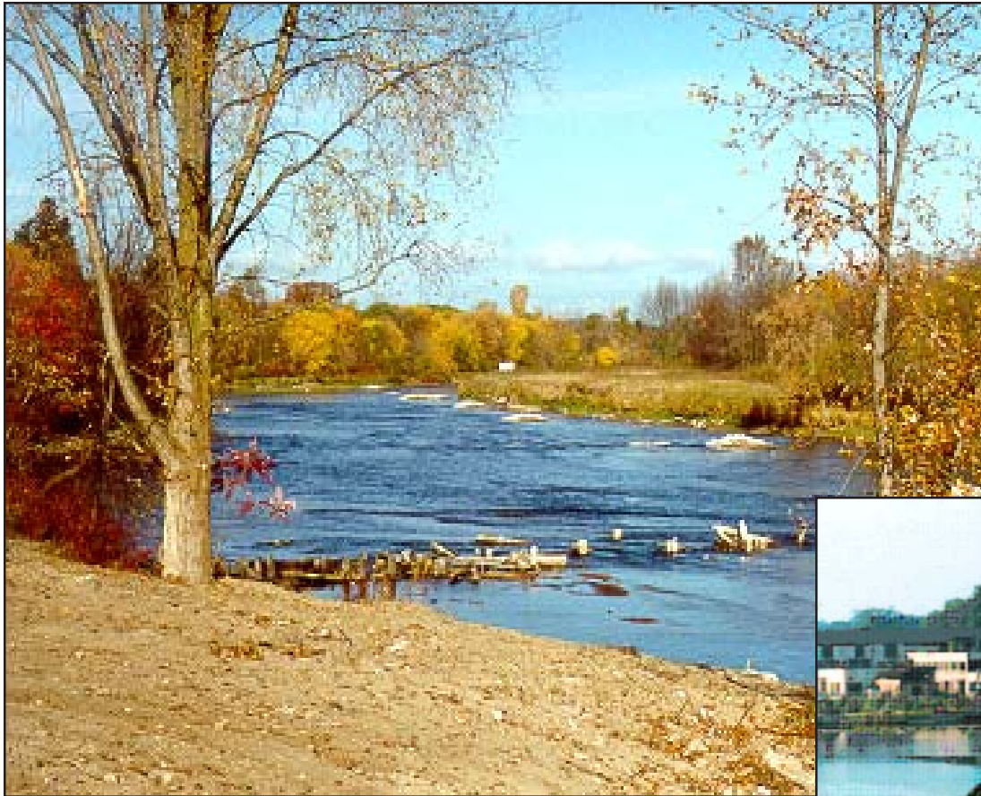
A railroad trestle once crossed the Muskegon river immediately above the dam. Here you can see the timber pilings from the trestle emerging from the water. These piles were removed by the contractor.
