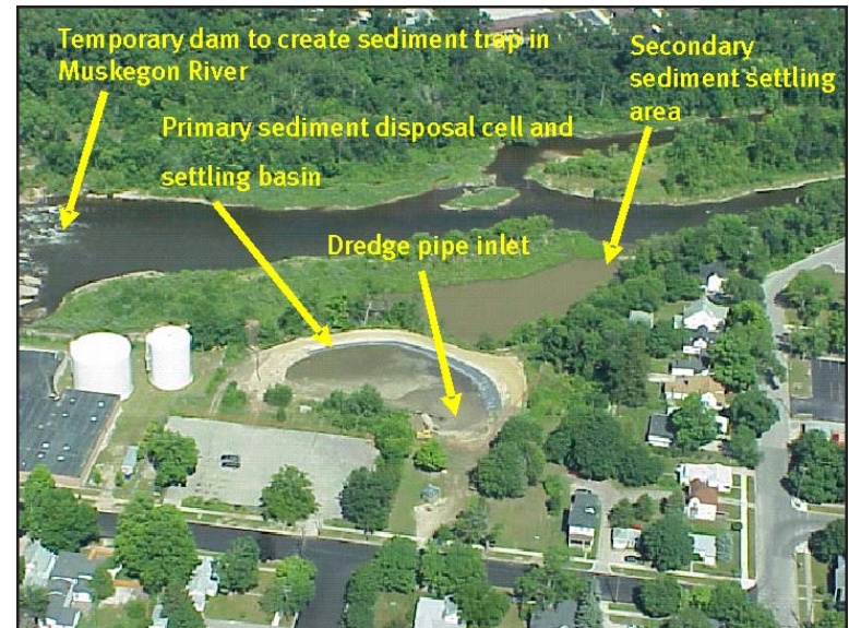
Aerial view of the sediment disposal process.
