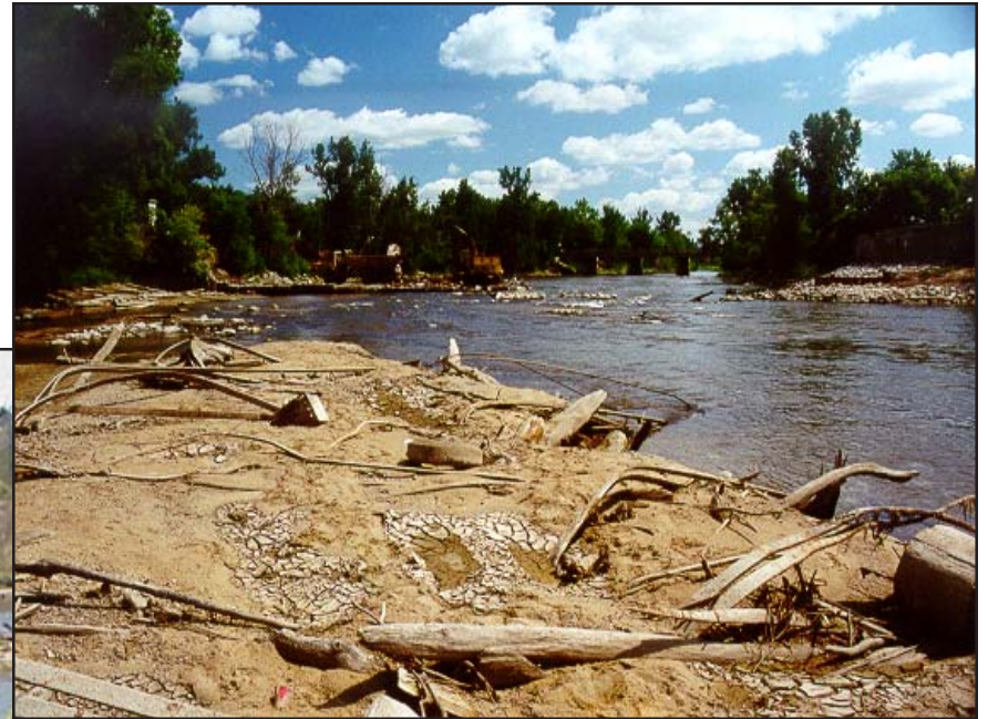
Once the dam's impoundment was drawn down over four feet, many interesting relics became exposed. Just above the dam, the remains of the former steel superstructure for a railroad bridge was found embedded in sediment. The contractor removed the steel and disposed of it.
