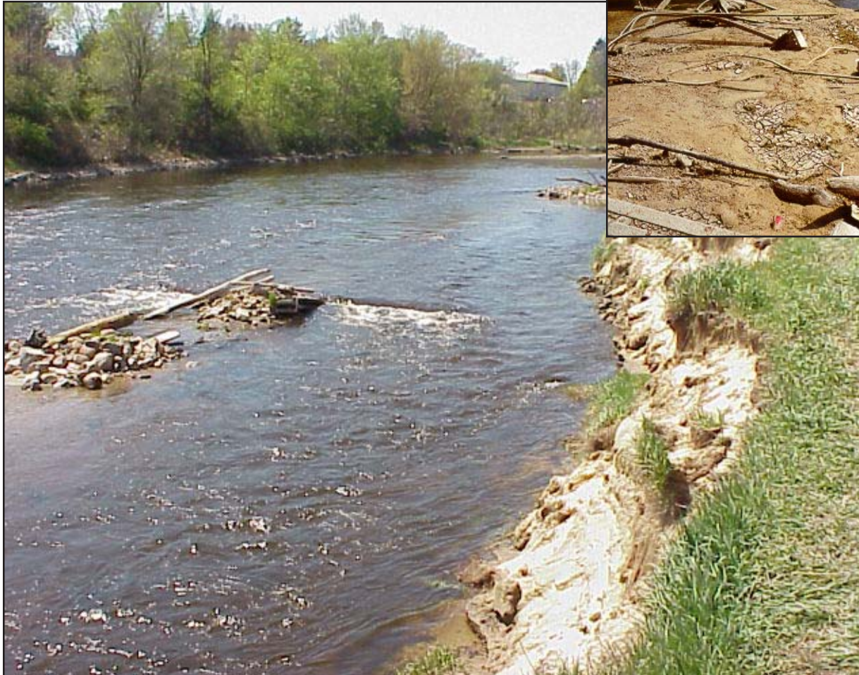
In the 1800s, loggers used timber and rock cribs to corral logs in the river. This formerly inundated old timber and rock crib caused the river's flow to erode a nearby bank.
