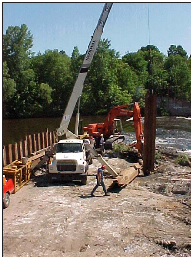
The demolition process began with the contractor driving steel sheet piling upstream of the dam remnant's west side to divert flow over the east side during the demolition process.
