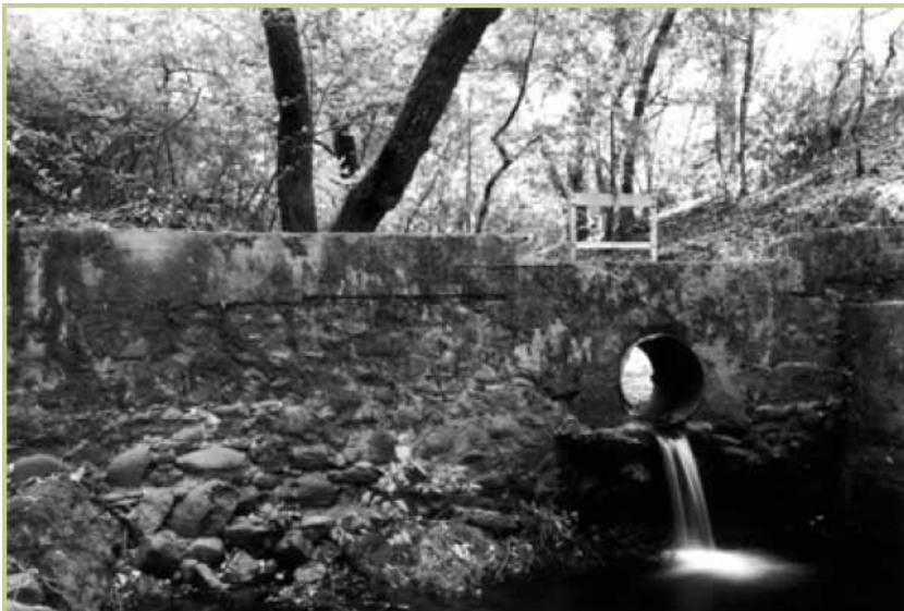
Figure 4-6. Former downstream diversion structure below Upper York Creek dam. (USACE & City of St. Helena, 2007b)
