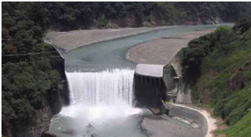
Figure I-8. Bar-lin Dam on the Dahan River in Taiwan, full of sediment in 2006 four years after completion (left), and post-failure in 2007 (right). (Kondolf, 2006 & 2007)
