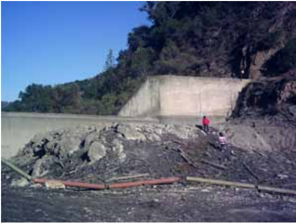
Figure 5-6. Los Padres Dam, upstream of San Clemente, is also filling with sediment and blocks steelhead passage.
