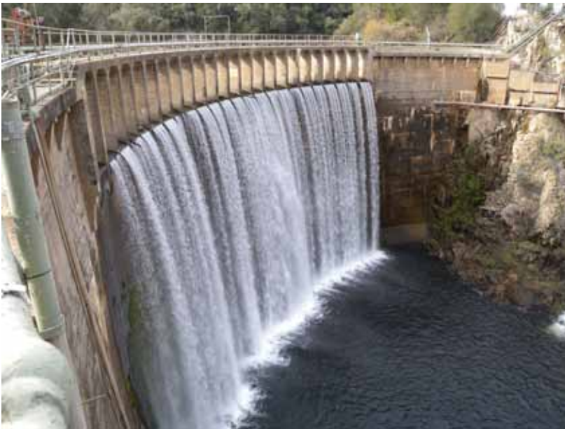
Figure 4-19. San Clemente Dam.
