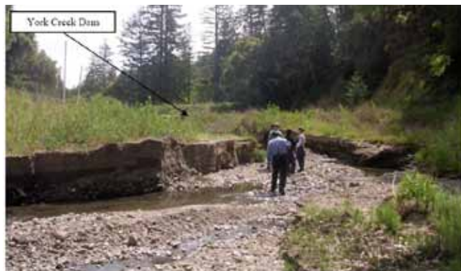
Figure 4-1. Photo of Upper York Creek dam and infilled reservoir. (J. Pollak, 4/8/08)
