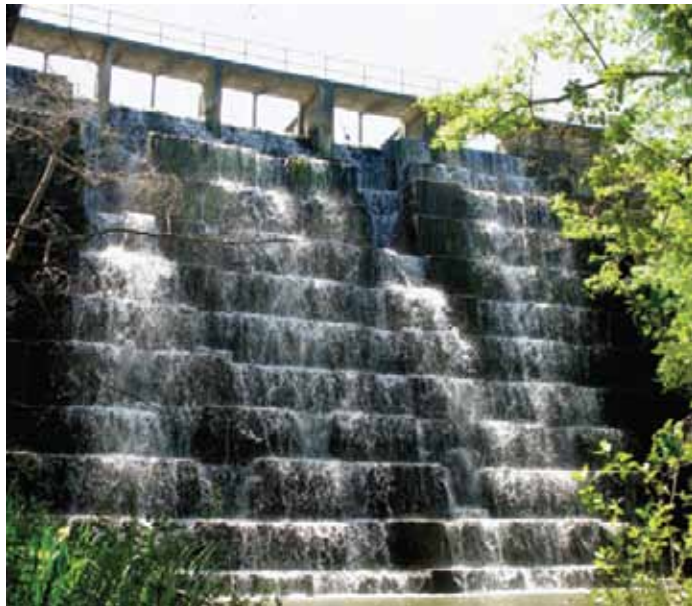
Figure 4-9. Searsville Dam from below. (Stanford University Land Use & Environmental Planning Office, 2009)
