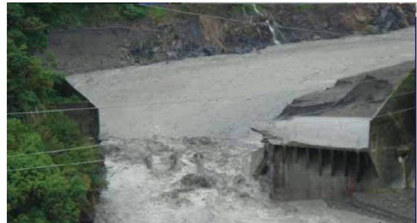
Figure I-8. Bar-lin Dam on the Dahan River in Taiwan, full of sediment in 2006 four years after completion (left), and post-failure in 2007 (right). (Kondolf, 2006 & 2007)
