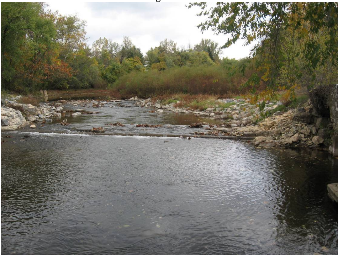
Photo 8. Wolf Lake dam site and impoundment. September 2006.
