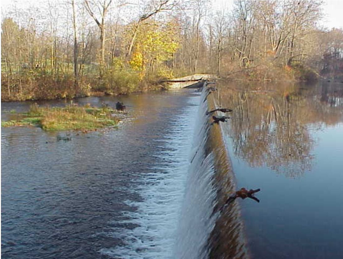
Photo 1. Siloam dam (28-010). Fall 2004.
