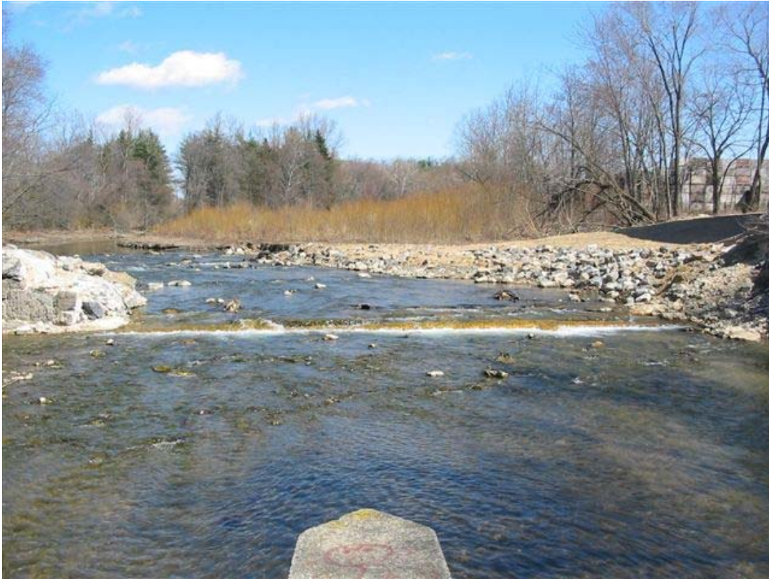
Photo 7. Wolf Lake dam site following removal. March 2006.
