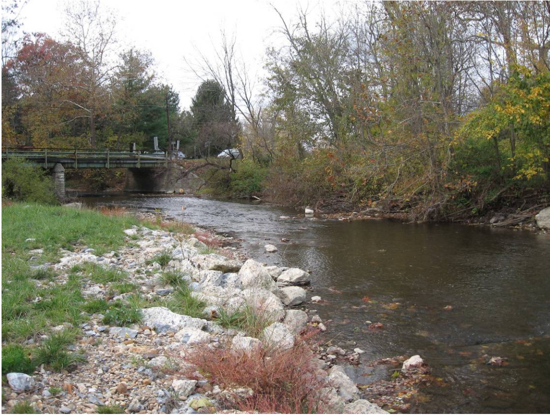
Photo 3. Former Siloam dam site. October 2006.
