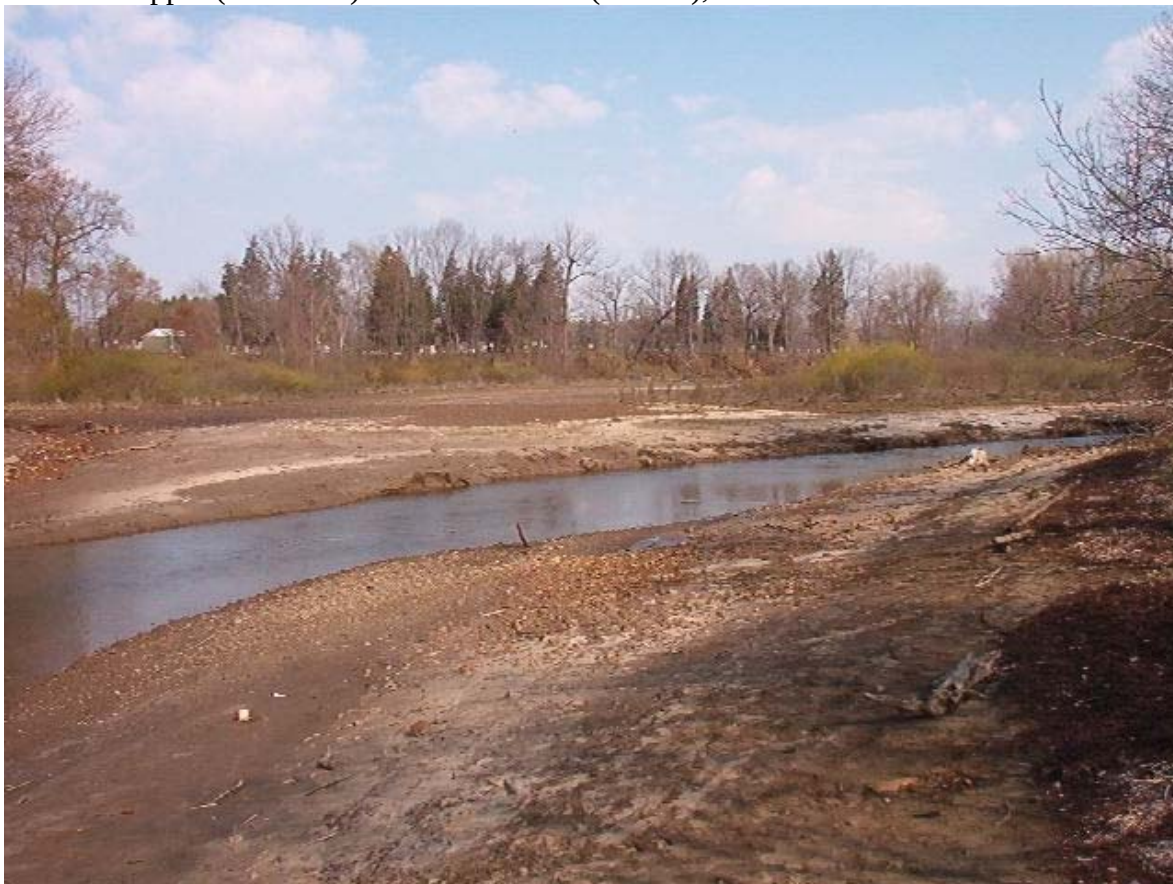
Photo 6. Upper Wolf Creek dam impoundment, immediately following removal. Fall 2004.
