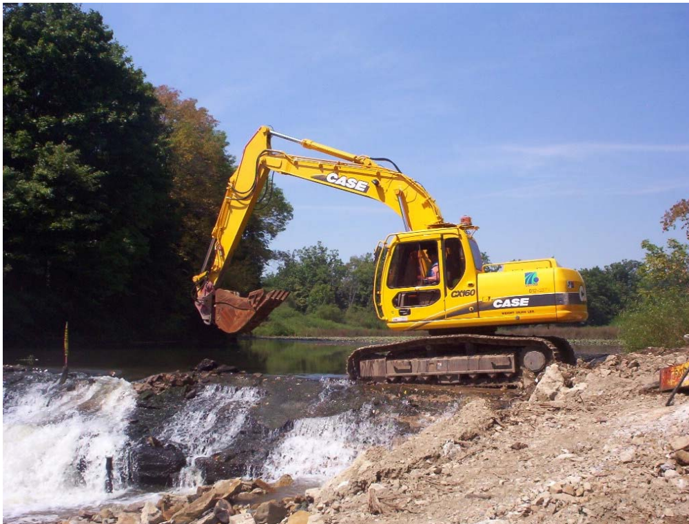
Photo 5. Upper (Unnamed) Wolf Creek dam (43-009), fall 2004.
