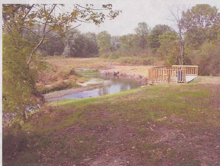
Overview of Observation Deck and Rootwads in Background
