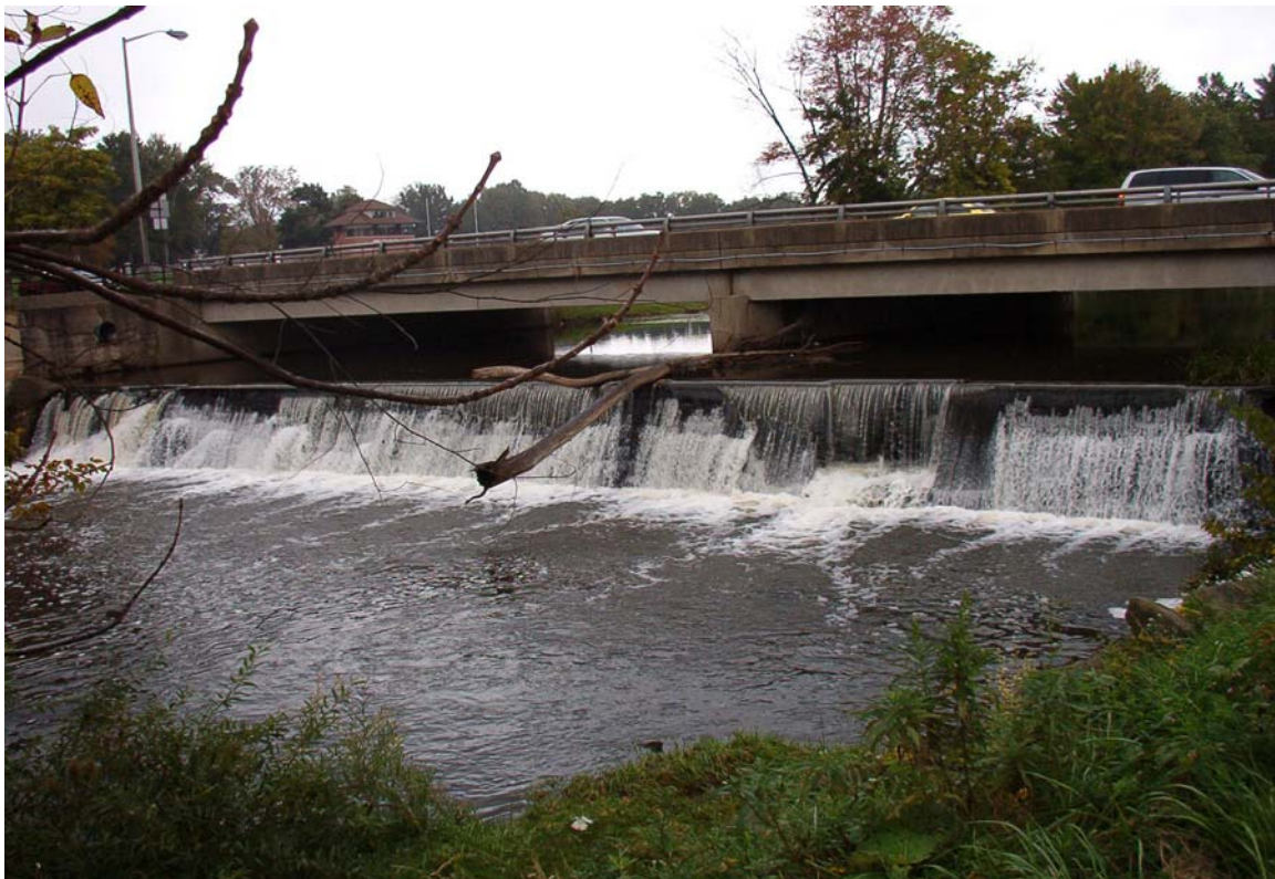
Photo 1. Cunningham Memorial dam (43-005), 2004.
