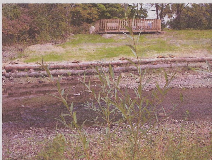
Below Observation Deck After Installation of a Cribwall, Note Willow Live Stake in Foreground
