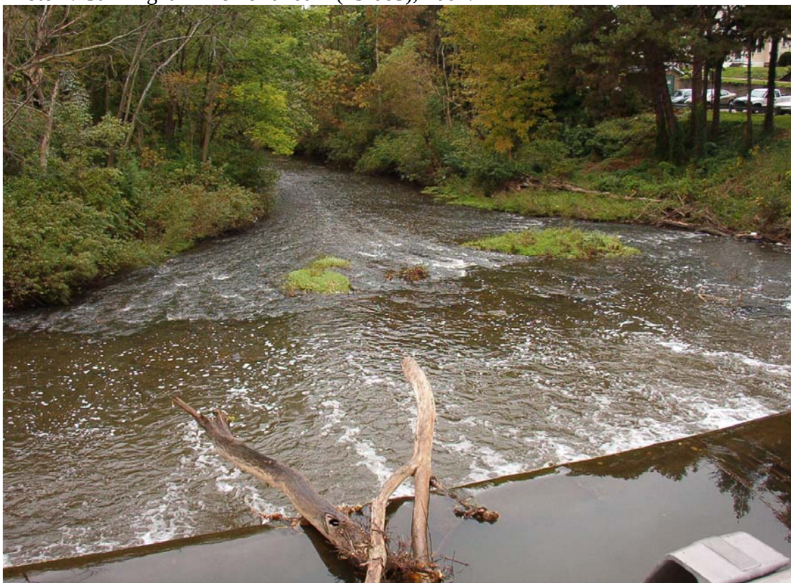
Photo 2. Looking over the crest of Cunningham Memorial dam. 2004.
