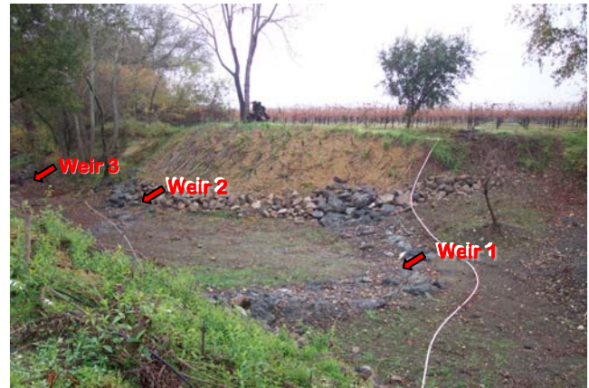
Post-construction: Banks were laid back and stabilized with willow brush mattress and toe rock. Three boulder weirs were installed to allow for easier fish passage and to stabilize the grade of the channel. (Dec. 2007)
