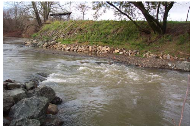
Site observed after flows subsided. No major erosion noted and flows were being directed toward the center of the channel and a pool created. (January 8, 2008)
