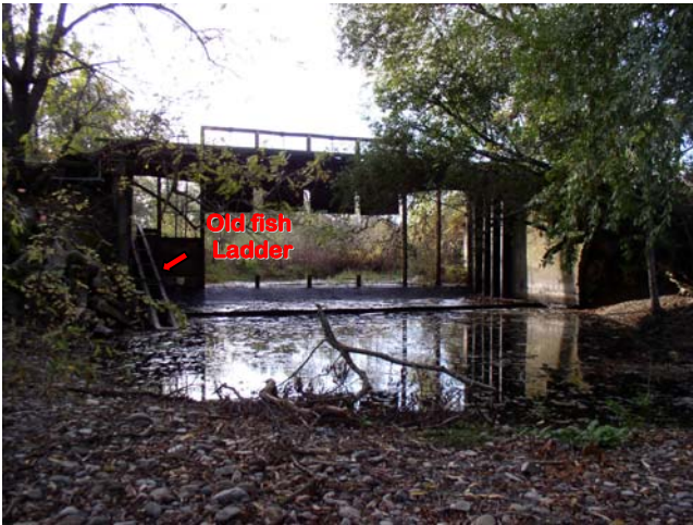
Pre-construction: Facing upstream at barrier, towards concrete sill and apron of the structure which were all removed in addition to the fish ladder on left. (July 2007)
