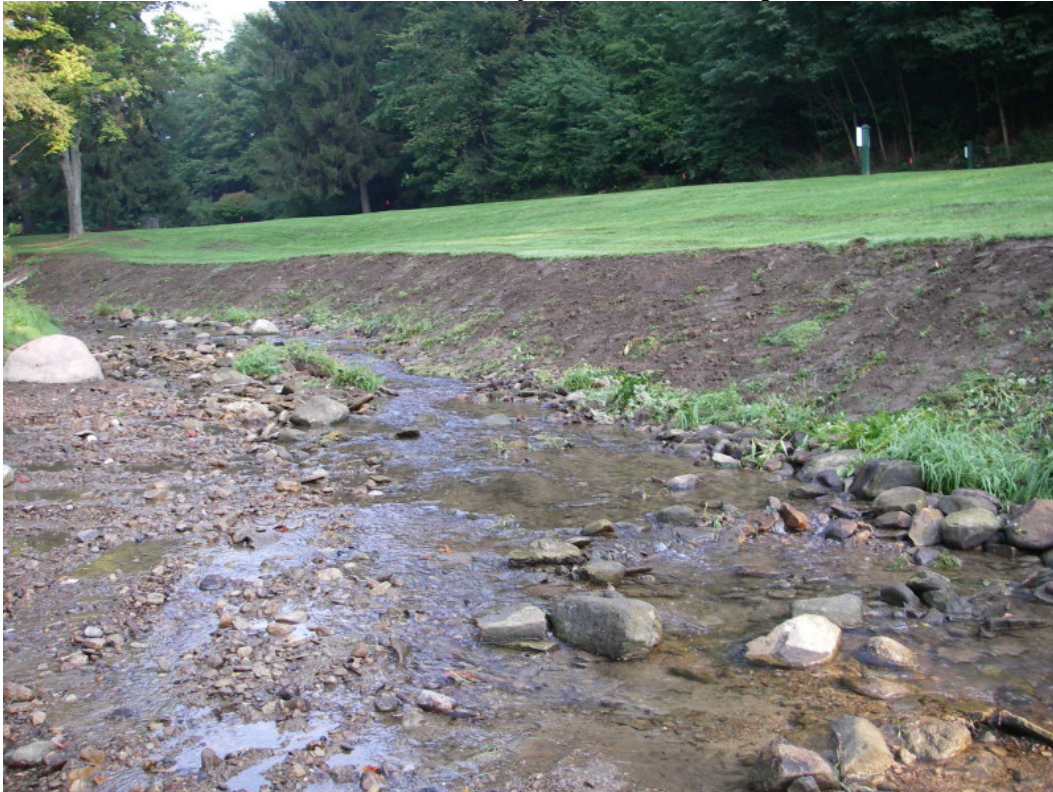
Photo 4. Graceland dam impoundment immediately after removal. September 2006.
