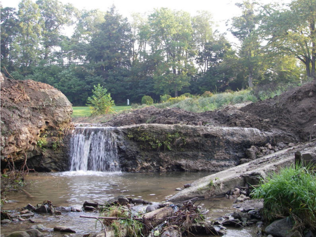
Photo 1. Graceland dam (37-026) prior to removal, summer 2006.
