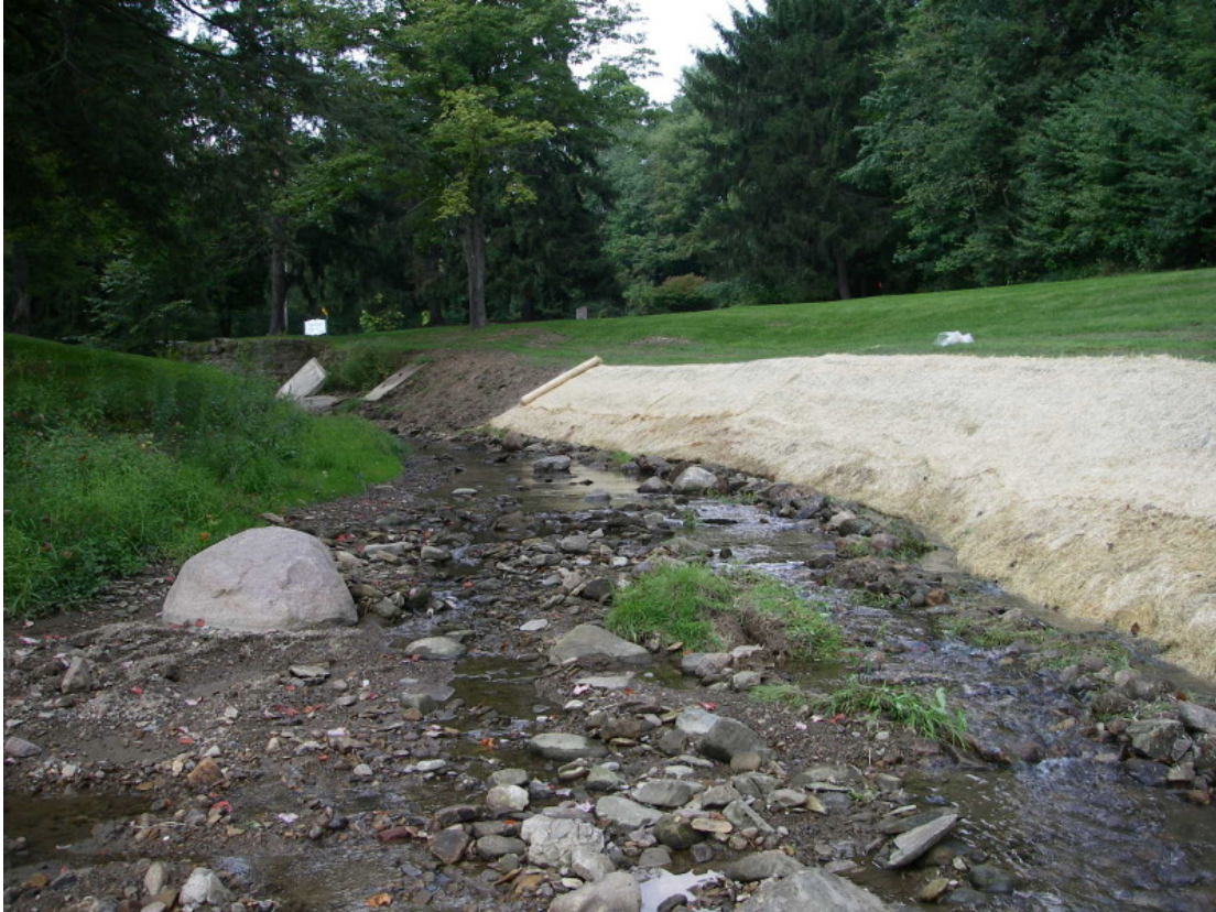
Photo 3. Graceland dam site immediately after removal. September 2006.
