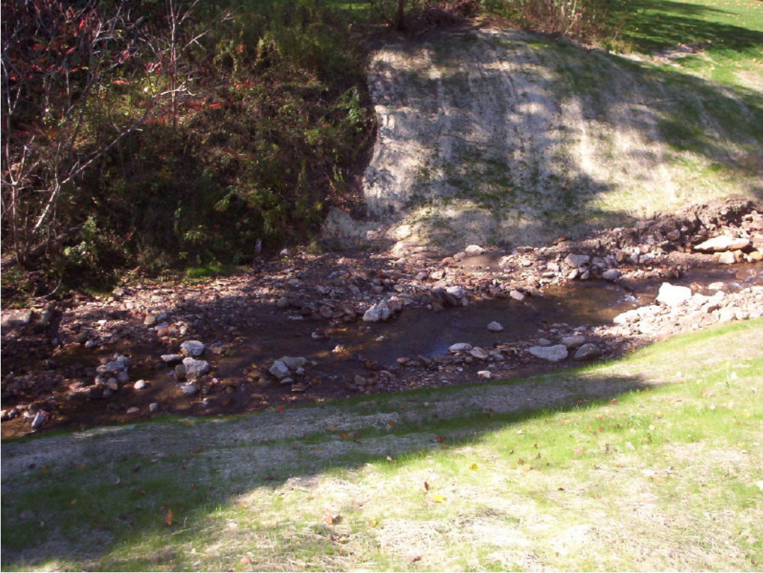
Photo 5. Graceland dam site one month after removal. October 2006.
