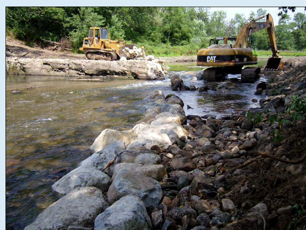
Installing lower weir on river left - 7/17/08
