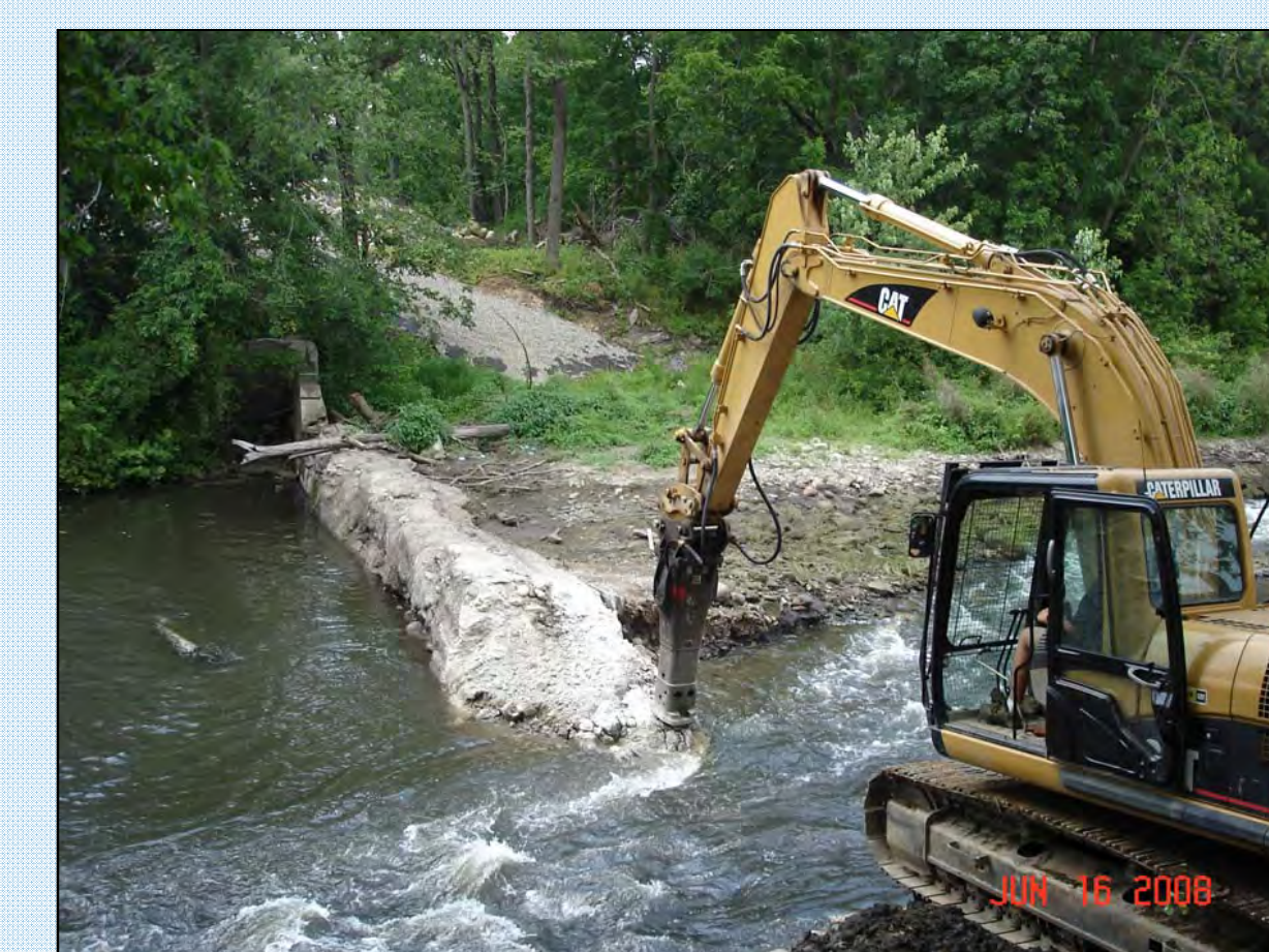
Removing river left half of dam to lower water levels and begin weir installation - 6/16/08
