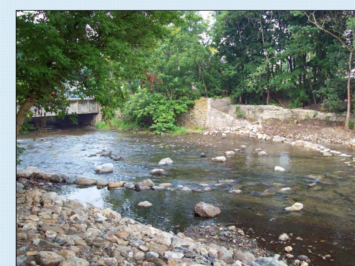
Completed lower weir - 8/6/08
