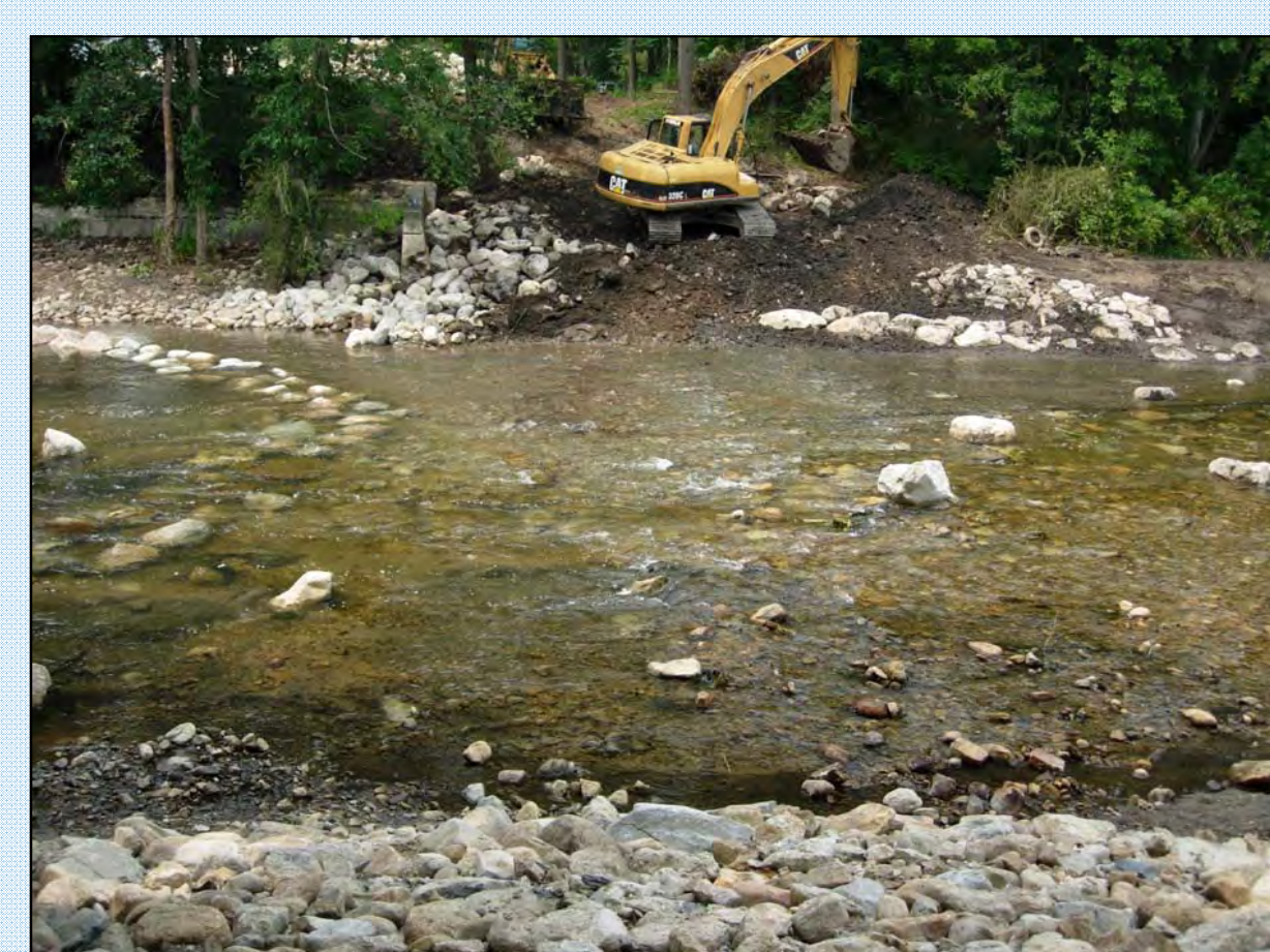
Installing upper weir on river right - 7/30/08
