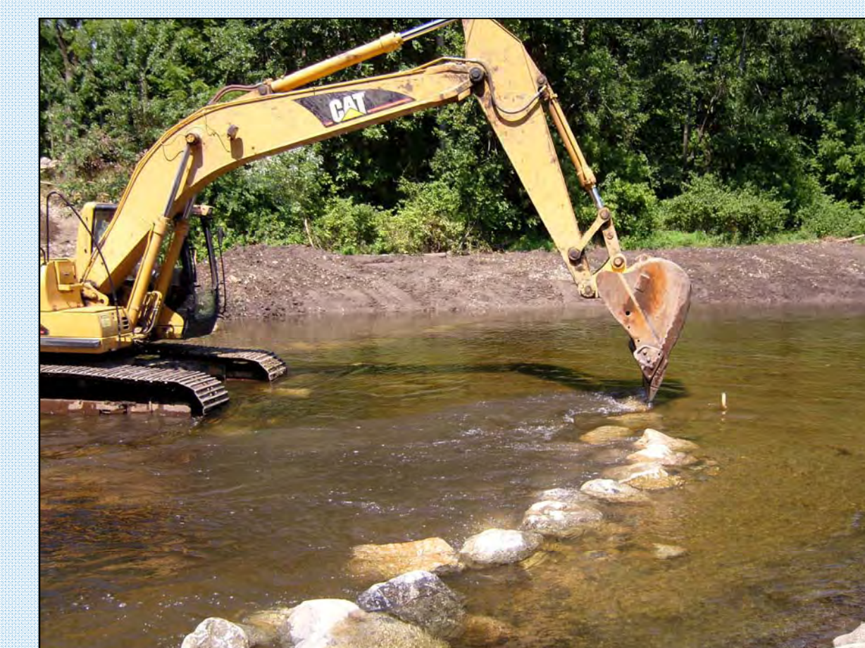
Modifying upper weir on river left - 7/25/08
