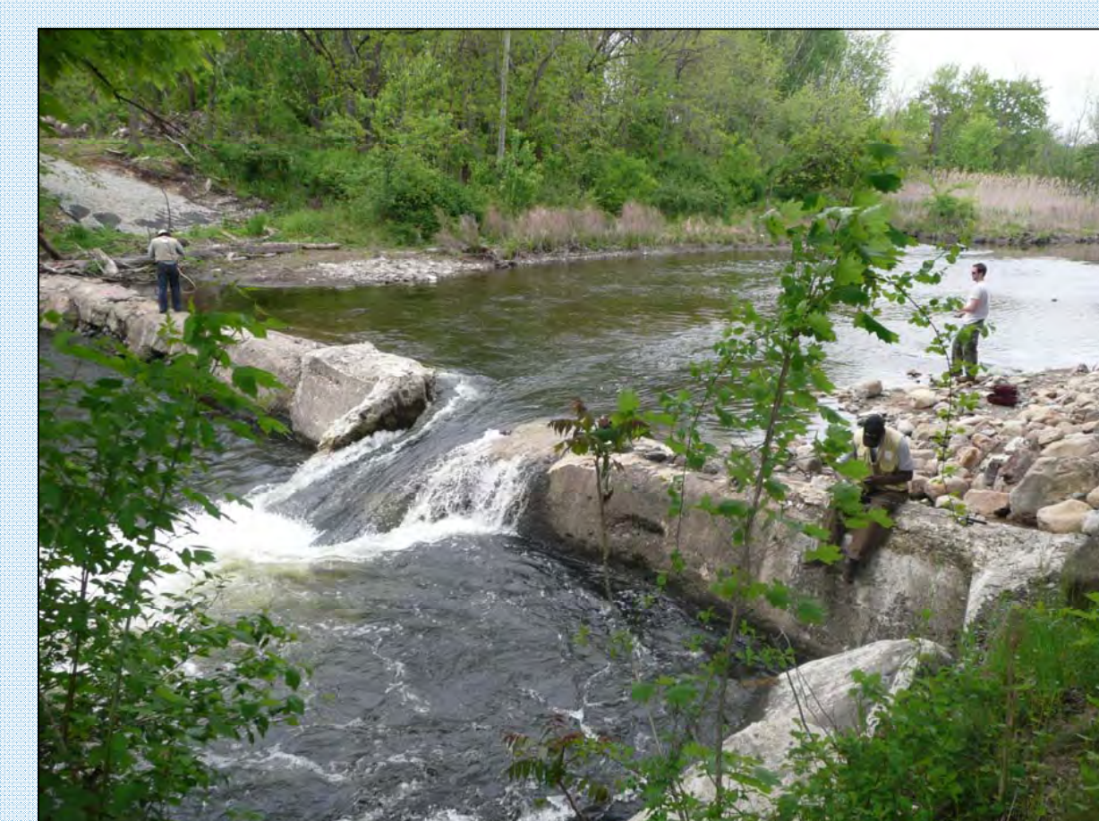
Dewatering the impoundment - 5/14/08
