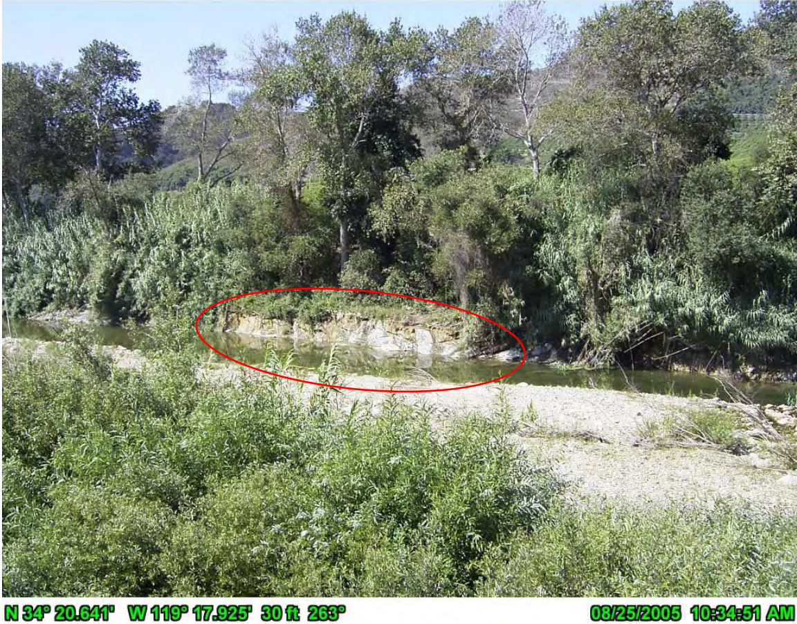
Figure 11.15. Exposed Bedrock along West side of Ventura River near OVSD Facility at RM 5.
