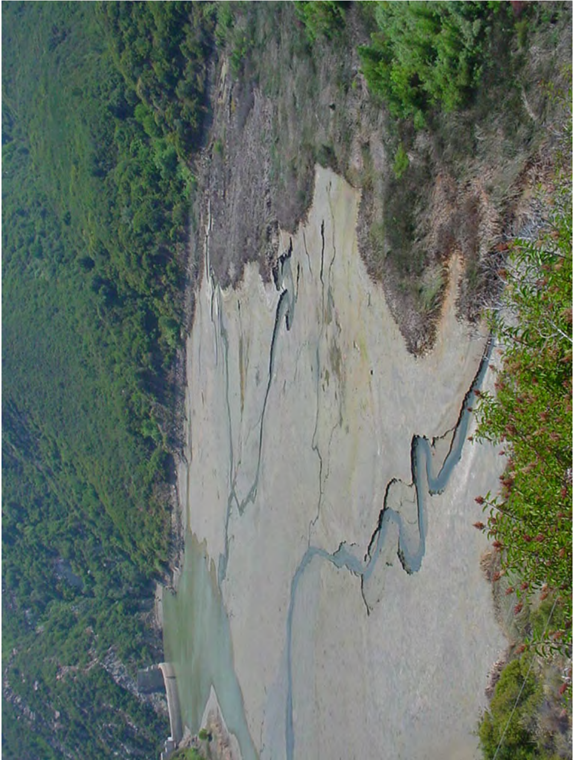
Figure 5.11. Picture of Sediment Trapped behind Matilija Dam While the Reservoir was Drawn Down. Picture was taken in July 2003 by Paul Jenkin of the Surfrider Foundation.
