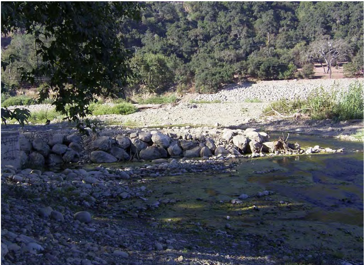
Figure 4.20. Groins installed after 2005 flood along east side of river at Foster Park.
