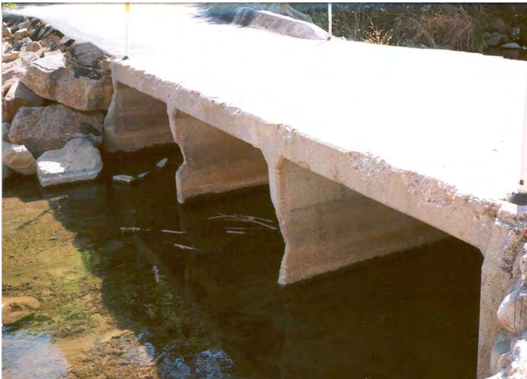
Figure 4.6. Downstream side of Camino Cielo.
