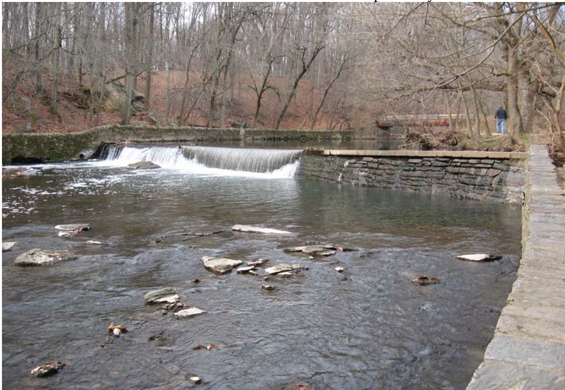
Photo 6. Roosevelt Blvd dam in December 2006.
