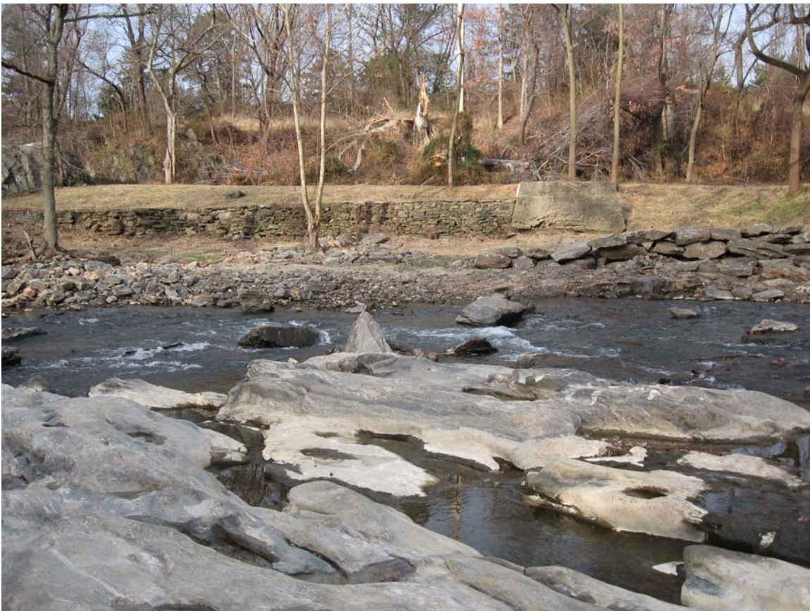
Photo 4. Frankford Ave. dam site immediately following removal. December 2006.
