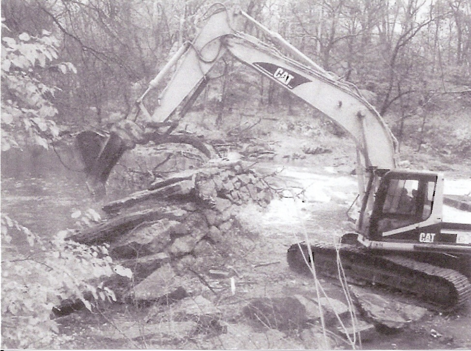
Photo 3. Frankford Ave. dam during removal. December 2006.
