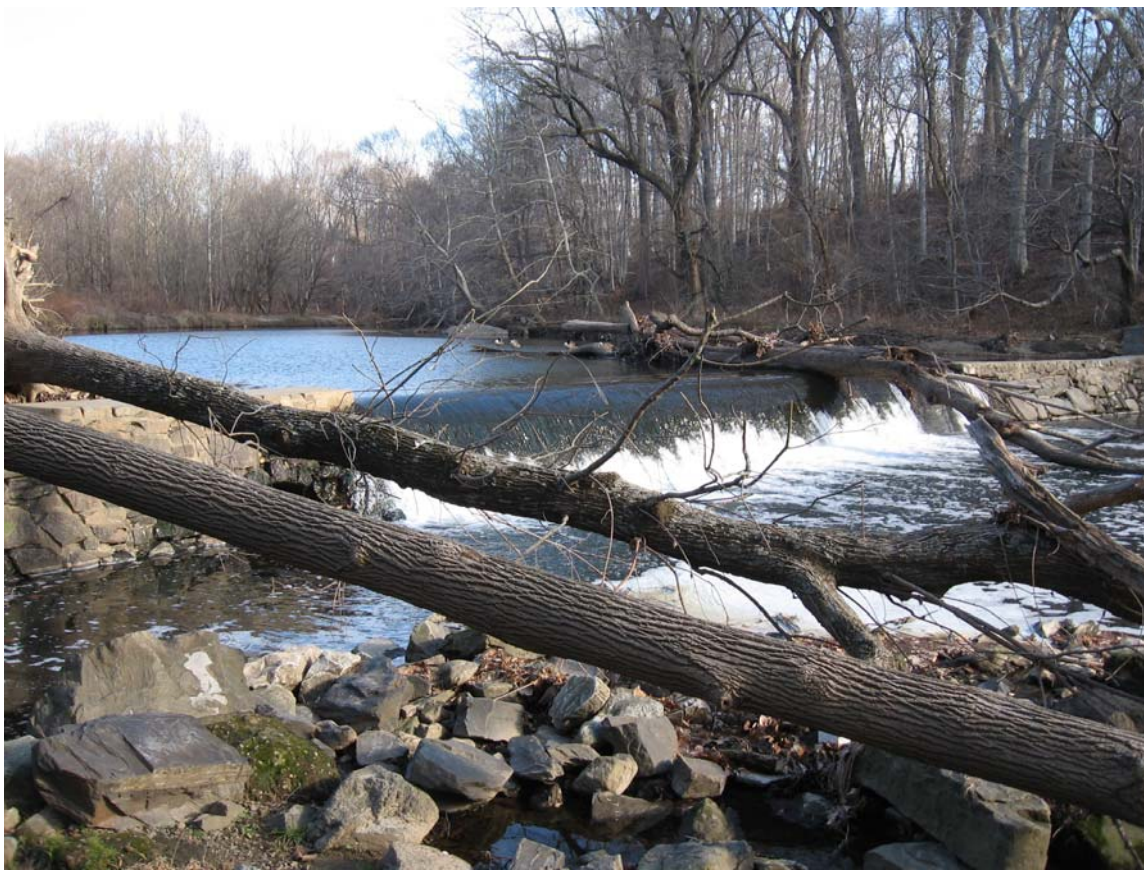
Photo 7. Verree Rd. dam in December 2006.
