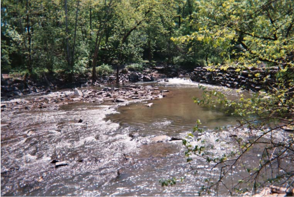
Photo 1. Rhawn St. dam before removal. Summer 2004.
