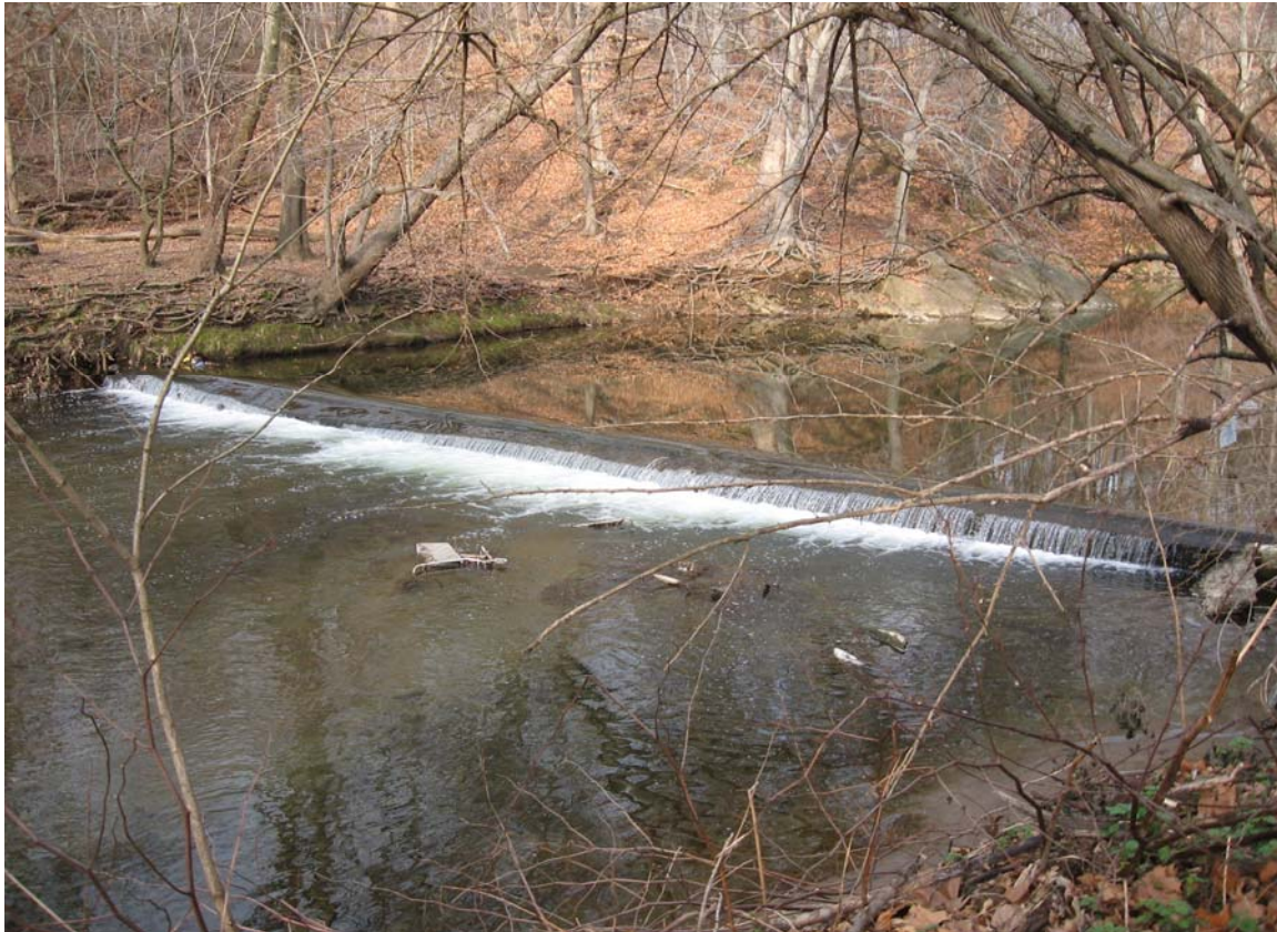
Photo 5. PWD Sewer Line 1 in December 2006. Rock ramp fishway to be built in 2007.
