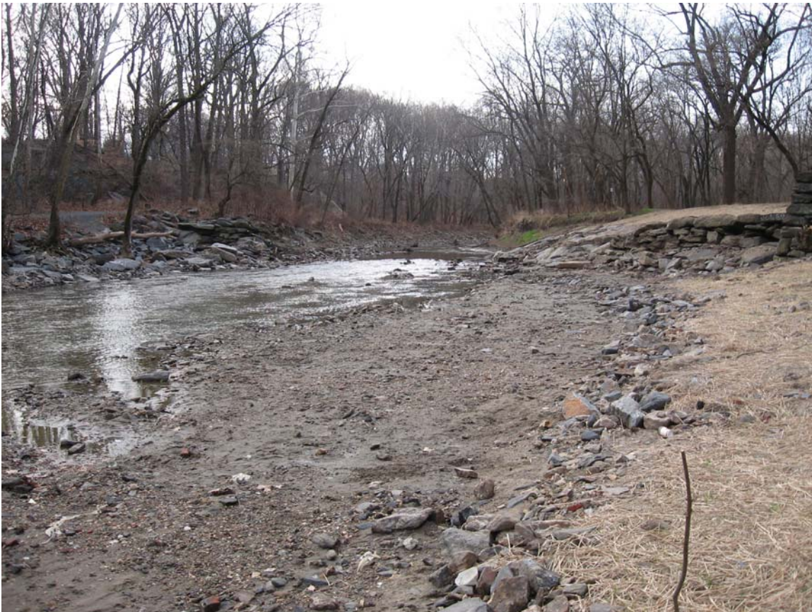
Photo 2. Rhawn St. dam site immediately following removal. December 2006.
