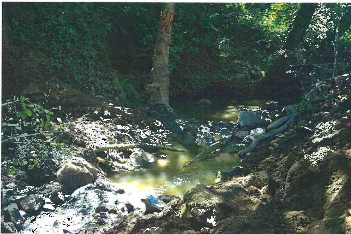
Photo 5: This post-dam removal shot shows an alder tree on the left bank that was scarred during construction.
