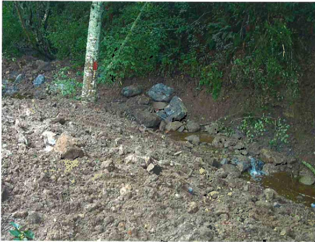
Photo 3: Taken on September 22, 2000, this photo shows the disturbed condition of the site immediately following the dam removal.
