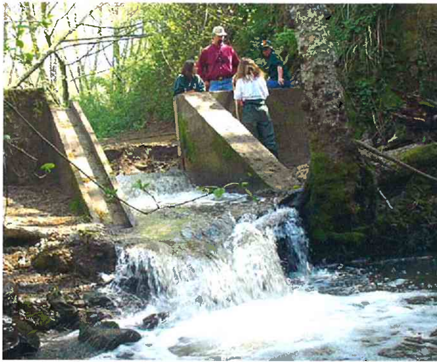
Photo 1: The dam as it appeared on March 17, 2000. After the 1997 construction was halted, all but one flashboard were removed from the dam.
