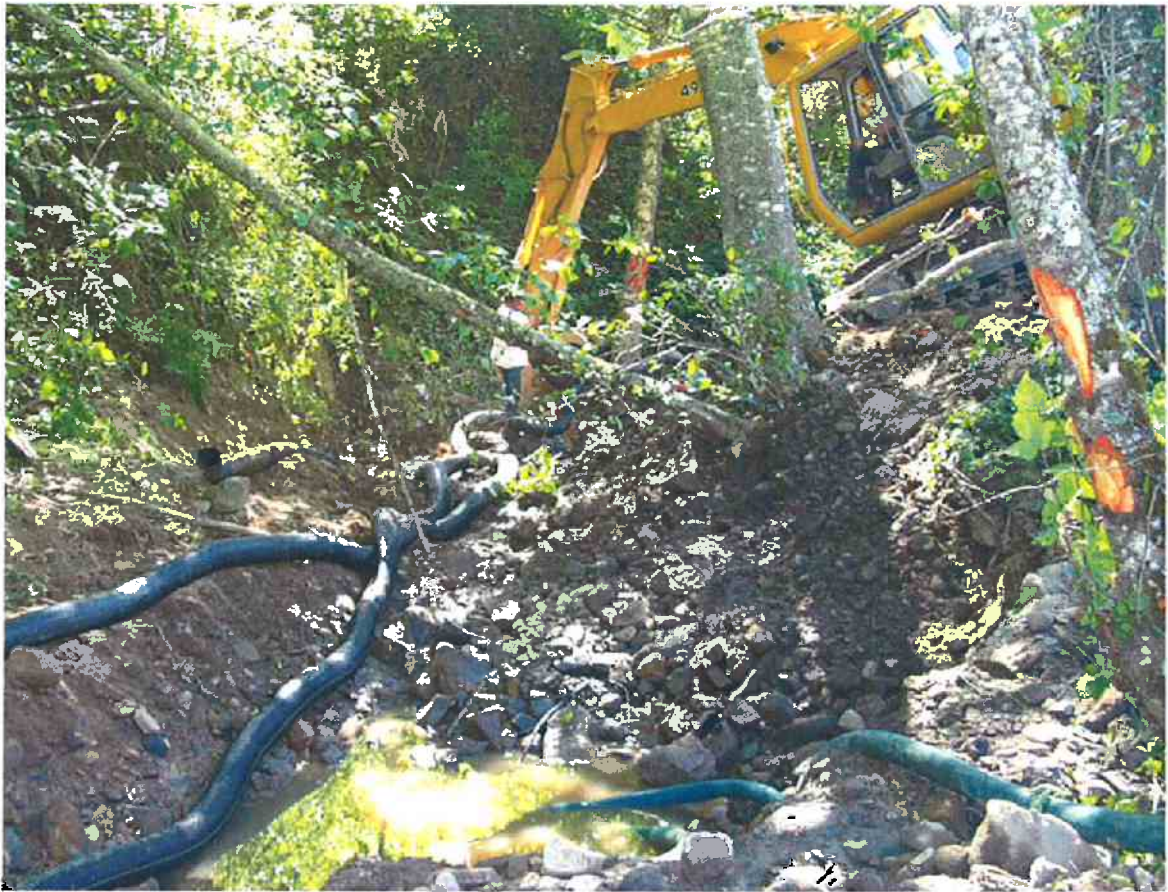
Photo 7: During the 2000 construction phase, the river was diverted through pipes. Excavation was used to establish a pool-riffle sequence.
