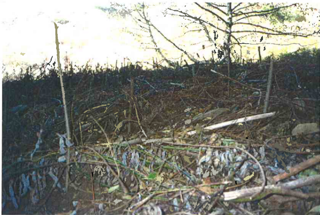
Photo 4: Efforts towards bank stabilization and revegetation had improved by the November 20, 2000 site visit. Cuttings from local vegetation had been strewn on the banks and willow poles had been planted.
