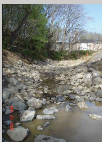
Finished channel looking upstream.
