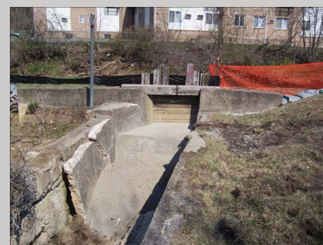
Plugging mill raceway with concrete.
