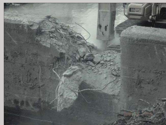
Demolition of spillway portion to be removed with hydraulic hammer.
