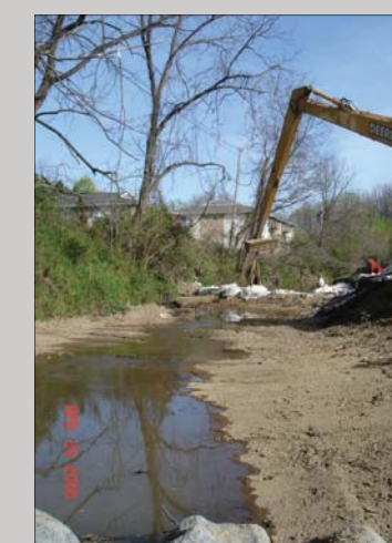
Releasing the Lopatcong to the finished channel and breach.
