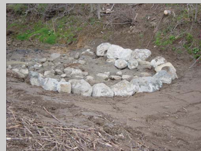
Installed rock vane (1 of 4).
