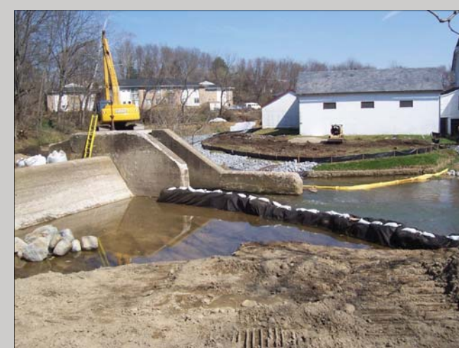
Setting up downstream cofferdam.
