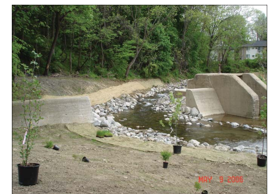
The Completed Fish Passage And Preserved Spillway
