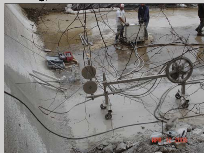
Diamond wire sawing of concrete spillway.
