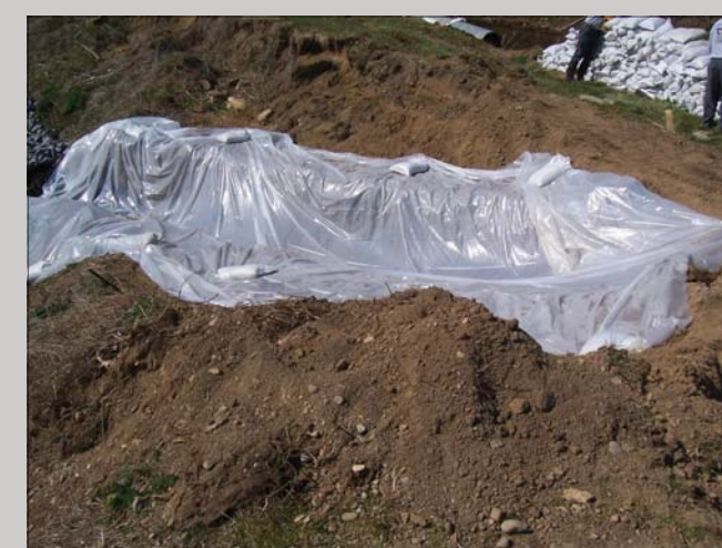
Excavation and lining of diversion channel at upstream end of project.
