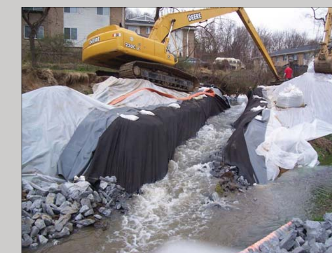
Diverting the Lopatcong Creek.
