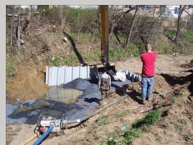
Installing sheetpile at upstream end to eliminate headcutting.
