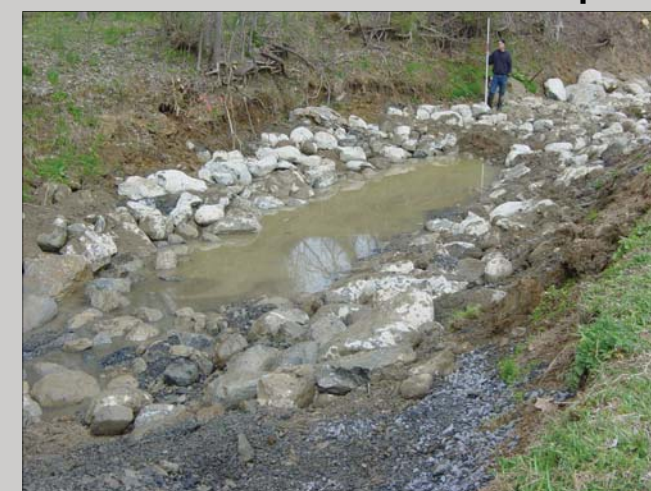
Installed deep pool.
