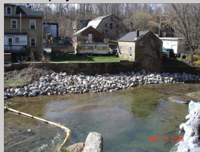
Armoring historic walls downstream of project with river stone
