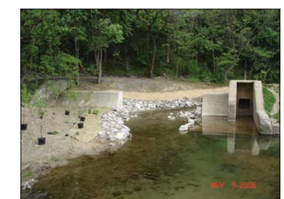
The Completed Fish Passage And Preserved Spillway
