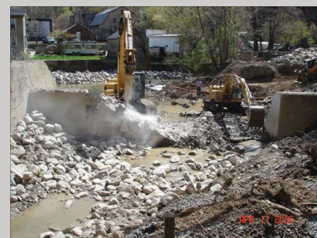
Continued demolition of spillway.
