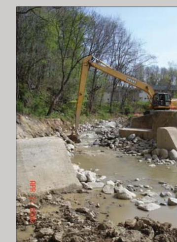
The final touches on the stream channel.
