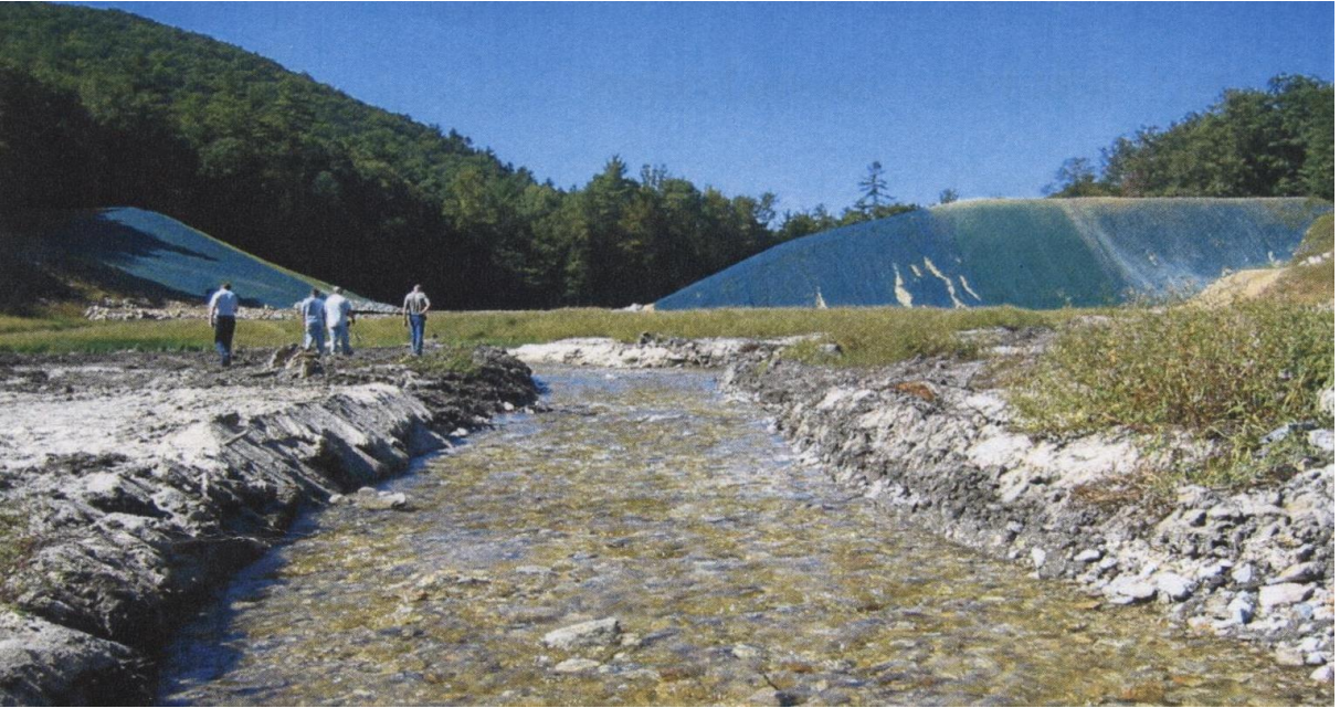
Figure 4. Image of the re-constructed Conococheague Creek channel after activation (DEP file photo dated, 1.February.2006). This image was used as photographic evidence of as-built conditions in order to submit a “Dam Breach Completion Certification” to DEP.
