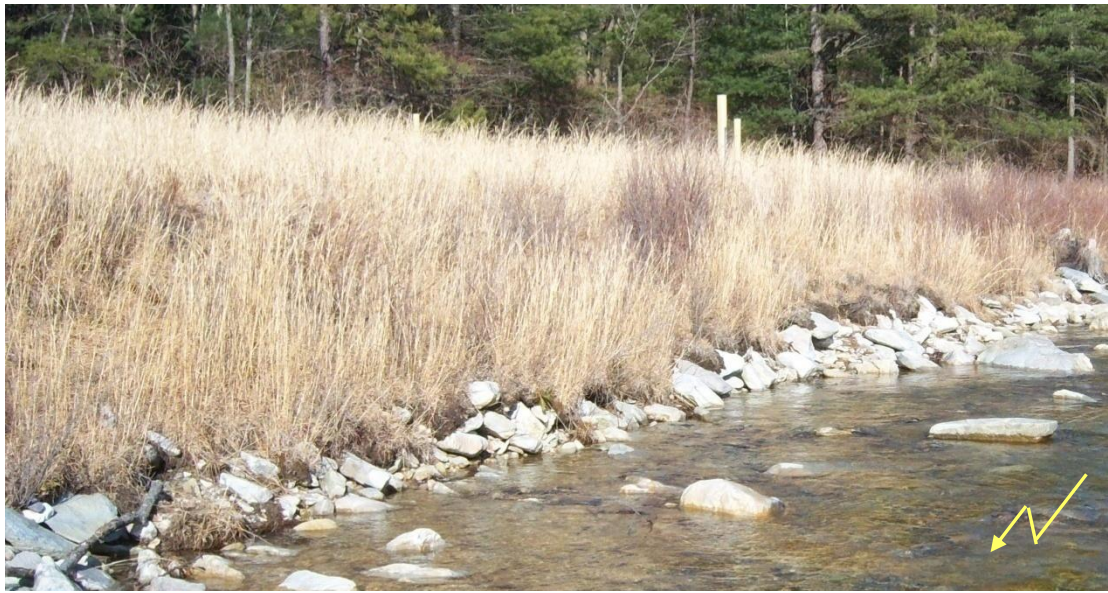
Figure 14. Image of the cobble-sized armoring along the right bank of the Bravo channel. Grasses are dominant cover along the majority of the bank (author's image dated, 05.March.2009).
