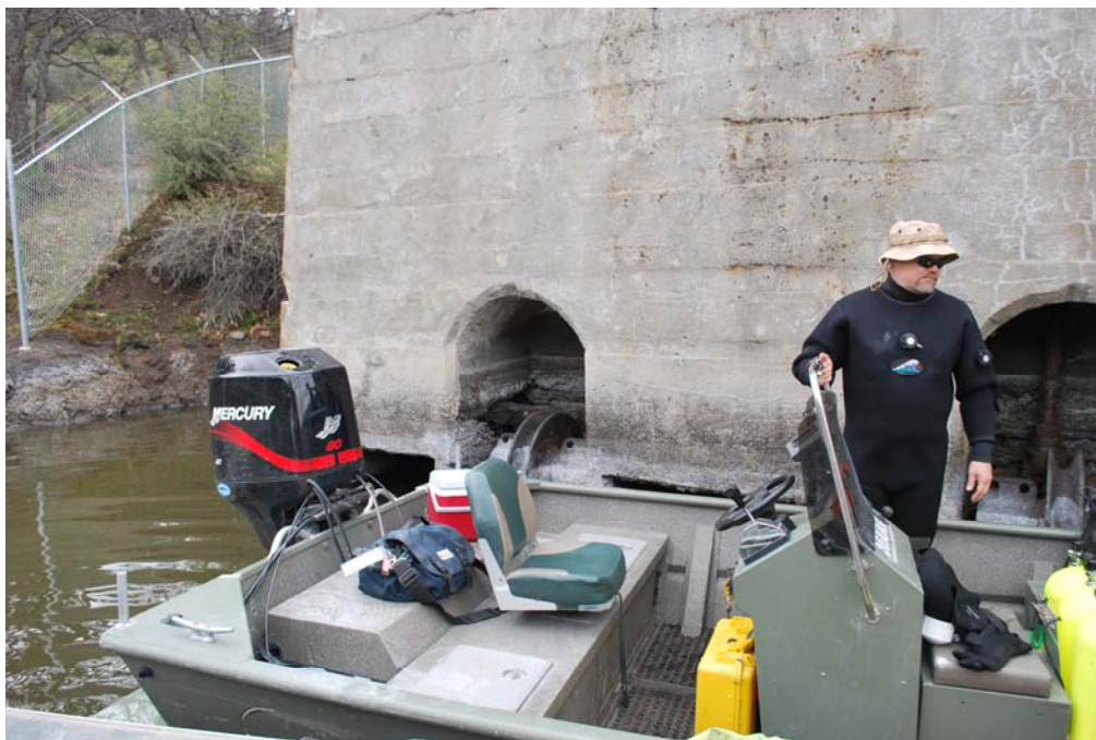
Photograph No. 14 Dive boat secured at right abutment near abandoned low level intake control structure at Copco 1 Dam. Bureau of Reclamation - Pacific Northwest Underwater Inspection Team. Copco 1 Dam, Klamath Hydroelectric Project, Oregon-California – April 12-16, 2010.
