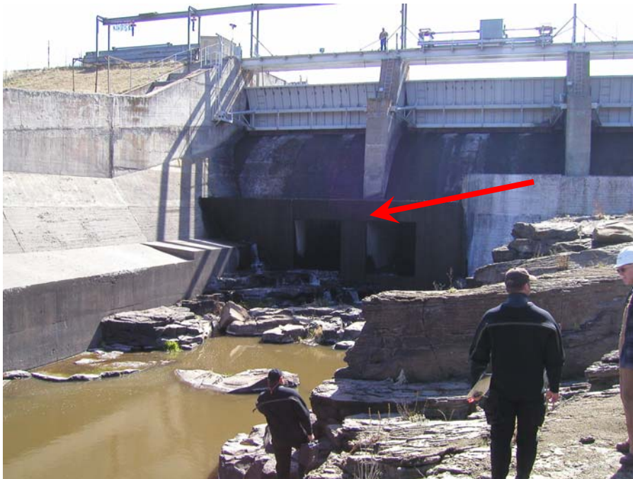
Photograph No. 24 View looking upstream at double barrel diversion conduit (red arrow) used during construction of JC Boyle Dam. Bureau of Reclamation - Pacific Northwest Underwater Inspection Team. JC Boyle Dam, Klamath Hydroelectric Project, Oregon-California – April 12-16, 2010.
