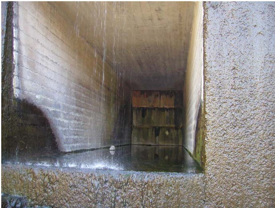
Photograph No. 25 View looking upstream at left double barrel diversion conduit. Bureau of Reclamation - Pacific Northwest Underwater Inspection Team. JC Boyle Dam, Klamath Hydroelectric Project, Oregon-California – April 12-16, 2010.
