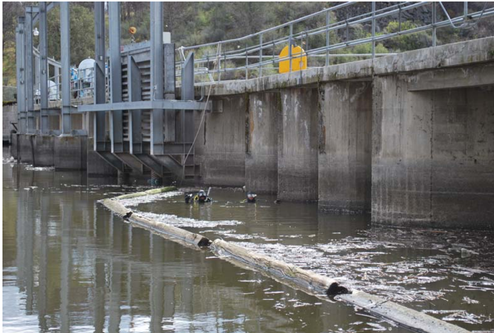
Photograph No. 13 Divers on surface relaying findings of dive inspection of the powerplant intake at Copco 1 Dam. Bureau of Reclamation - Pacific Northwest Underwater Inspection Team. Copco 1 Dam, Klamath Hydroelectric Project, Oregon-California – April 12-16, 2010.
