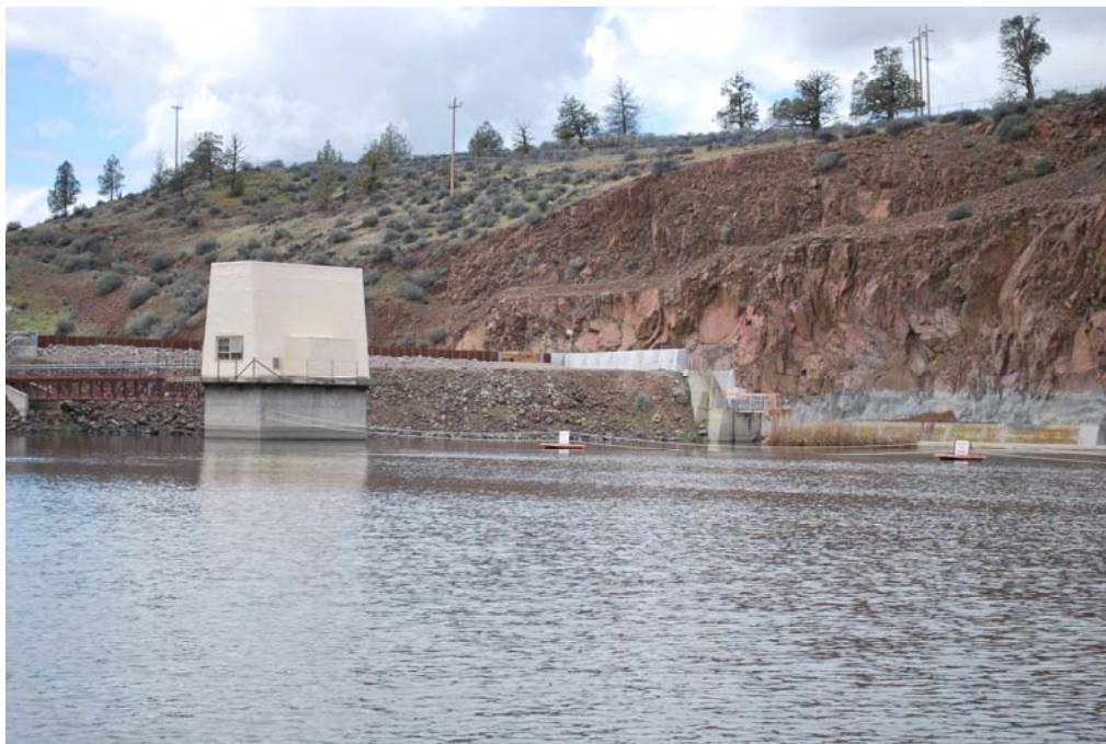
Photograph No. 4 Right abutment of Iron Gate dam at approximate location for deployment of ROV used to survey intake structure. Bureau of Reclamation - Pacific Northwest Underwater Inspection Team. JC Boyle, Copco 1 and Iron Gate Dam, Klamath Hydroelectric Project, Oregon-California – April 12-16, 2010.
