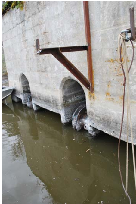
Photograph No. 15 Cable roller device for abandoned low level intake structure at Copco 1 Dam. Bureau of Reclamation - Pacific Northwest Underwater Inspection Team. Copco 1 Dam, Klamath Hydroelectric Project, Oregon-California – April 12-16, 2010.
