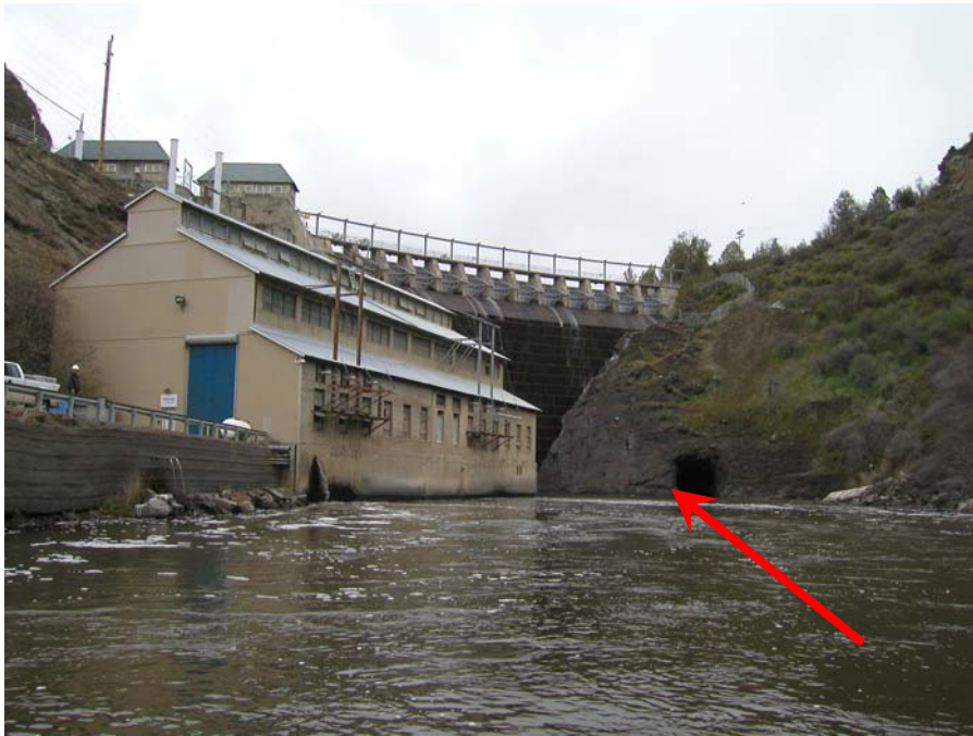
Photograph No. 17 Upstream view of Copco 1 Dam. On left side is powerplant generator structure. On right side (red arrow) shows abandoned low level outlet tunnel. Divers made a boat assisted surface inspection of concrete plug. Bureau of Reclamation - Pacific Northwest Underwater Inspection Team. Copco 1 Dam, Klamath Hydroelectric Project, Oregon-California – April 12-16, 2010.
