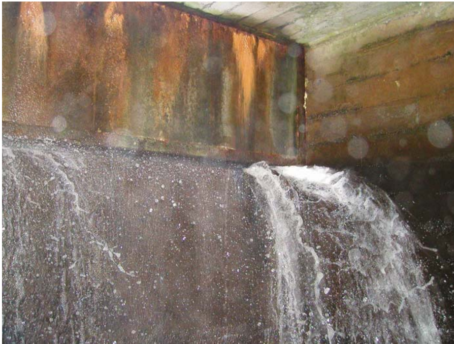
Photograph No. 30 Flow through the stop logs on the right side of the double barrel diversion conduit. Bureau of Reclamation - Pacific Northwest Underwater Inspection Team. JC Boyle Dam, Klamath Hydroelectric Project, Oregon-California – April 12-16, 2010.
