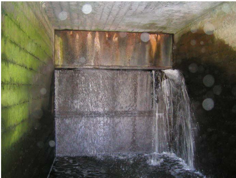
Photograph No. 29 Upstream view on right side of double barrel diversion conduit showing flow through the concrete stop log. P-Delta effects were noted by divers on the upstream side of this structure. Bureau of Reclamation - Pacific Northwest Underwater Inspection Team. JC Boyle Dam, Klamath Hydroelectric Project, Oregon-California – April 12-16, 2010.
