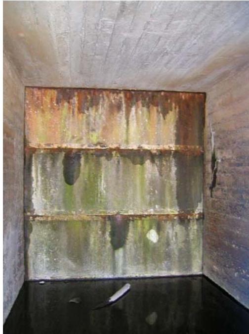
Photograph No. 26 Upstream view of stop logs in the left side of the double barrel diversion conduit. Bureau of Reclamation - Pacific Northwest Underwater Inspection Team. JC Boyle Dam, Klamath Hydroelectric Project, Oregon-California – April 12-16, 2010.
