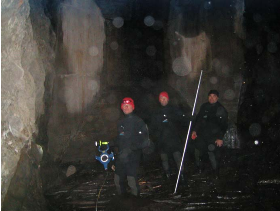
Photograph No. 18 Divers standing at furthest most point accessible next to concrete plug, making field measurements. Bureau of Reclamation - Pacific Northwest Underwater Inspection Team. JC Boyle, Copco 1 and Iron Gate Dam, Klamath Hydroelectric Project, Oregon-California – April 12-16, 2010.
