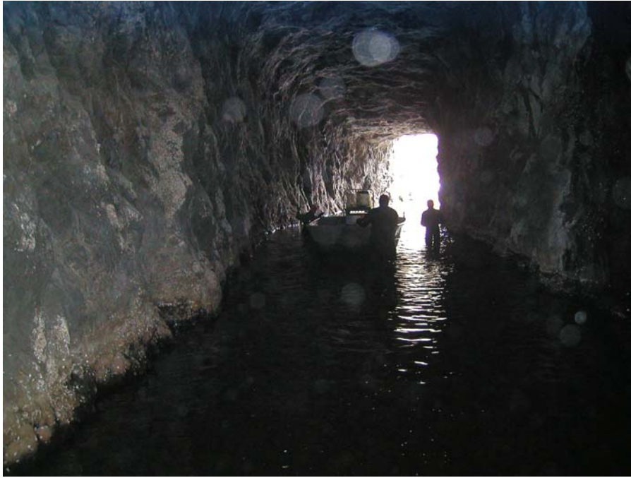
Photograph No. 20 View of low-level outlet tunnel looking downstream to portal. Bureau of Reclamation - Pacific Northwest Underwater Inspection Team. Copco 1 Dam, Klamath Hydroelectric Project, Oregon-California – April 12-16, 2010.
