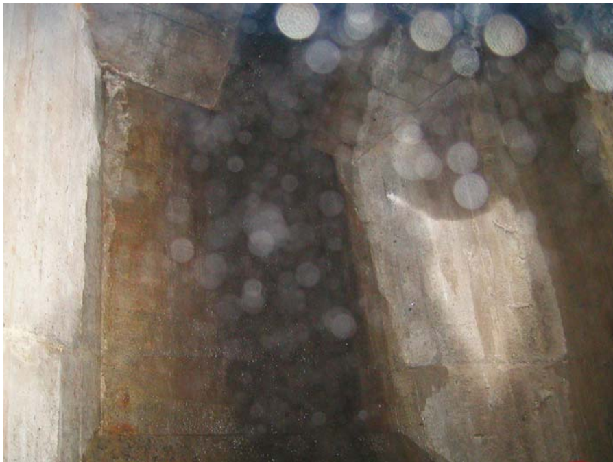
Photograph No. 19 Close-up view of concrete plug in the abandoned low-level outlet tunnel at Copco 1 Dam. Bureau of Reclamation - Pacific Northwest Underwater Inspection Team. Copco 1 Dam, Klamath Hydroelectric Project, Oregon-California – April 12-16, 2010.
