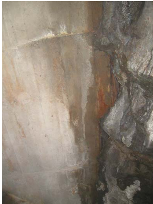
Photograph No. 23 Concrete plug interface with rock tunnel in the abandoned low-level outlet tunnel at Copco 1 Dam. Bureau of Reclamation - Pacific Northwest Underwater Inspection Team. Copco 1 Dam, Klamath Hydroelectric Project, Oregon-California – April 12-16, 2010.
