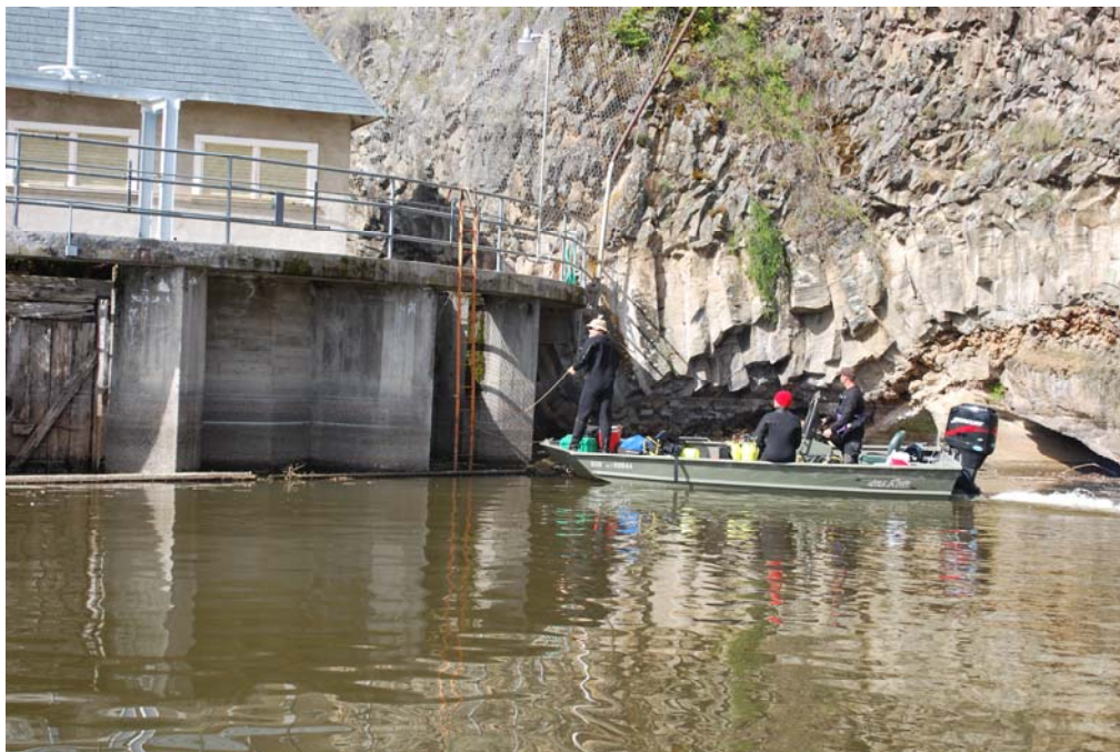
Photograph No. 12 Dive team securing boat for dive inspection of powerplant intake structure at Copco 1 Dam. Bureau of Reclamation - Pacific Northwest Underwater Inspection Team. Copco 1 Dam, Klamath Hydroelectric Project, Oregon-California – April 12-16, 2010.
