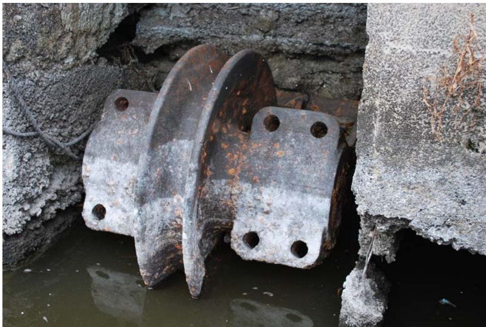
Photograph No. 16 Close up of roller for abandoned low level intake structure at Copco 1 Dam. Copco 1 Dam, Klamath Hydroelectric Project, Oregon-California – April 12-16, 2010.
