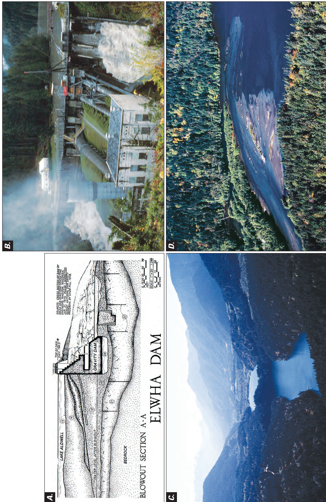
Figure 1.3. Diagram and photographs showing the Elwha Dam, Washington, completed in 1913. (A) Elwha Dam is a concrete gravity dam with adjacent buttress-type intake sections flanked by spillways. (B) The dam measures 32 meters high and is 137 meters wide at its crest. (C) The dam creates the Lake Aldwell reservoir. (D) A large delta of sediment deposits has formed at the head of the reservoir.
