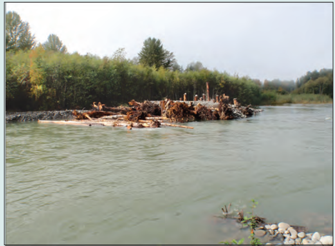
Figure S3.1.1. Newly constructed engineered log jam on the Elwha River, Washington during winter flooding 2009. This structure is one of 50 that the Lower Elwha Klallam Tribe has installed in the lower Elwha River prior to dam removal.
