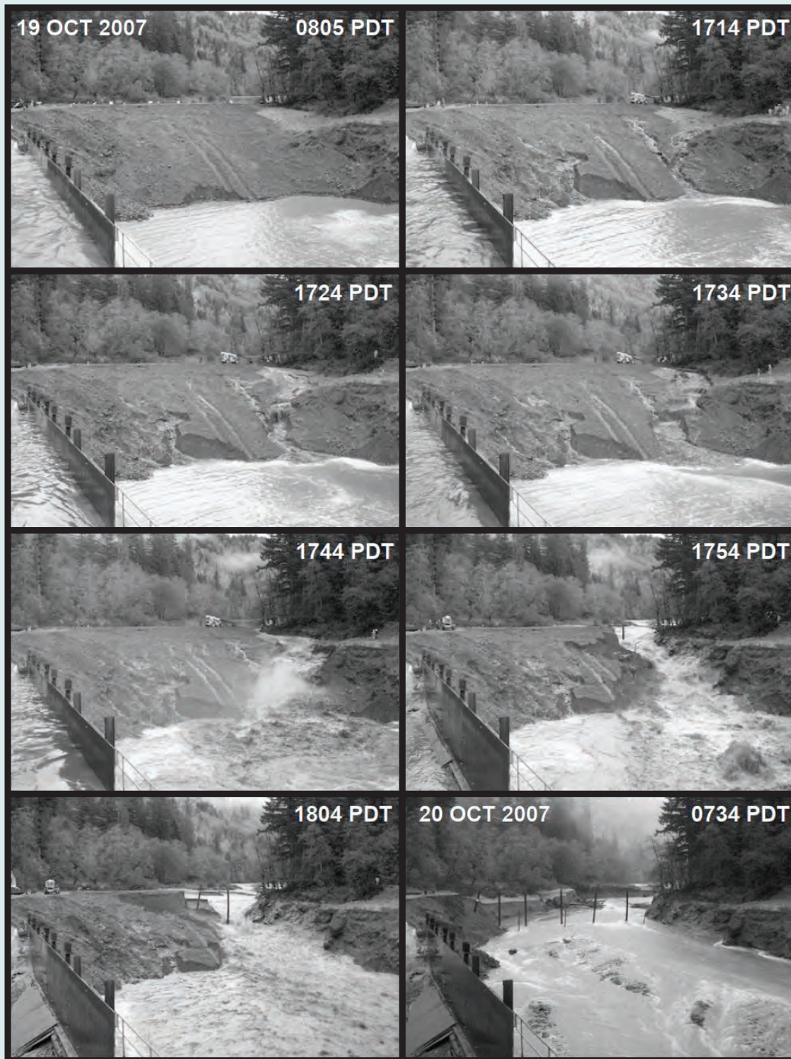
Figure S2.1. Breaching of the temporary earthen coffer dam on October 19–20, 2007, at the site of the manually removed Marmot Dam in northwest Oregon. Note the seepage and mass failures on the downstream face of the dam by 1714 Pacific daylight time (PDT). Incision downward into the coffer dam was nearly complete by 1804 PDT, and nearly all the coffer dam structure had been removed by 0734 PDT the next morning
