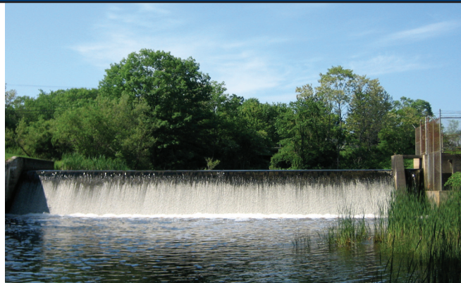
The Winnicut River Dam in spring of 2009, before the project began.
