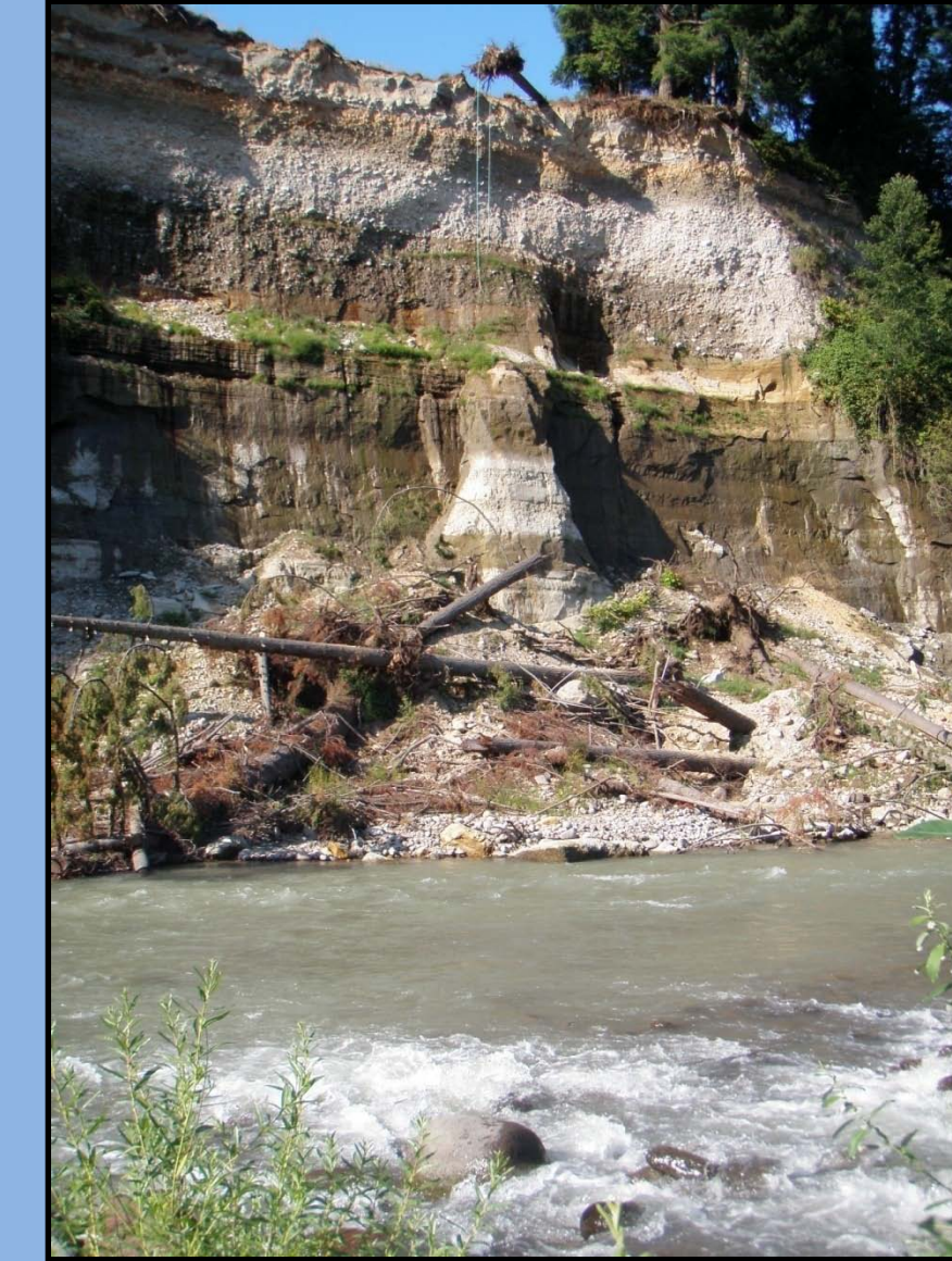
1660 m 3 landslide on cliff face
