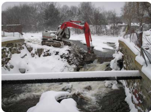
Maxwell Pond Dam Removal, March 2009
