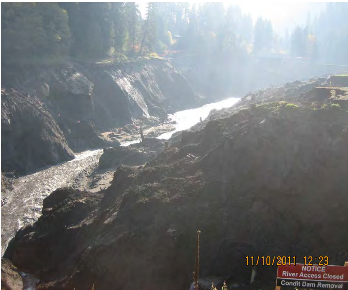
Photo Point #9 Looking Downstream 11.10.11 (Significant reservoir erosion ceased)
