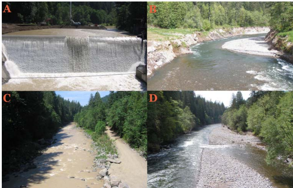
Figure 2 Paired photographs taken from the same location 50m below the dam looking upstream (A&B) and downstream (C&D) before removal (A&C) in July 2007 and after removal (B&D) in July 2009.
