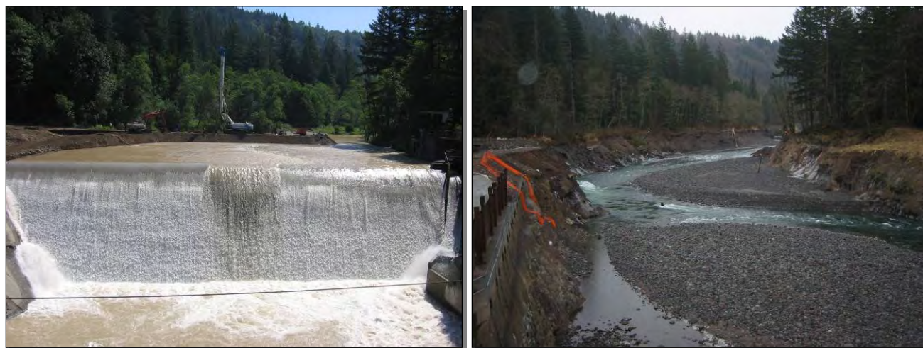
Figure 3 - Marmot Dam Site in July 2007 (left) and January 2008 (right). Construction of the cofferdam is visible in the 2007 photograph.
